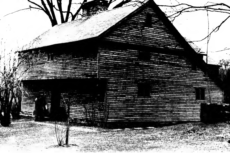
FRAMED OVERHANG, WHITMAN HOUSE, FARMINGTON
