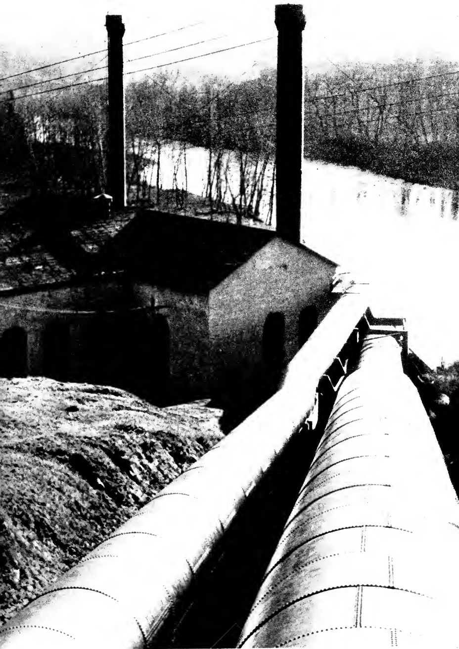
HYDROELECTRIC PLANT, BULLS BRIDGE
