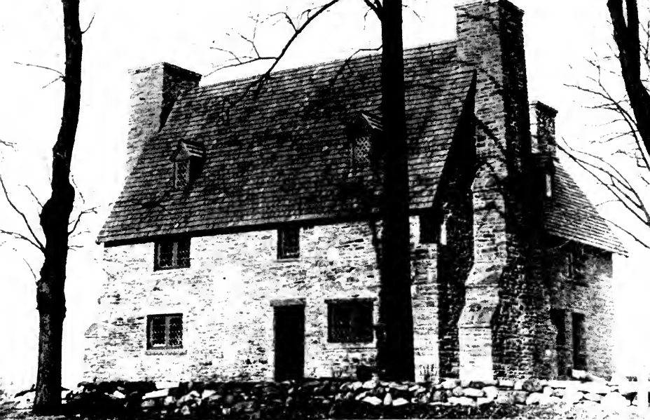
WHITFIELD STONE HOUSE, GUILFORD
