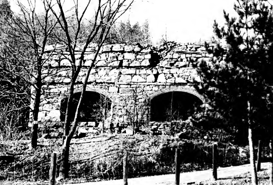
CEMENT KILN, WOODBRIDGE
