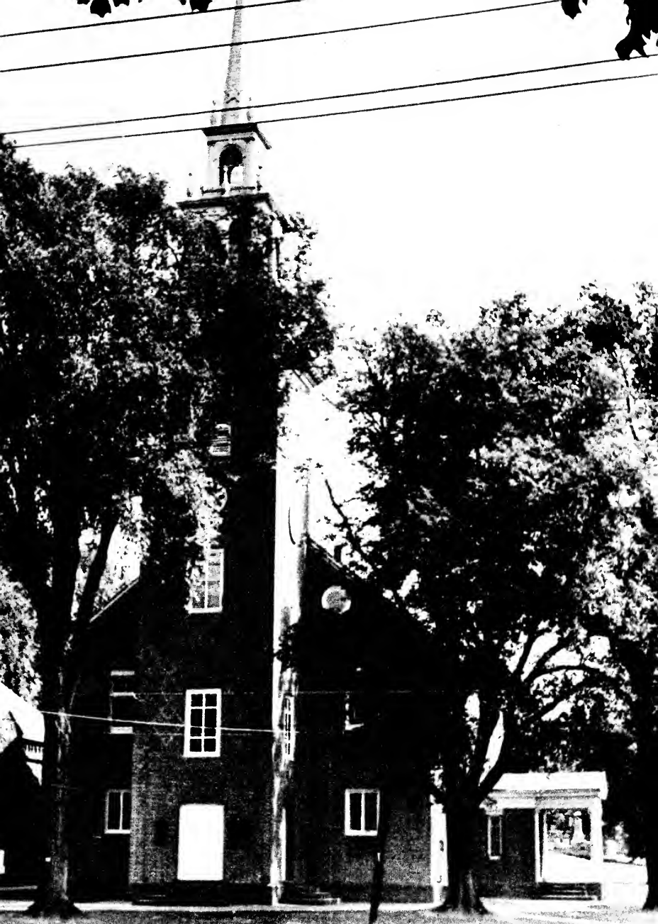
CONGREGATIONAL CHURCH, WETHERSFIELD
