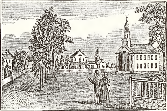
South view of the central part of Canterbury.
