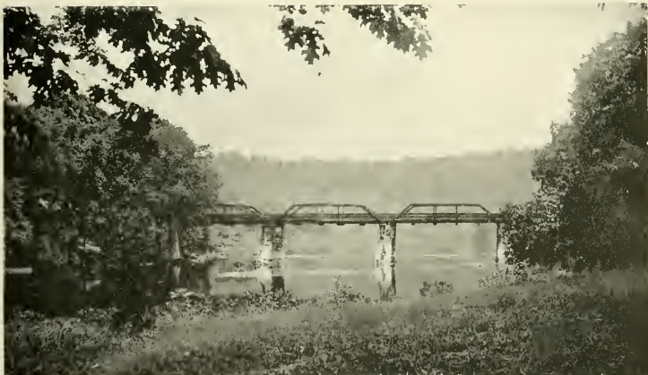
BRIDGE AT TARIFFVILLE.
