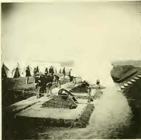
MORTAR BATTERY, LOOKING SOUTH.
