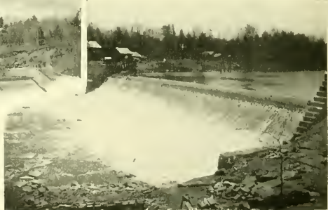
AT THE FARMINGTON RIVER POWER CO'S STATION.
