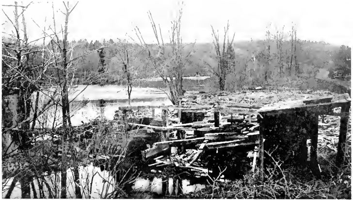
RUINS OF THE SPOONVILLE FACTORY, Where electro-plated ware was first made in the United States.
