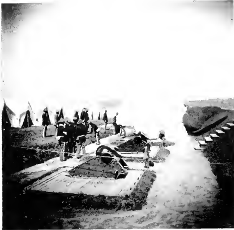
MORTAR BATTERY, LOOKING SOUTH.
