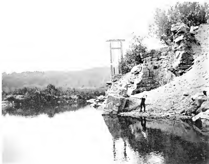
THE BROKEN DAM.
