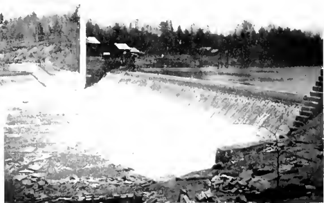
AT THE FARMINGTON RIVER POWER CO'S STATION.
