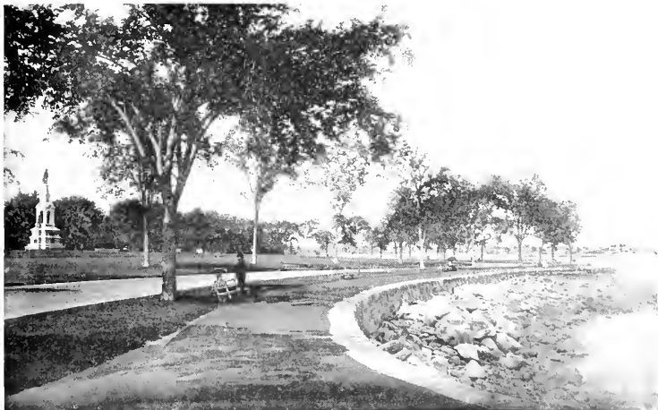
VIEW SHOWING SEA-WALL.
