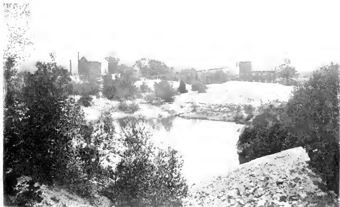
PLANT AT BRISTOL MINES, (GENERAL VIEW).
