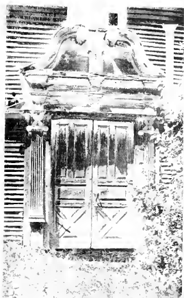
DOORWAY TO CHERHILL HOUSE, BUILT ABOUT 1750.
