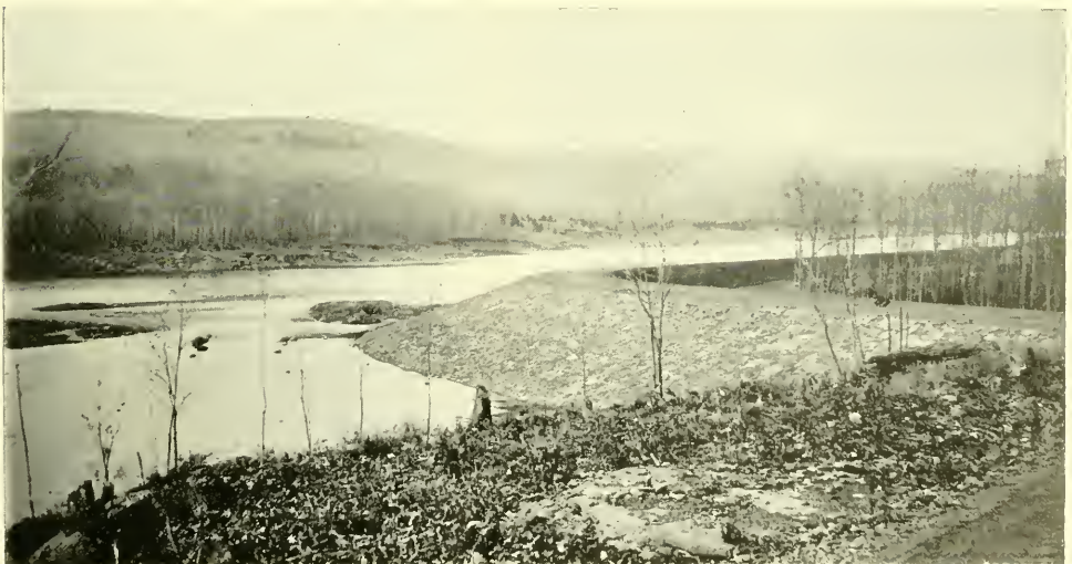
DAM AND DRIVE EAST OF RESERVOIR NO. 6.
