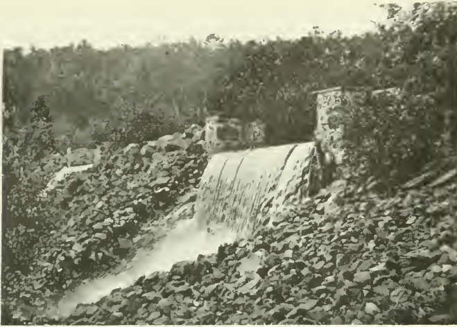
OVERFLOW FOR RESERVOIR NO. 5.
