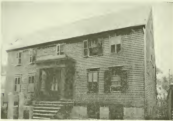
THE TROWBRIDGE HOUSE.
