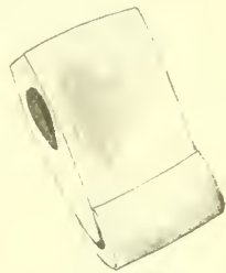
THE OVERCOAT STEEL IN PLACE.
