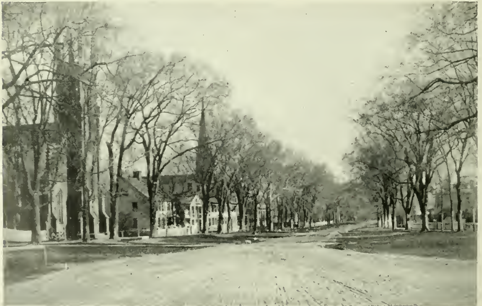
SOUTH STREET LOOKING SOUTH.
