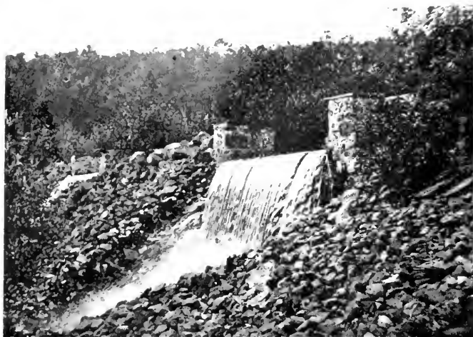
OVERFLOW FOR RESERVOIR NO. 5.
