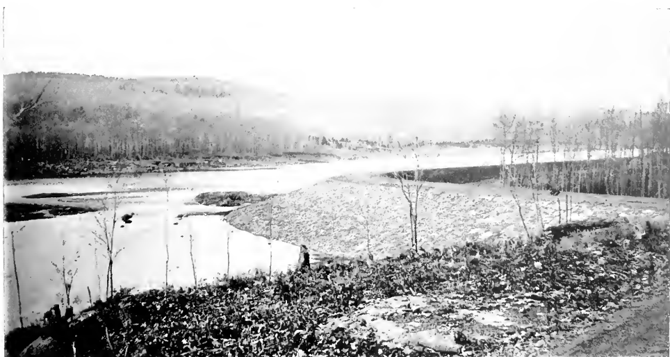
DAM AND DRIVE EAST OF RESERVOIR NO. 6.
