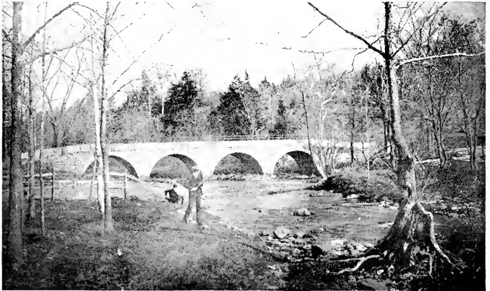
THE BRIDGE AT BROOKSIDE, SOUTH GLASTONBURY.
