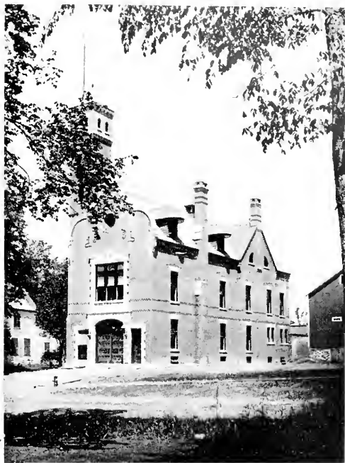
FIRE DEPARTMENT BUILDING.
