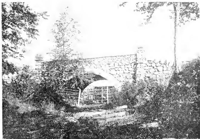
CLARK BRIDGE, OVER "PARADISE BROOK."
