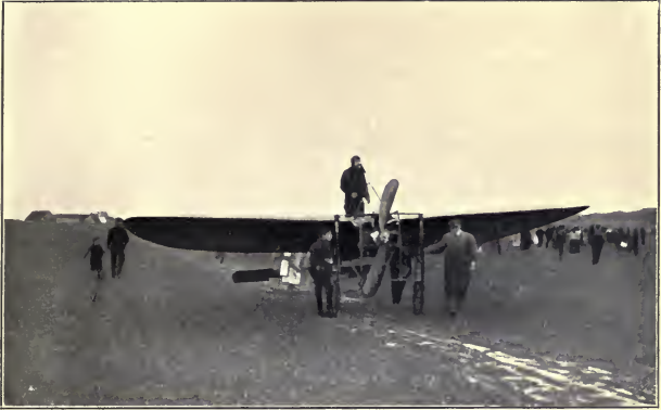
THE BLÉRIOT AEROPLANE PREPARING TO LEAVE THE FRENCH COAST (THE AVIATOR STANDING ON HIS BIRD, AND THE WOODEN PROPELLER AND MOTOR CAN BE PLAINLY SEEN)
