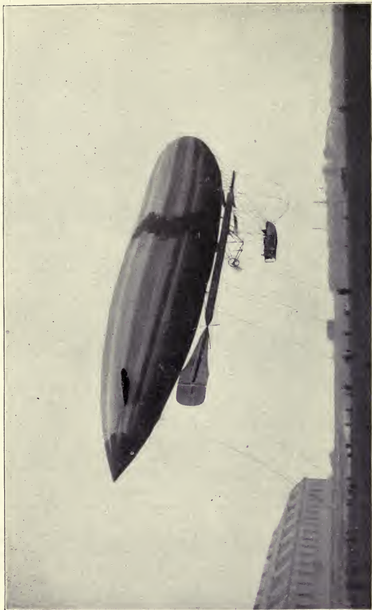
THE "PARSEVAL" FLEXIBLE AIRSHIP WITH TWO COMPENSATING BALLONETS
