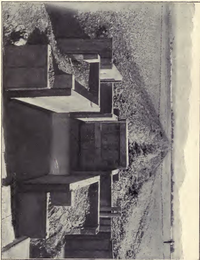
DIVISION BOX AT BOZEMAN, MONTANA, SHOWING METHOD OF TURNING WATER INTO LATERALS FOR IRRIGATING THE FIELD
