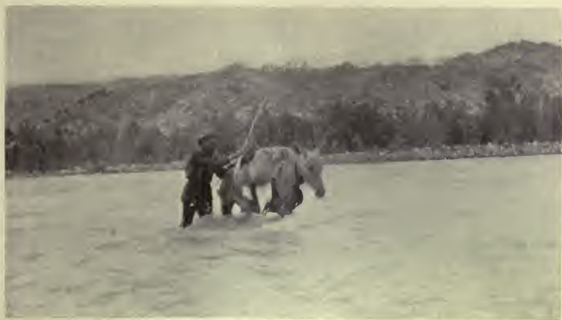
ED. BARRILL FORDING THE EAST BRANCH OF THE KAHILTNA RIVER.
