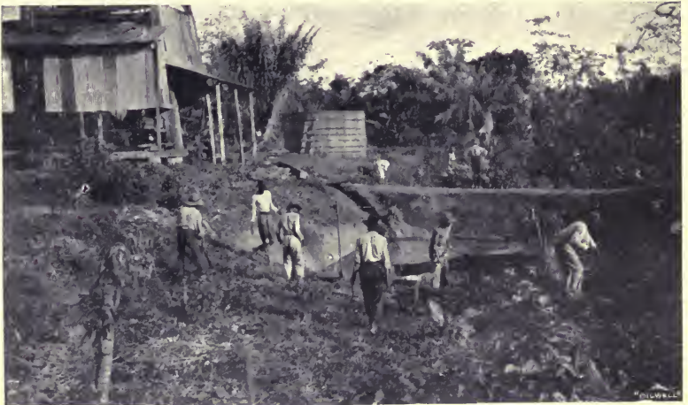
DIGGING A "SUMP" ON A TRINIDAD OIL-FIELD. A pond is provided near the well to receive the oil directly it is struck.
