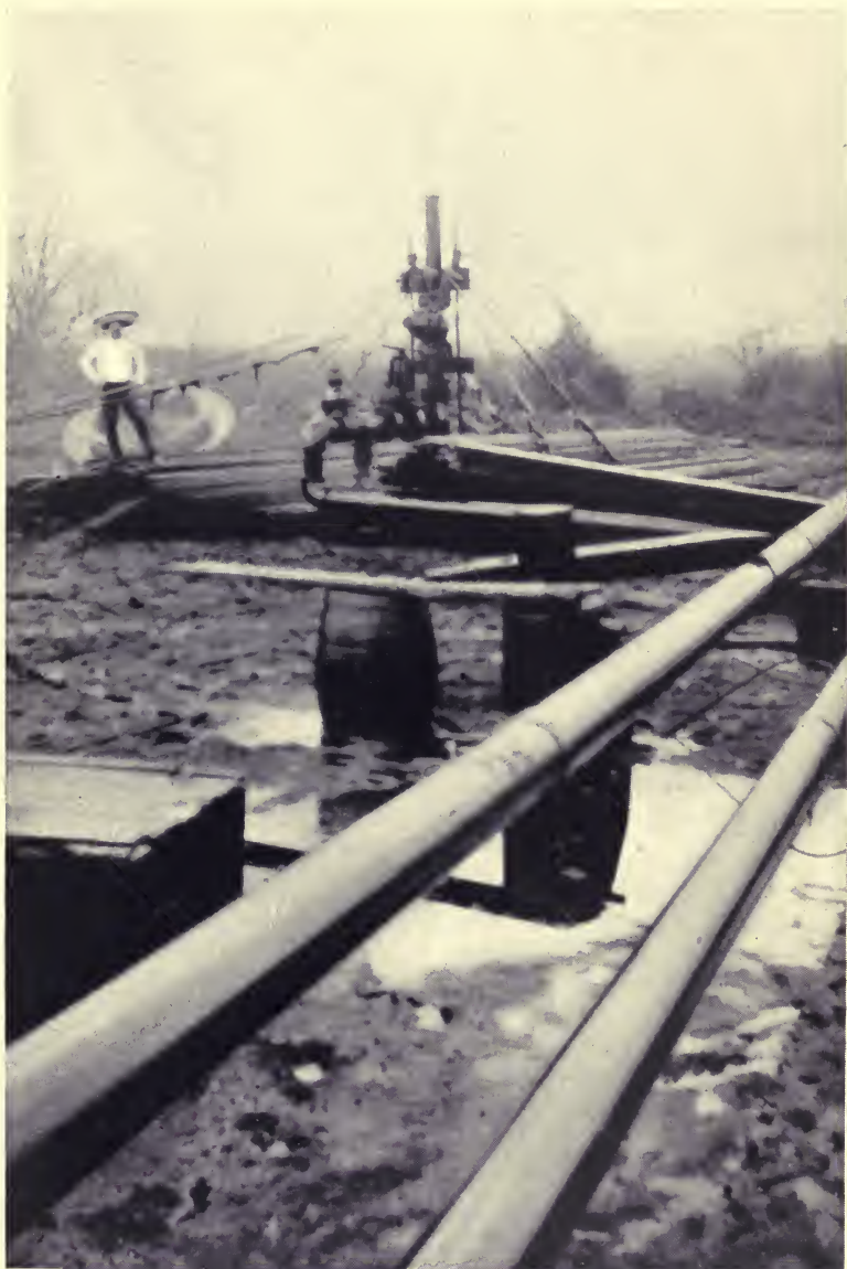
THE GATE VALVE WHEREWITH THE MEXICAN GUSHER POTRERO DE LLANO NO. 4 WAS BROUGHT UNDER CONTROL.
