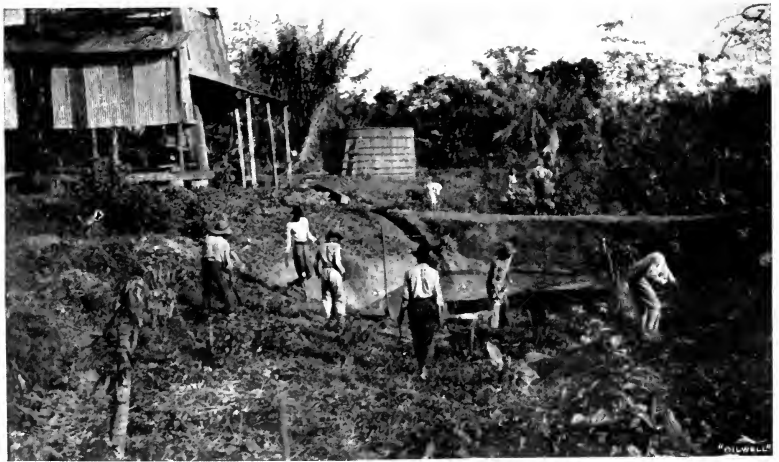
DIGGING A "SUMP" ON A TRINIDAD OIL-FIELD. A pond is provided near the well to receive the oil directly it is struck.
