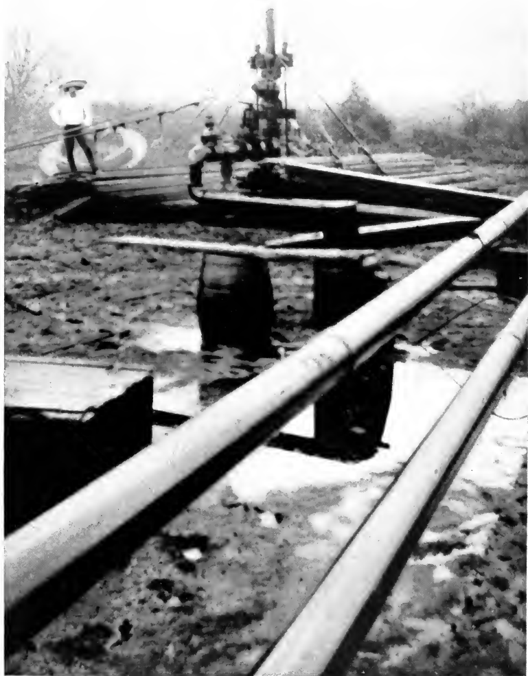
THE GATE VALVE WHEREWITH THE MEXICAN GUSHER POTRERO DE LLANO NO. 4 WAS BROUGHT UNDER CONTROL.
