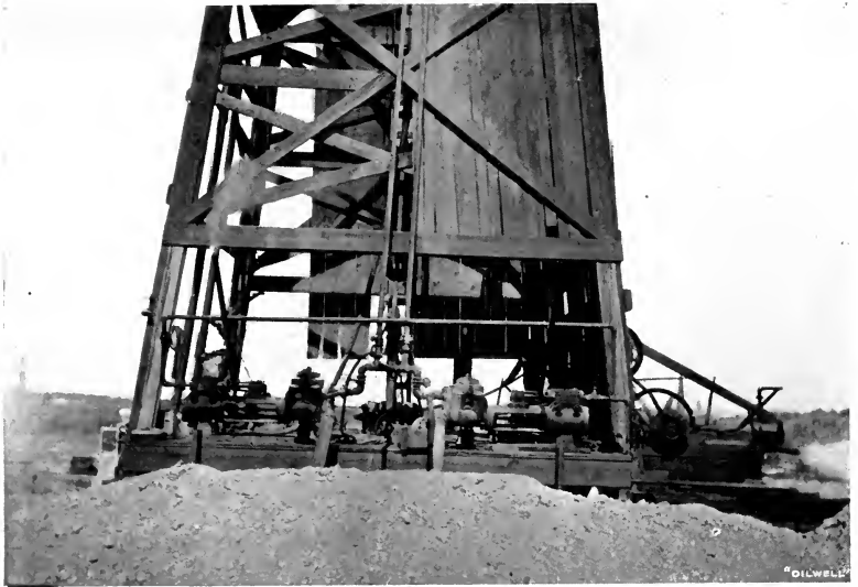
GENERAL VIEW OF A ROTARY DRILLING PLANT.
