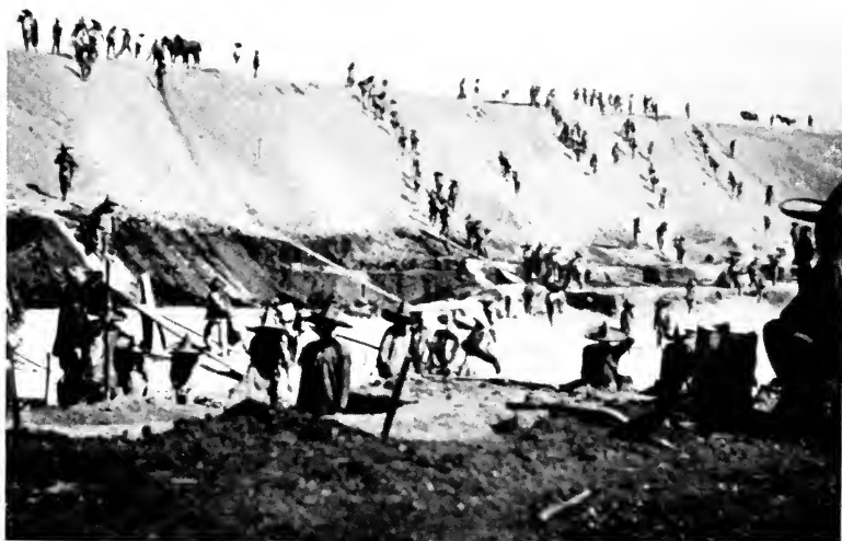
BUILDING THE EARTH RESERVOIR TO RECEIVE THE FLOW FROM POTRERO DE LLANO NO. 4.
