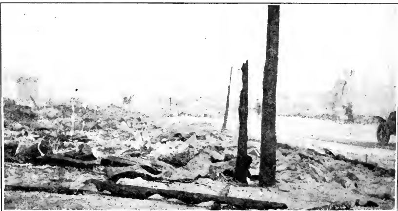
ANOTHER VIEW IN CHISHOLM, AFTER THE FIRE
