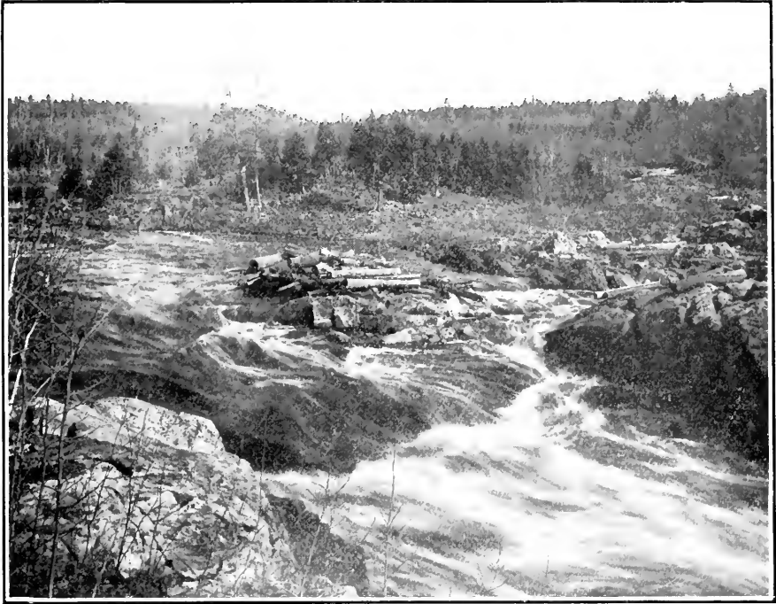
Dam Site on Chippewa River, Wisconsin, at Brunett's Falls
