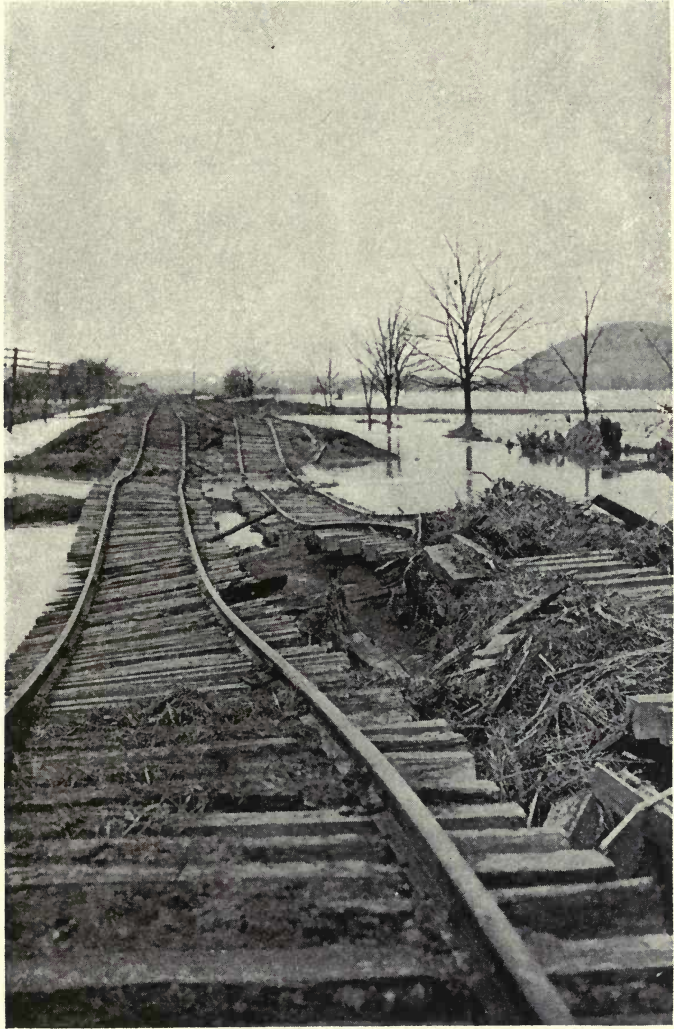
FIG. 85. TRACK OF MAIN NEW YORK-ST. LOUIS LINE NEAR NEWCOMERSTOWN, OHIO
