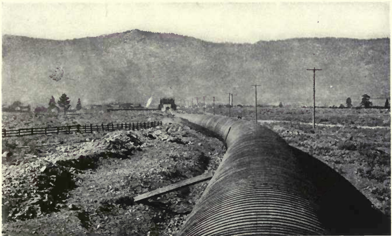
FIG. 42. TRUCKEE RIVER GENERAL ELECTRIC CO. WOOD STAVE PIPE (Stone and Webster Eng. Corp.)
