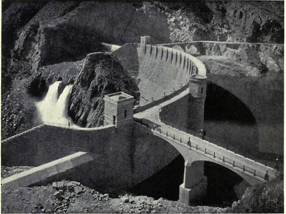
FIG. 26. ROOSEVELT DAM, SALT RIVER PROJECT, ARIZONA
