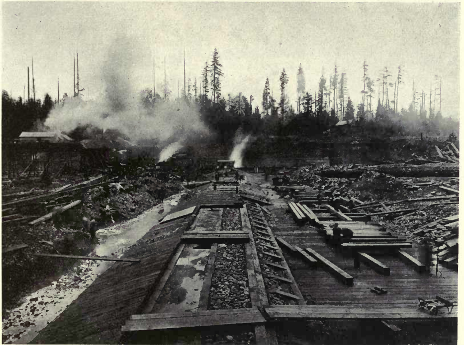
FIG. 25. A LOW AND INEXPENSIVE DAM ACROSS WHITE RIVER, WASHINGTON (Stone and Webster Eng. Corp.)
