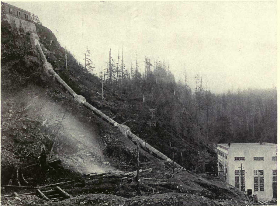
FIG. 57. POWER HOUSE AND PENSTOCK—SNOQUALMIE FALLS DEVELOPMENT PUGET SOUND TRACTION, LIGHT AND POWER CO., SEATTLE, WASH. (Stone and Webster Eng. Corp.)
