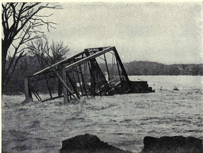
FIG. 82. BRIDGE No. 83, OVER KOKOSING RIVER
