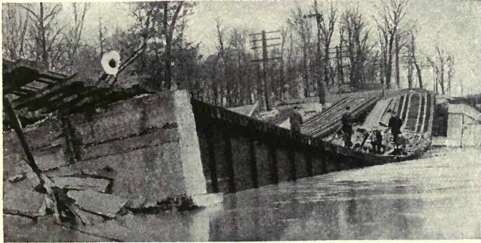
FIG. 81. BRIDGE OVER BLACK FORK, WHICH HAD TO BE ENTIRELY REPLACED
