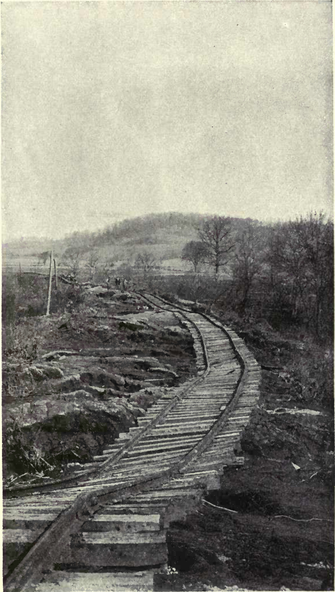
FIG. 86. NORTH OF BRIDGE NO. 123. NORTH OF WARSAW, OHIO Track was, before the flood, on a high embankment
