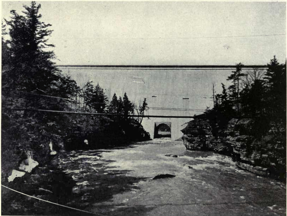
FIG. 28. ASHOKAN DAM, N. Y. WATER SUPPLY, SHOWING STREAM FLOWING THROUGH CONDUIT LATER FILLED WITH CONCRETE
