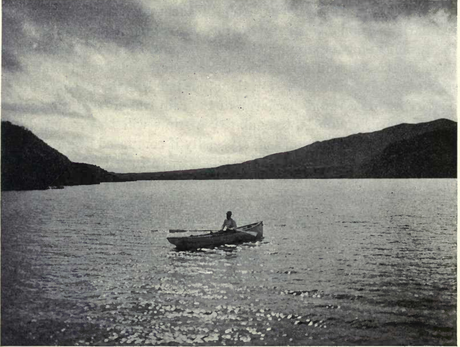
FIG. 4. SALT RIVER PROJECT, ARIZONA
