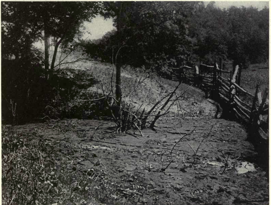
FIG. 68. EROSION OF TOP LAYER OF SOIL, BALSAM GAP, JACKSON CO., N. C. (U. S. Forest Service)
