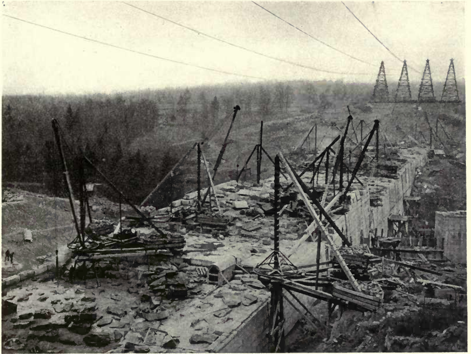
FIG. 29. ASHOKAN DAM UNDER CONSTRUCTION (J. Waldo Smith, Chief Engineer)
