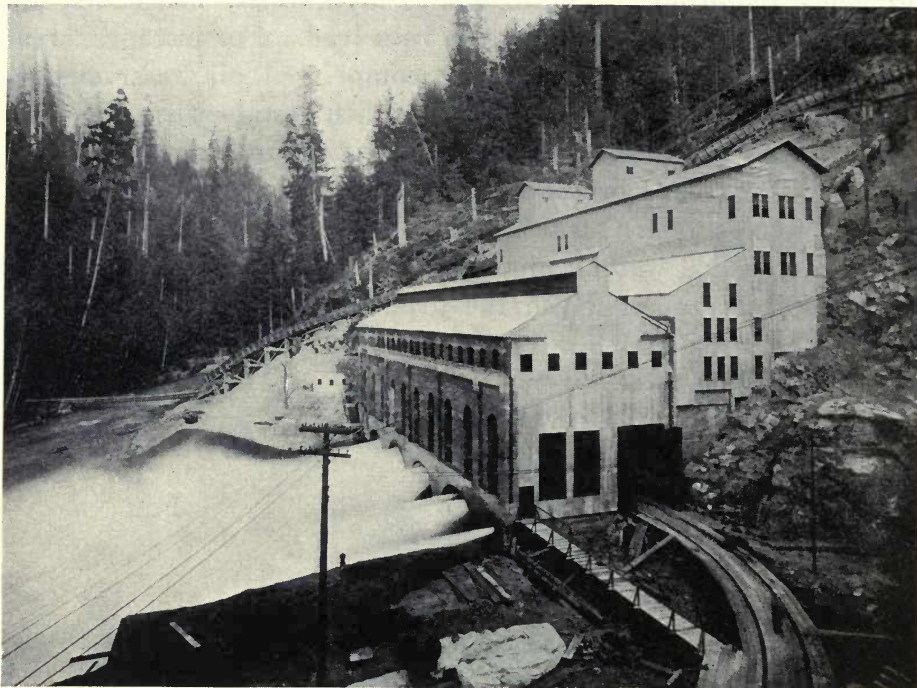
FIG. 59. POWER HOUSE WITH FOUR UNITS IN OPERATION—ELECTRON DEVELOPMENT PUGET SOUND TRACTION, LIGHT AND POWER CO., SEATTLE, WASH.
