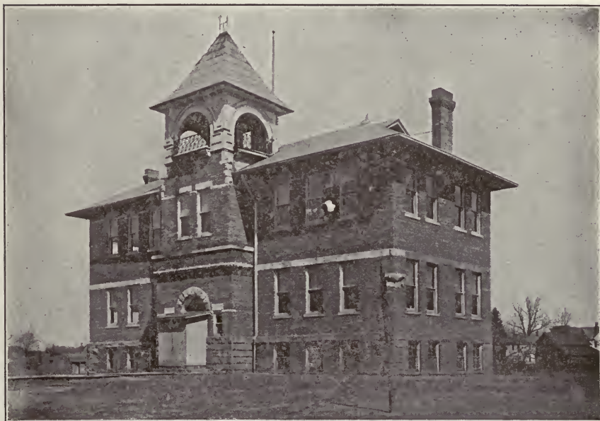
Kinsman Township Consolidated School Building, Trumbull County, Ohio.
