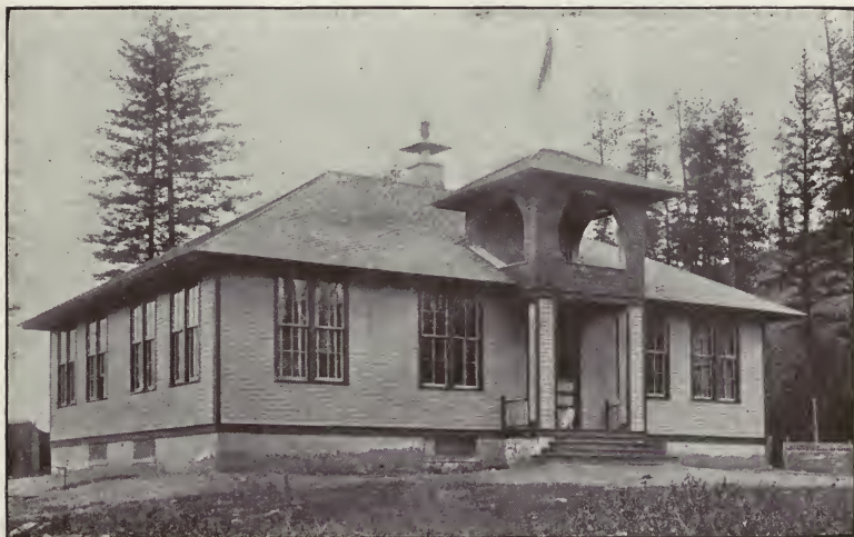
Milan Consolidated School Building in Spokane County.
