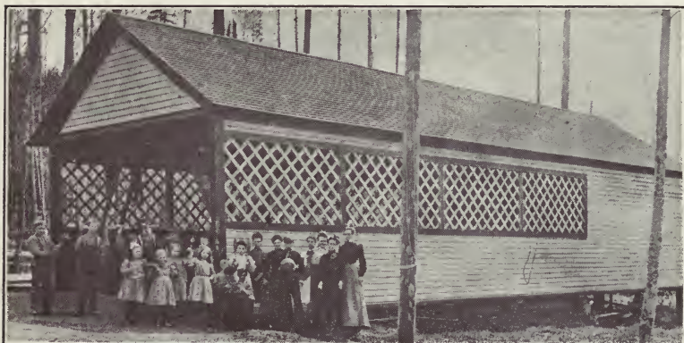
Rural School Gymnasium in Skagit County.
