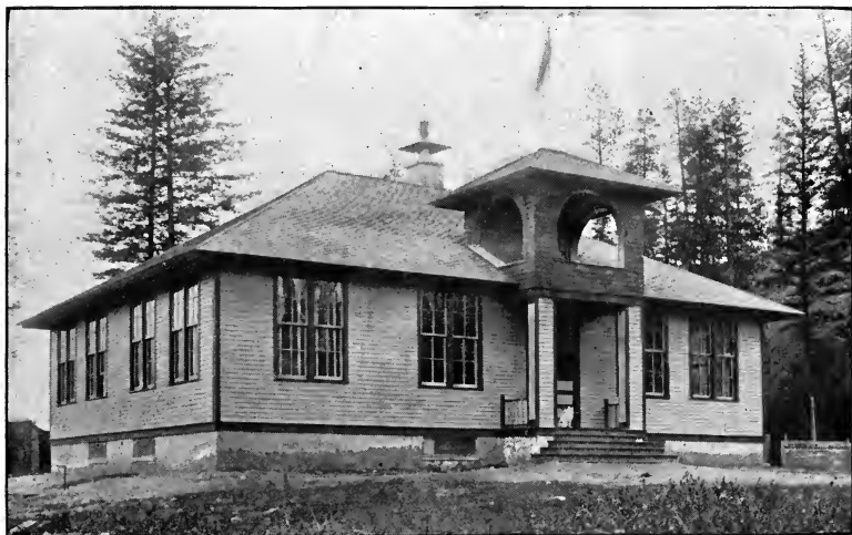
Milan Consolidated School Building in Spokane County.
