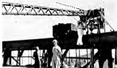
Grinding the track on which huge dome will rotate. Note small wheel inside yoke grinding side of track.
