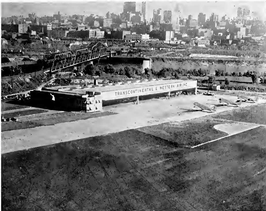
TWA's system maintenance base at Kansas City, considered by many as the most modern base of its kind in the world.
