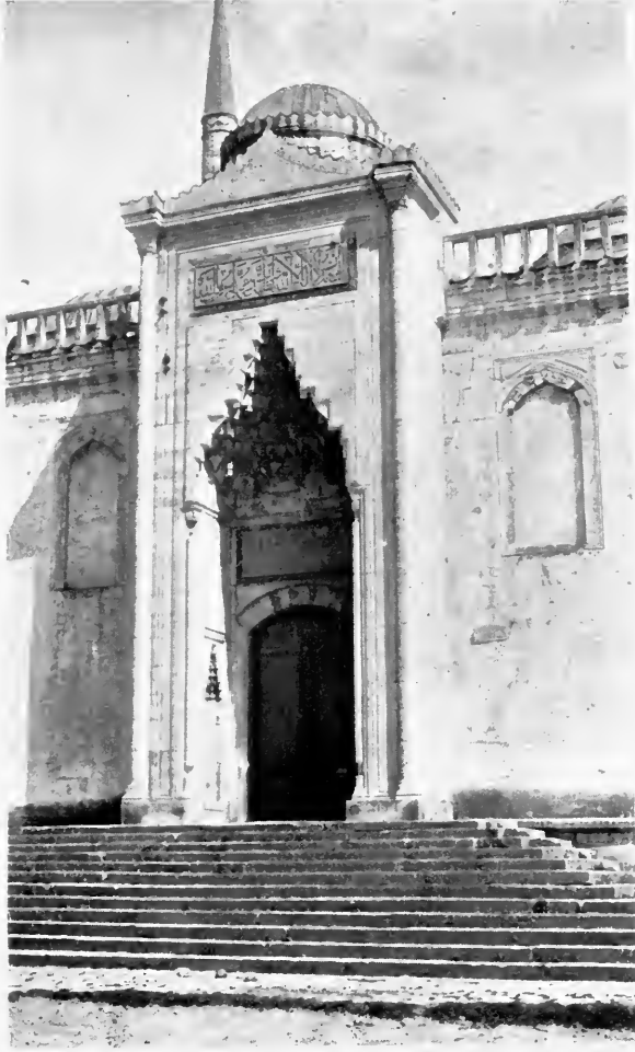
PRINCIPAL ENTRANCE OF THE MOSQUE OF SULTAN ACHMET I
