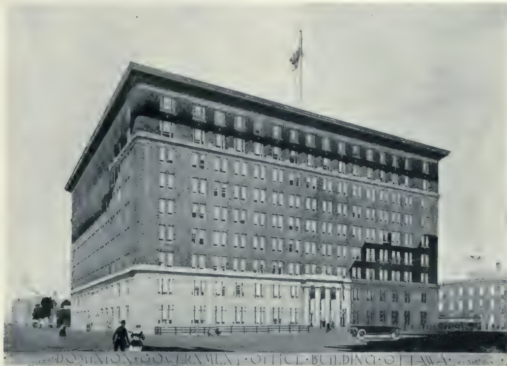
DOMINION GOVERNMENT OFFICE BUILDING, OTTAWA, FOR WHICH THE CONTRACT WAS RECENTLY LET.
