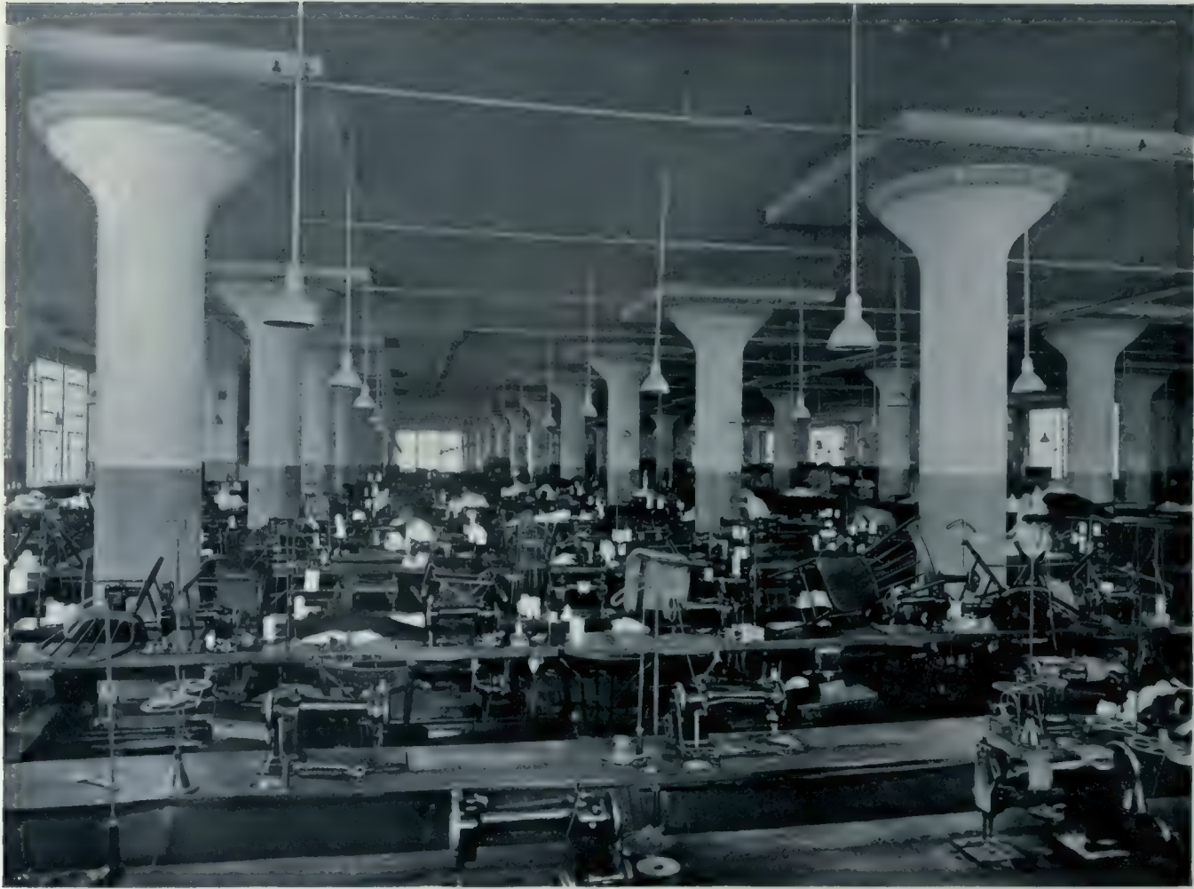
VIEW SHOWING TYPICAL FINISHED COLUMNS, THE T. EATON COMPANY'S NEW FACTORY, TORONTO.
