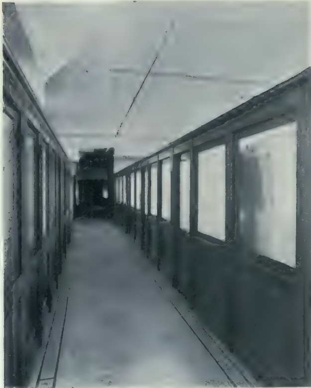
UPPER FLOOR OFFICE CORRIDOR.
