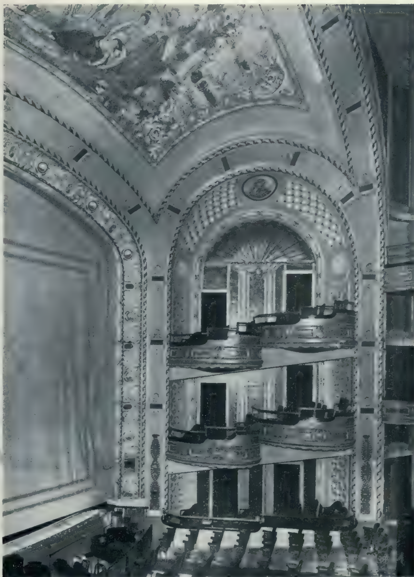
DETAIL OF BOXES, NEW PRINCESS THEATRE, MONTREAL.
