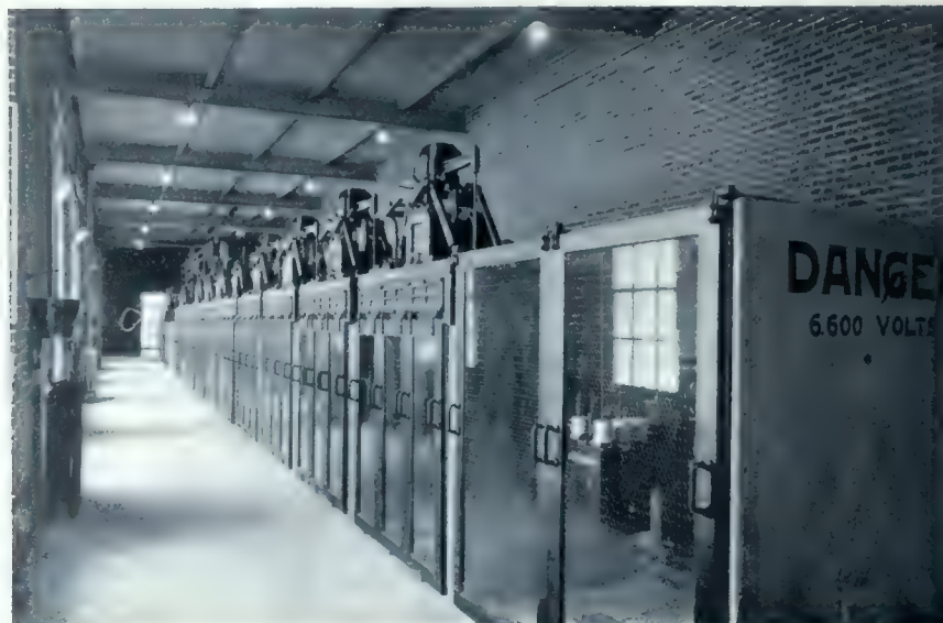
ENCLOSED SWITCHES.
