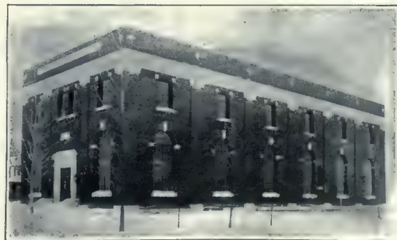
Pointe Aux Trembles Power-House of Montreal Tramways Co. General Contractors: Muir & Shea, Montreal. Roofers: Metal Shingle & Siding Co., Limited, Montreal.
