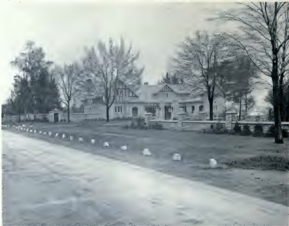
STABLE AND GARAGE, MAJOR W. F. EATON'S ESTATE, OAKVILLE, ONT.
