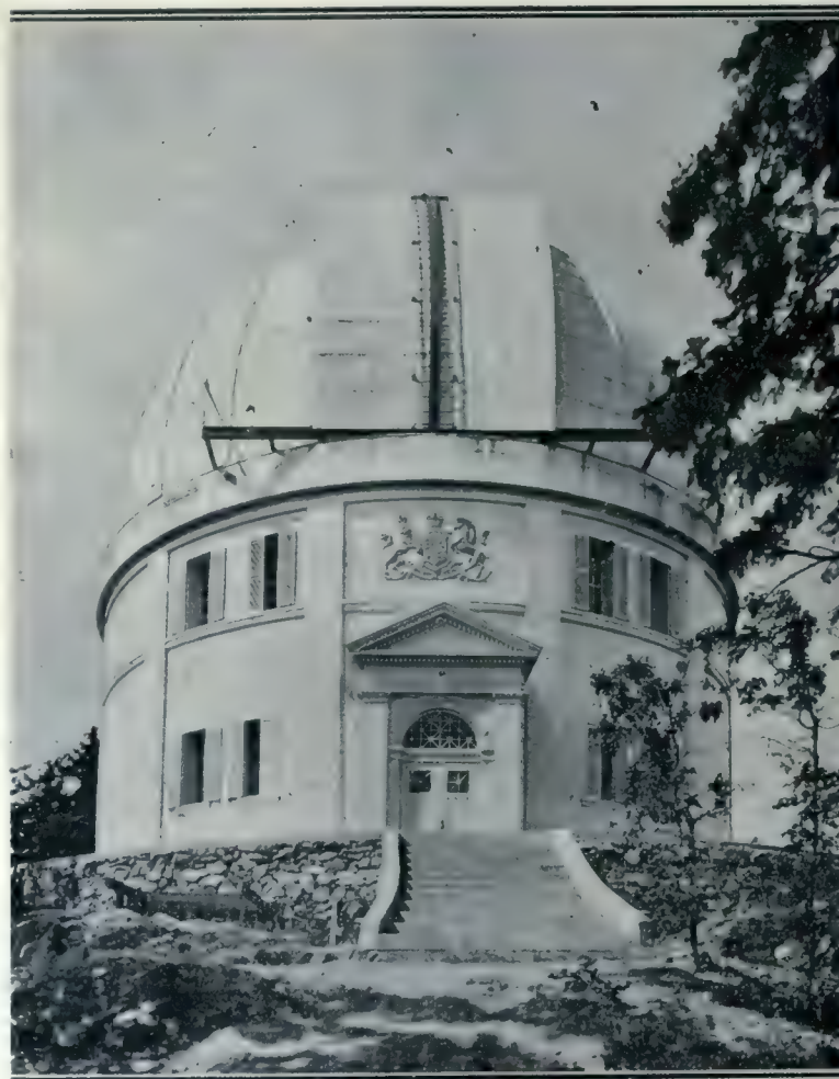
THE BRITISH COLUMBIA OBSERVATORY IS CIRCULAR, 66 FEET IN DIAMETER AND SURMOUNTED BY A REVOLVING DOME. IT IS ENTIRELY OF STEEL CONSTRUCTION.
