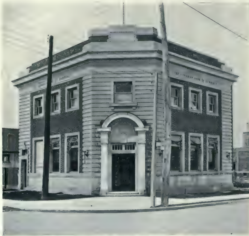
EARLSCOURT BRANCH, CANADIAN BANK OF COMMERCE, TORONTO. V. D. HORSBURGH, F.R.I.B.A., ARCHITECT.
