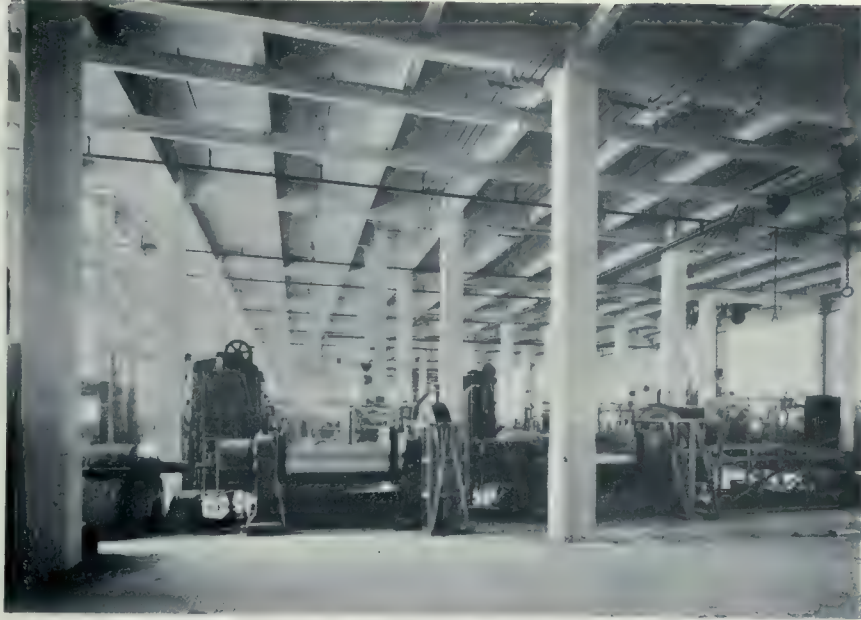
MILL ROOM, GOODYEAR TIRE AND RUBBER COMPANY'S NEW FACTORY.
