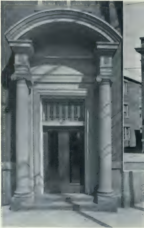
DETAIL OF ENTRANCE.
