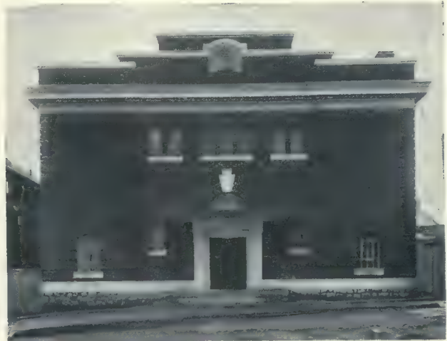
ARCHIVES BUILDING, VANCOUVER, B.C.
