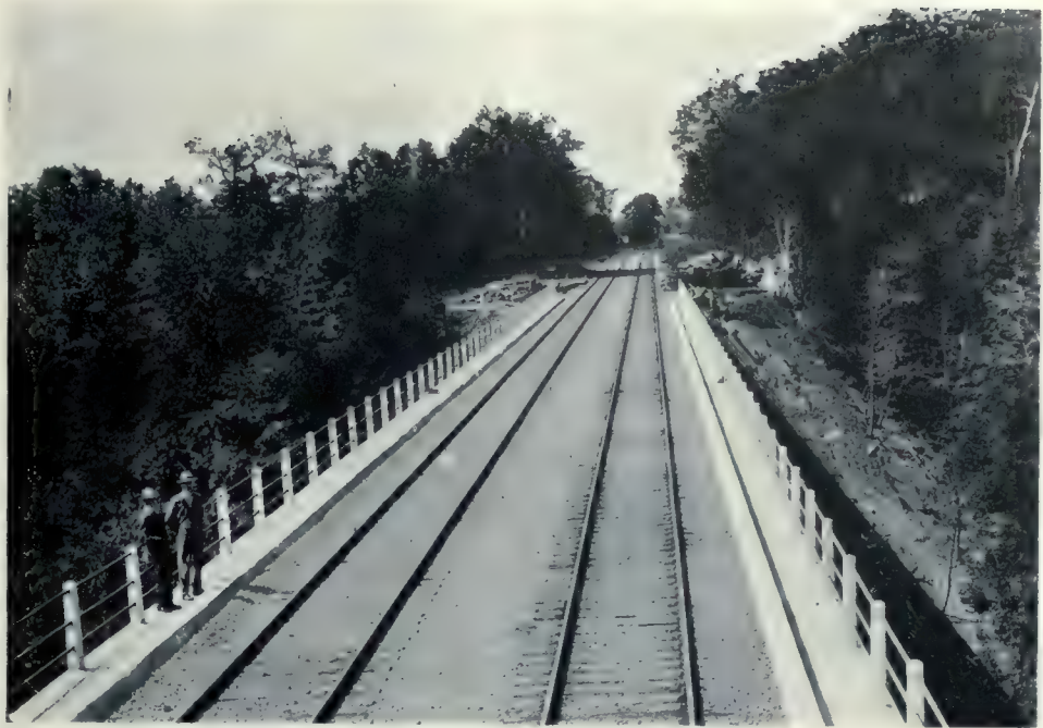
VIEW ALONG VIADUCT AT ROADBED LEVEL.
