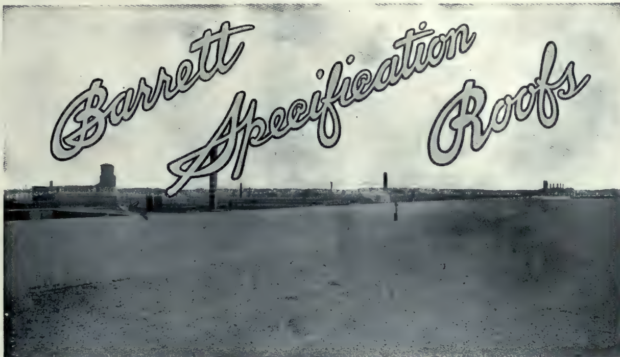
Barrett Specification Roof on CANADIAN FAIRBANKS-MORSE Co., Limited, Toronto, Ont. Engineers: T. Pringle & Son, Limited, Montreal and Toronto Roofer: R. Gilday, Toronto
