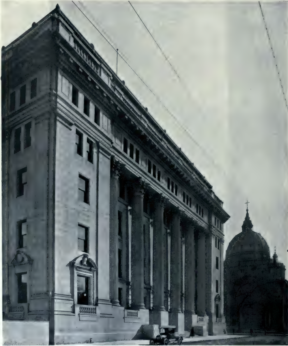
Sun Life Building, Montreal.
