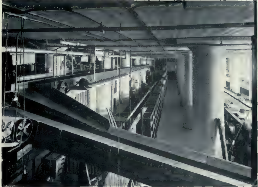
MEZZANINE VIEW SHOWING CONVEYOR AND PARCEL CHUTE.
