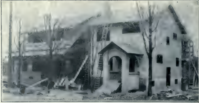
Houses erected by E. A. Grison, Esq., Ottawa, Ont. Outside walls of 2 x 4 studding. Stucco Board on exterior. Sheathing Board on interior. Over Sheathing Board, a 1 x 2 Furring was applied, then Stucco Board and Plaster, giving double air space, increasing the warmth, yet keeping down the cost.
