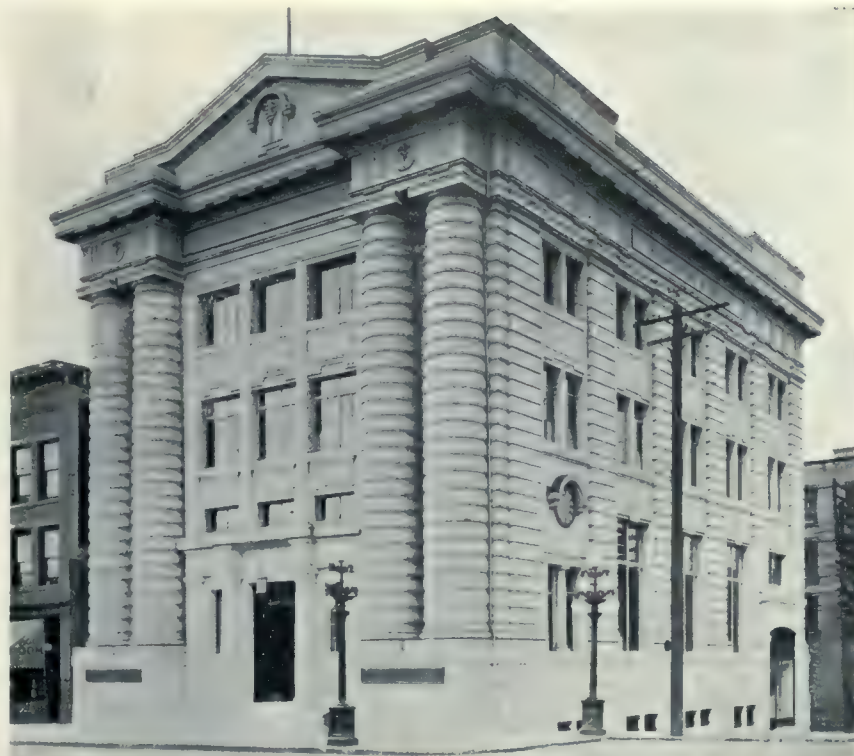
CANADIAN BANK OF COMMERCE (EAST END BRANCH), VANCOUVER, B.C. V. D. HORSBURGH, F.R.I.B.A., ARCHITECT.
