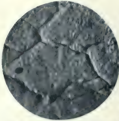
Figure 1.—White lead paint showing chalked condition.
