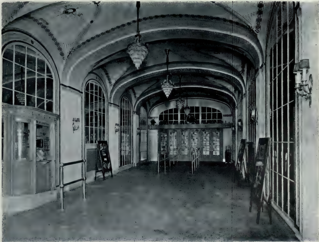
ENTRANCE LOBBY, LOEW'S THEATRE, HAMILTON, ONT.
