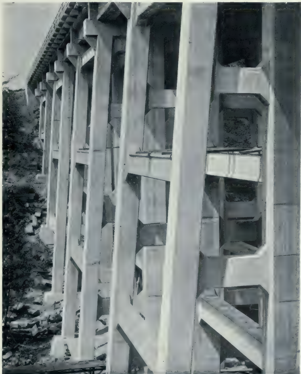
CLOSE VIEW OF C.P.R. VIADUCT NO. 0.9, NORTH TORONTO SUBDIVISION.
