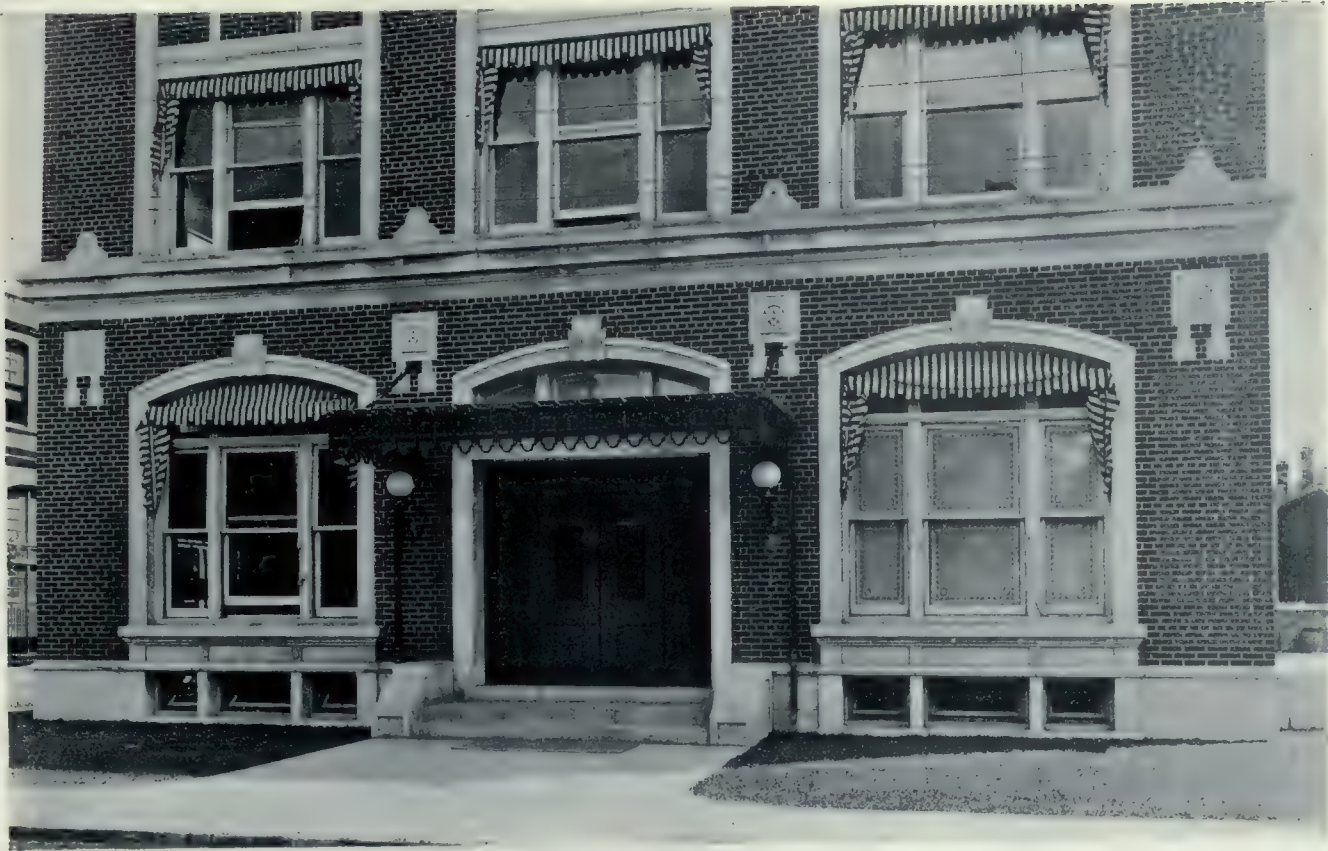
LOWER FACADE. GENERAL OFFICES, CANADIAN WESTINGHOUSE COMPANY, HAMILTON, ONT.
