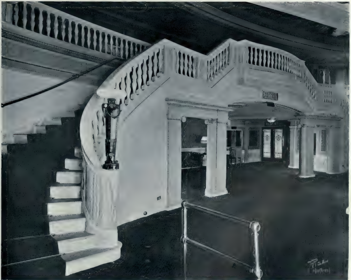
GRAND STAIRCASE, LOEW'S THEATRE, MONTREAL.
