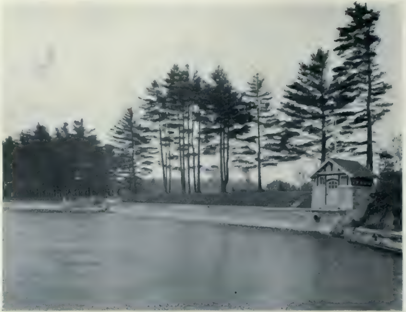
CONCRETE SEA-WALL, MAJOR W. F. EATON'S ESTATE, OAKVILLE, ONT.
