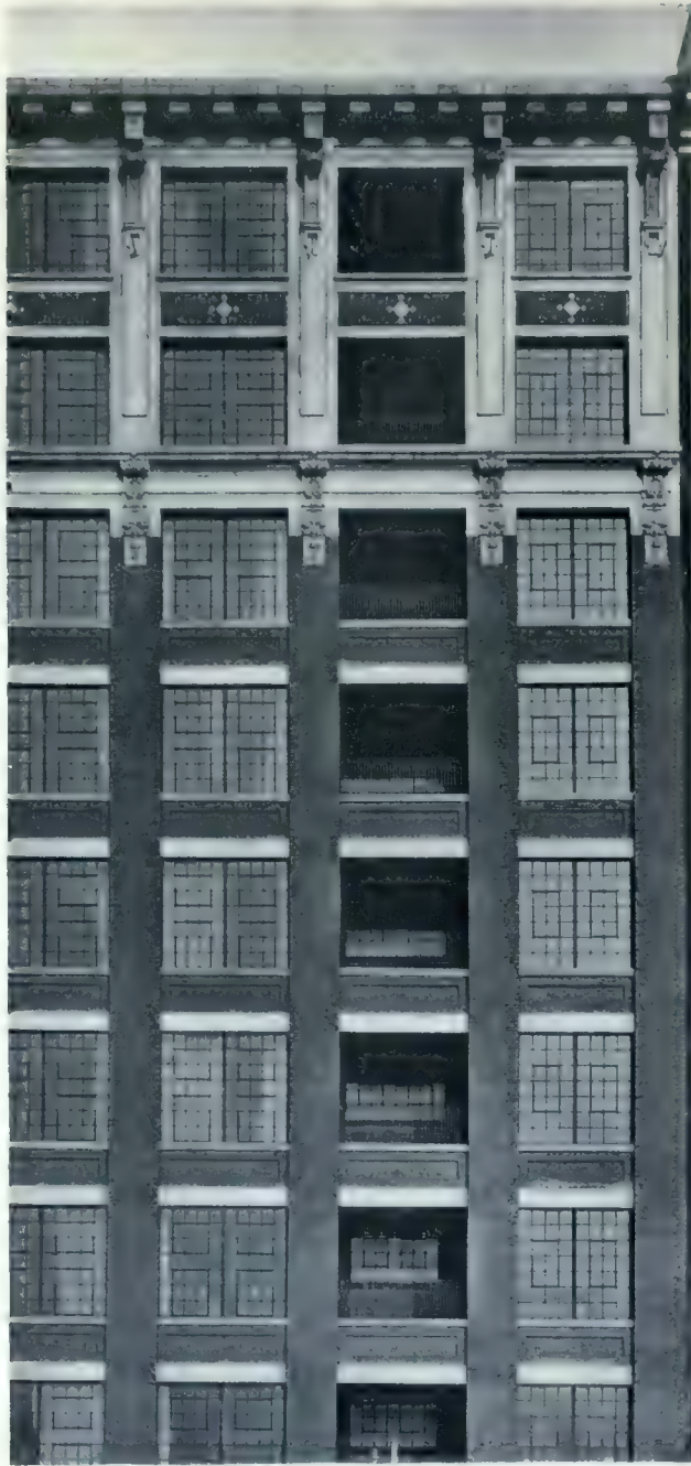
OPENING OR AIR SPACE ADJOINING ENCLOSED STAIRCASE.
