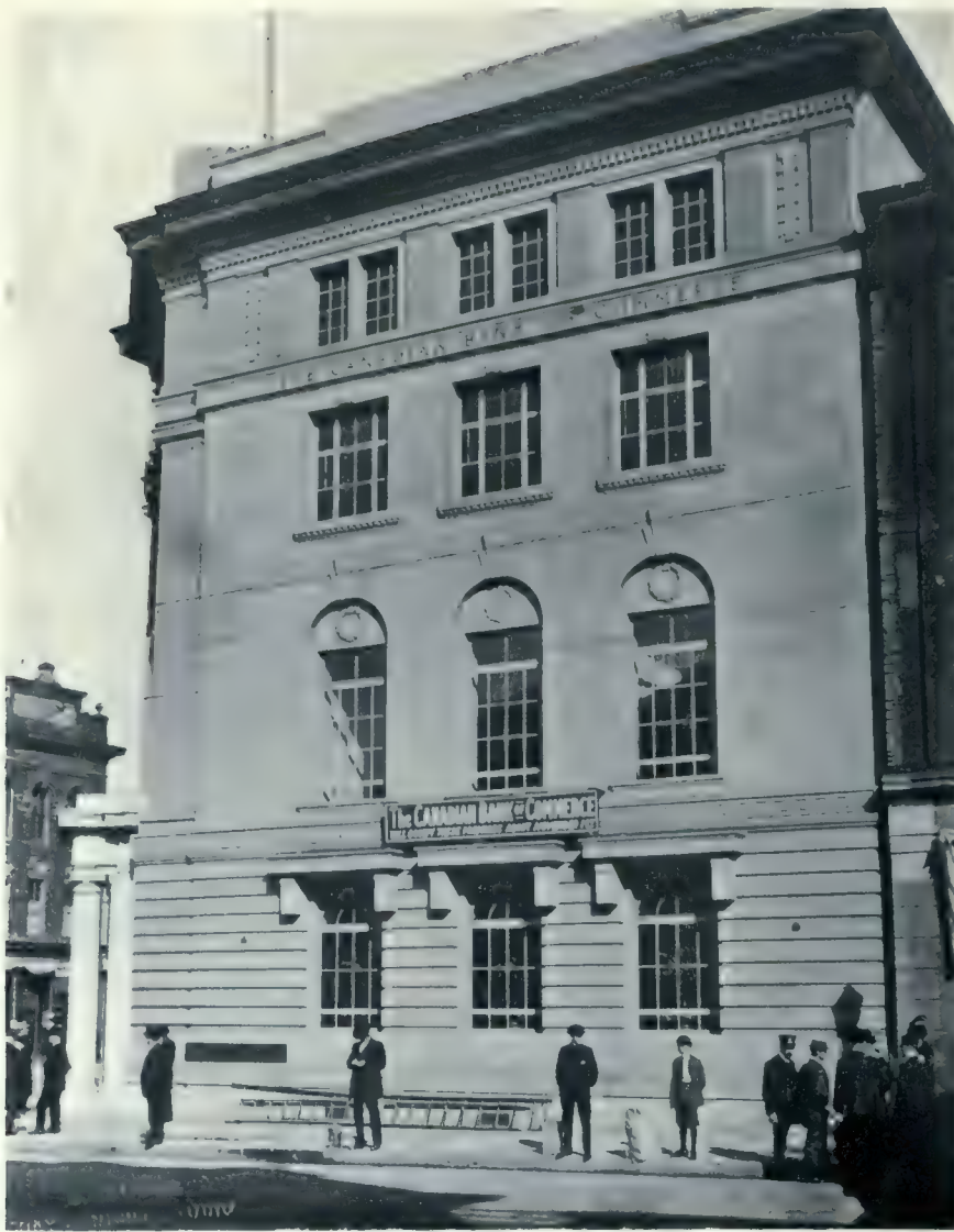
CANADIAN BANK OF COMMERCE, WINDSOR, ONT. V. D. HORSBURGH, F.R.I.B.A., ARCHITECT.
