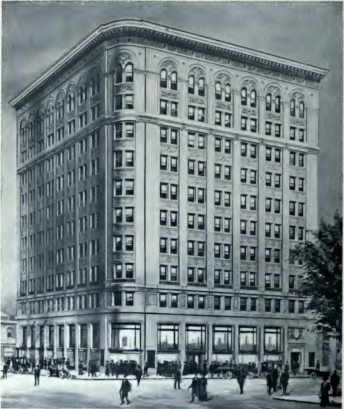
BIRKS BUILDING, VANCOUVER, B.C.
