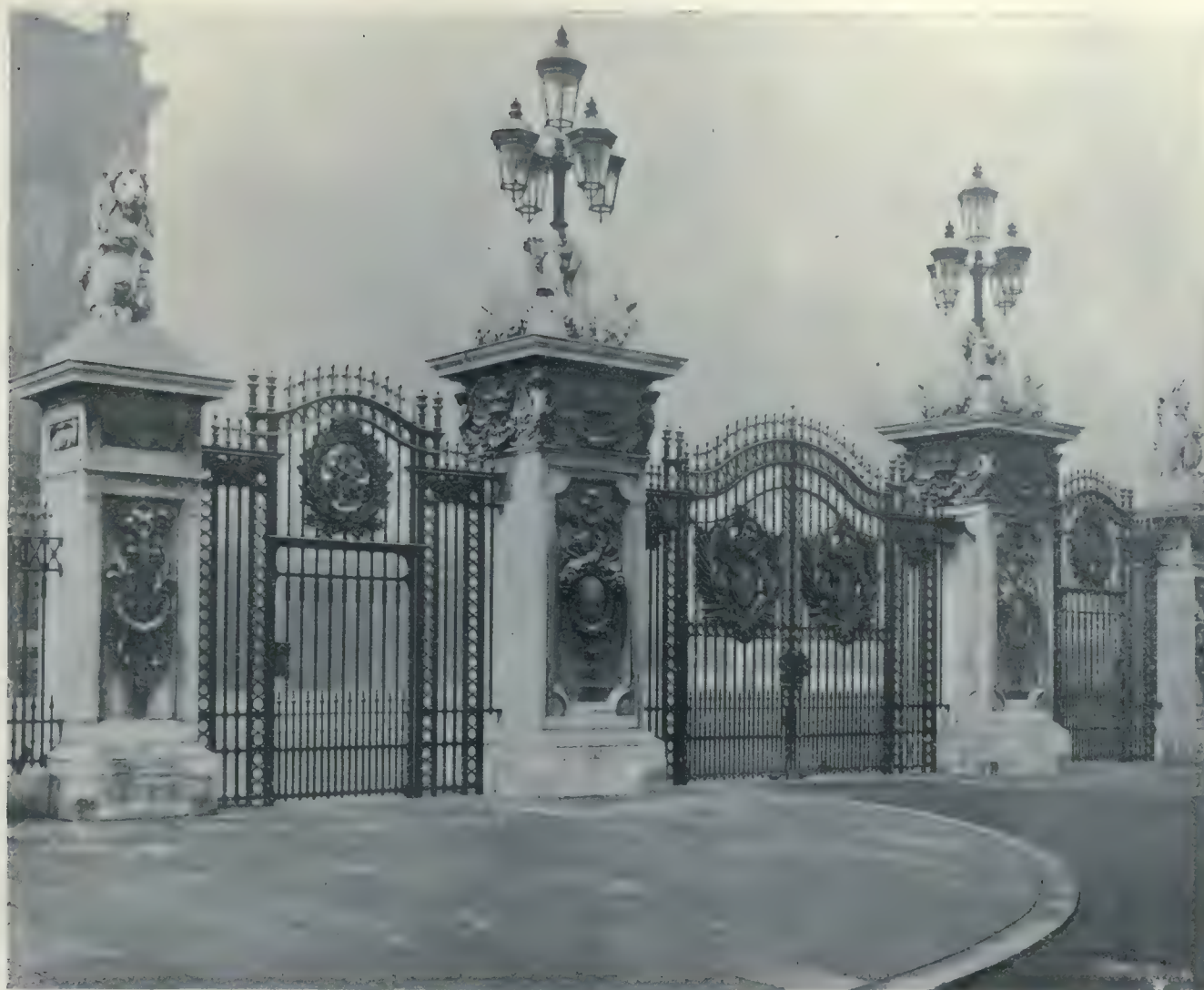
GATES OF BUCKINGHAM PALACE, AN IMPRESSIVE AND STATELY EXAMPLE OF ENGLISH WROUGHT IRON AND BRONZE WORK.
