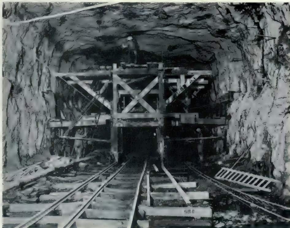
PROGRESS VIEW, SHOWING TUNNEL DURING PERIOD OF CONSTRUCTION.
