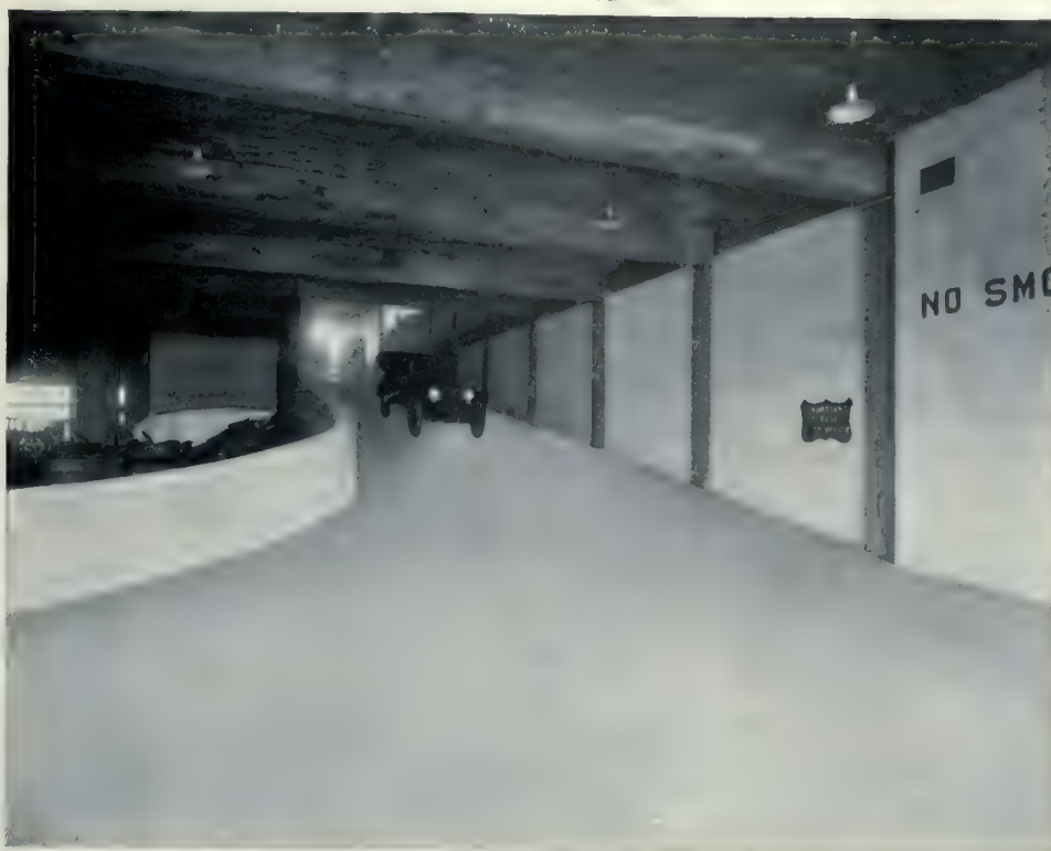
VIEW OF RAMP, OTTAWA CAR COMPANY'S GARAGE, OTTAWA, ONT.
