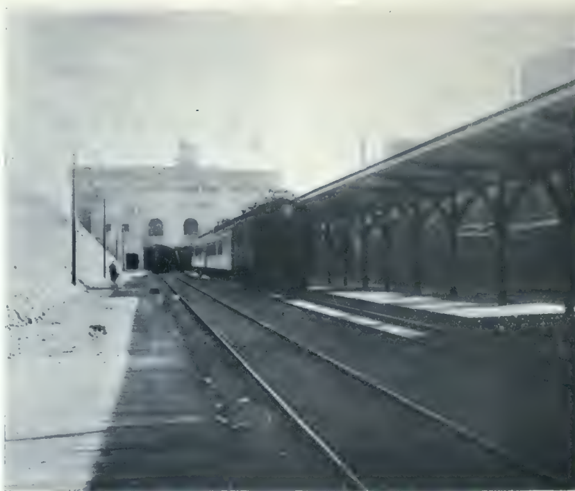
VIEW OF TERMINAL FROM REAR ALONG TRACKS.
