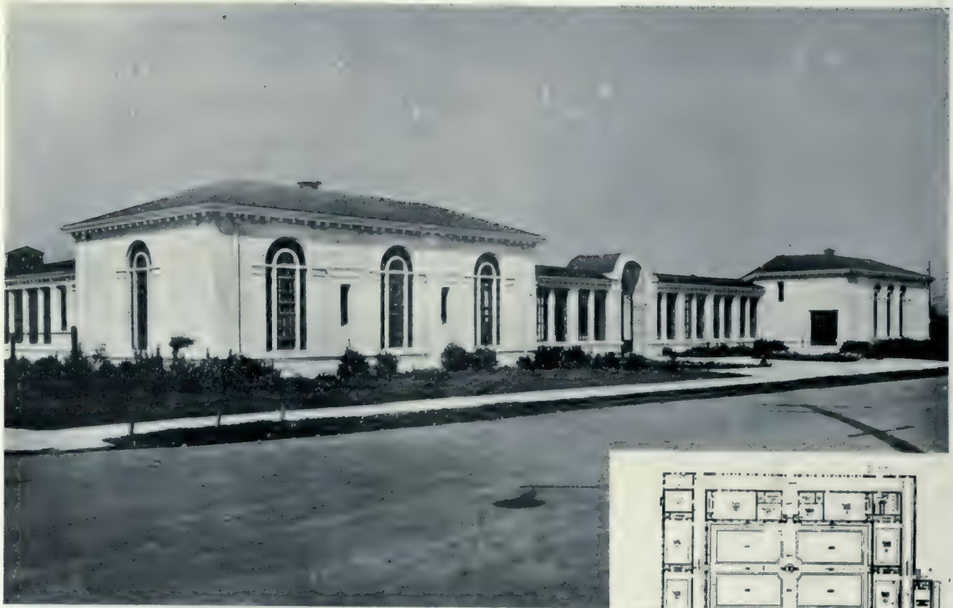
SANTA FE ELEMENTARY SCHOOL, OAKLAND, CALIFORNIA. JOHN J. DONOVAN, ARCHITECT.
