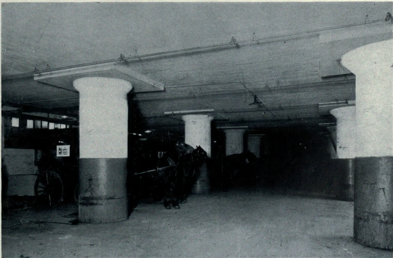
DRIVEWAY UNDER BUILDING AT GROUND FLOOR LEVEL, ROBERT SIMPSON MAIL ORDER BUILDING, TORONTO.
