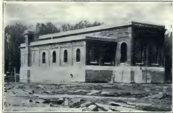
Pumping-Station of Riordan Pulp and Paper Co., Limited, Hawkesbury, Ont. General Contractors: George A. Fuller Co., Limited, Montreal. Roofers: Hickey and Aubut, Montreal.
