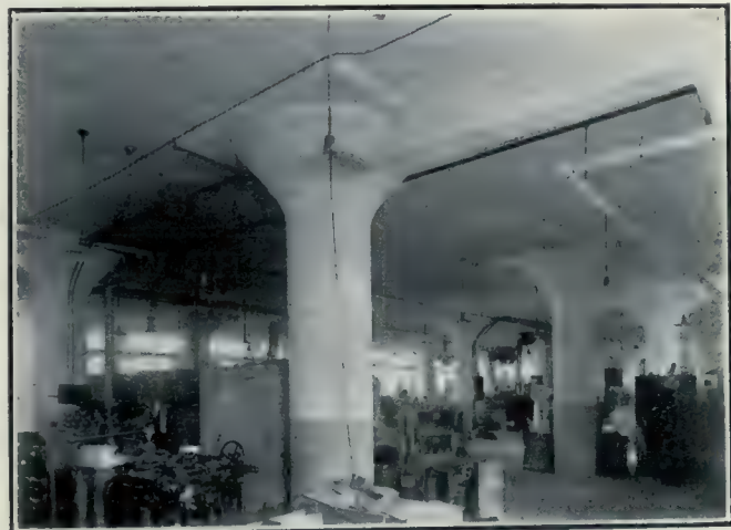
INTERIOR VIEW, SHOWING TYPE OF COLUMNS.
