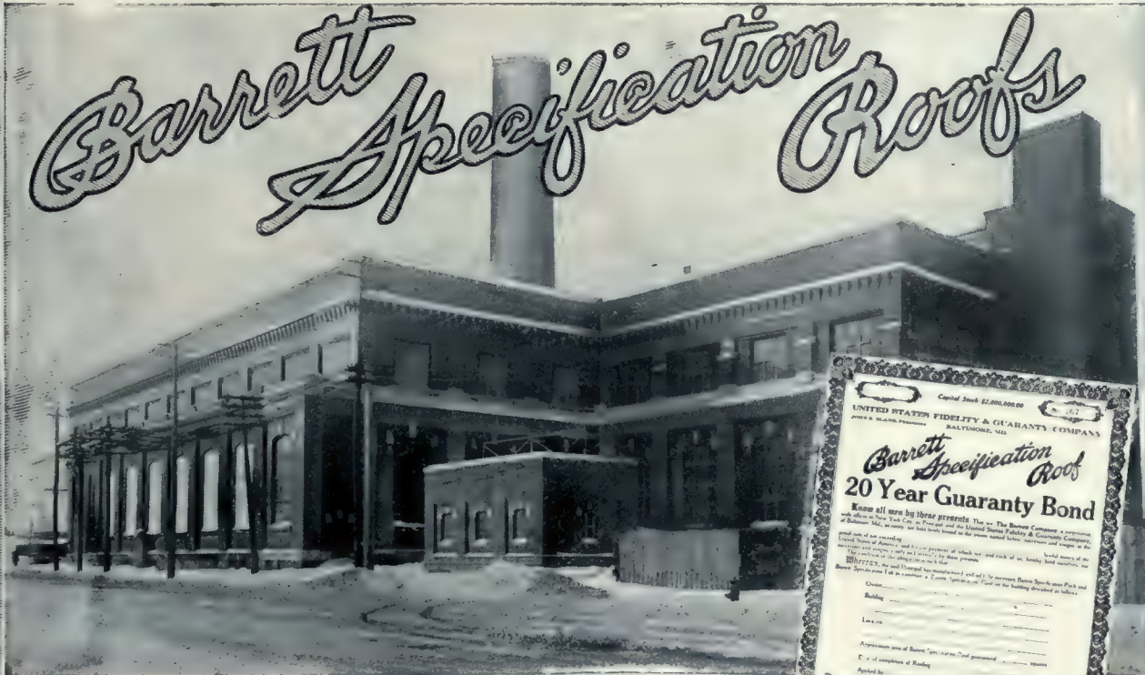
Barrett Specification Roof on Hochelaga Power House, Montreal Tramways Co., Montreal. Roofers: McFarlane Douglas Co., Limited, Montreal; Geo. W. Reed & Co., Limited, Montreal. General Contractors, Raymond Construction Co., Limited; Laurin & Leitch, Montreal.
