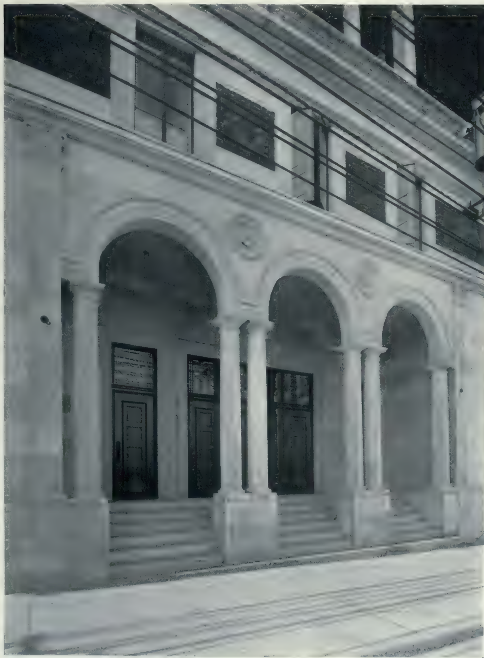
DETAIL OF ENTRANCE.
