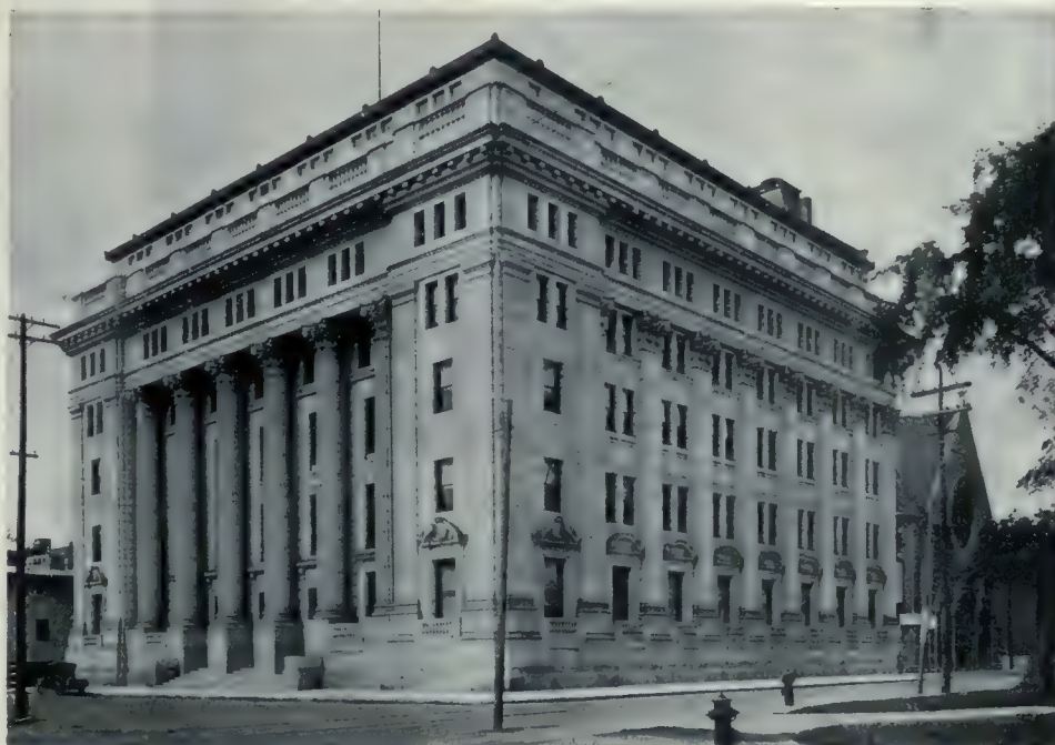
SUN LIFE BUILDING, MONTREAL.
