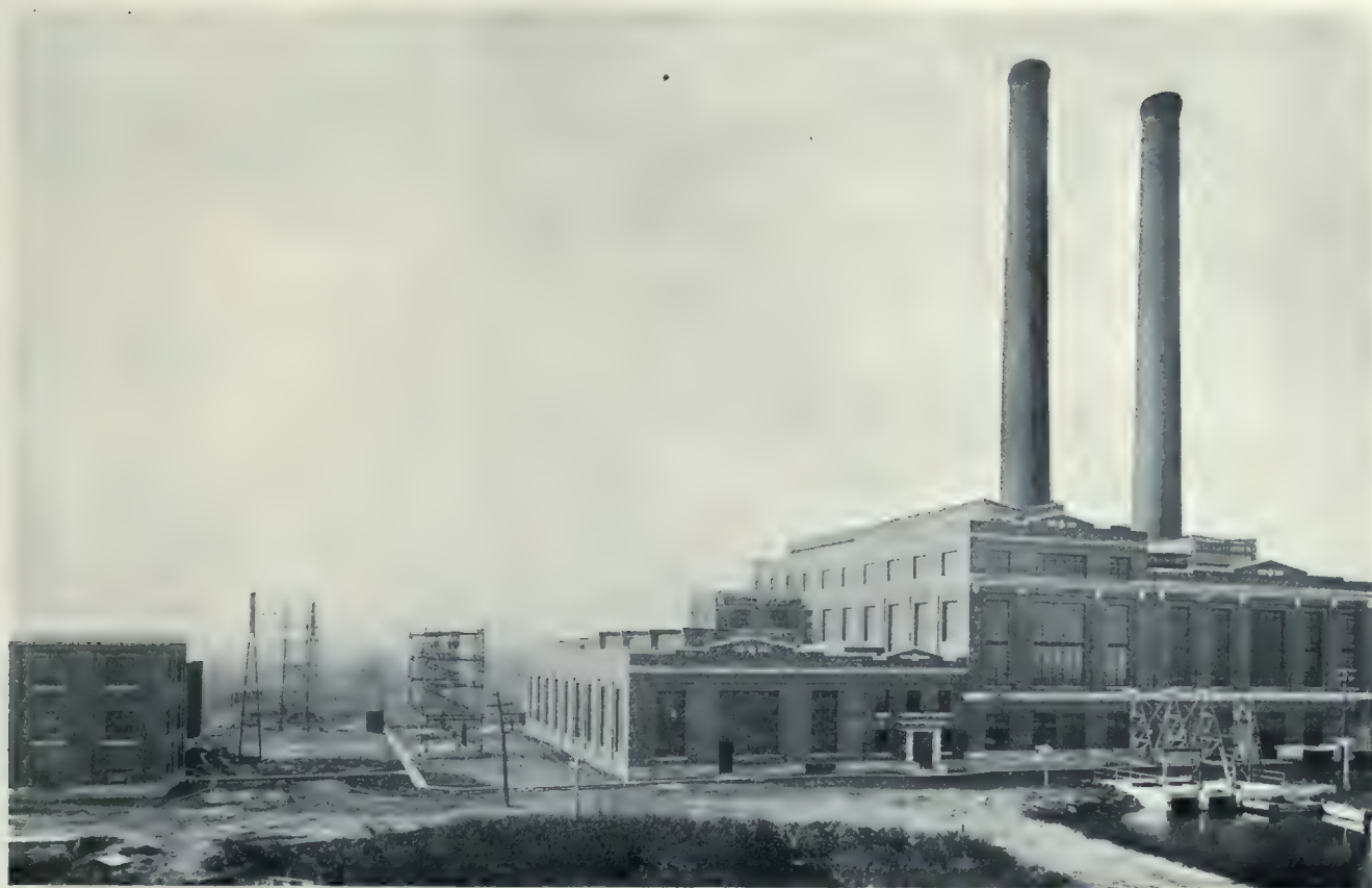
POWER STATION OF DOMINION POWER AND TRANSMISSION COMPANY, HAMILTON, ONT.
