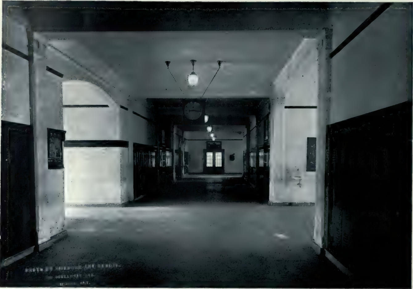
VIEW OF CORRIDOR, COLLEGIATE INSTITUTE, WINDSOR, ONT.
