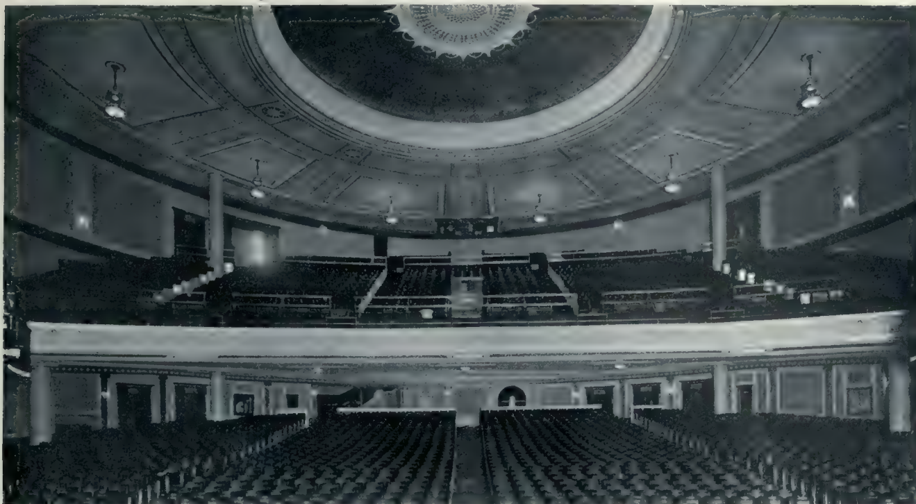
REAR AUDITORIUM VIEW, LOEW'S THEATRE, HAMILTON, ONT.
