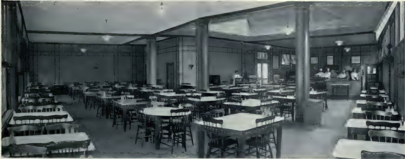
INTERIOR OF CAFETERIA, PORT STANLEY BATHING PAVILLION, WATT & BLACKWELL, ARCHITECTS.
