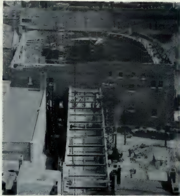
PROGRESS VIEW SHOWING APPROACH FROM STREET.
