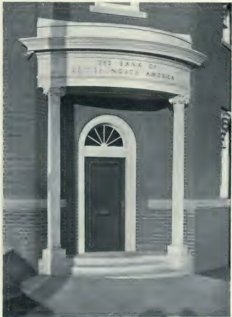
DETAIL OF ENTRANCE.
