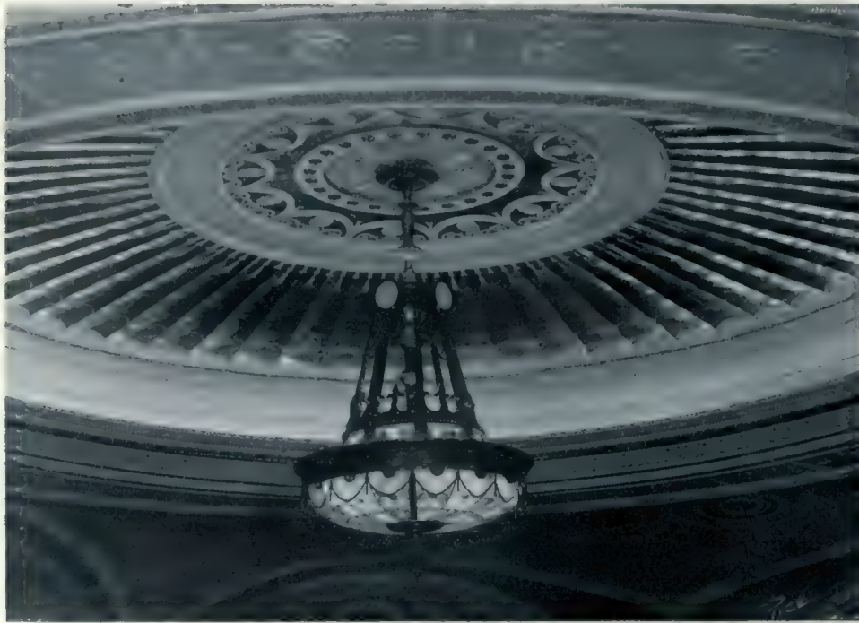
DETAIL OF CEILING, LOEW'S THEATRE, MONTREAL.
