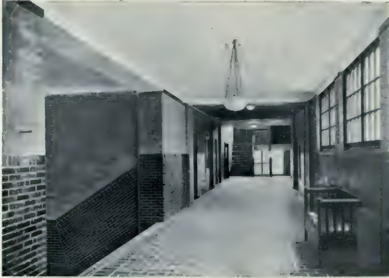
MAIN CORRIDOR, TECHNICAL SCHOOL, LONDON.
