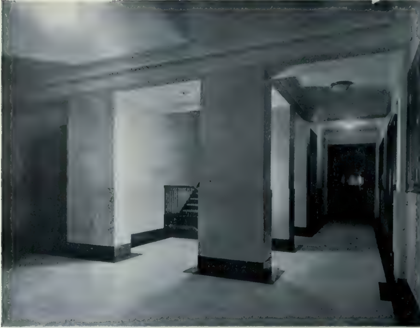
TYPICAL UPPER CORRIDOR.
