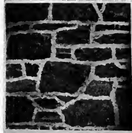
Fig 2. Rough Rubble - large white, roughly pointed joints
