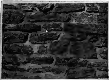
Fig 4. Rough Rubble, or ledged work Raked joints.
