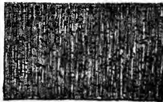
Finish made by the Bush Hammer
