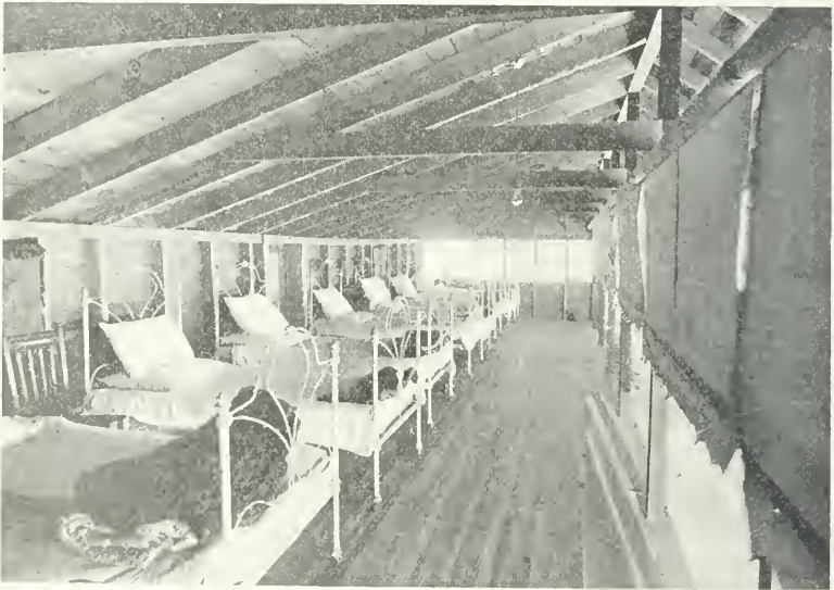
FIG. 54—Interior of old lean-to. Sleeping quarters, Loomis Sanatorium Annex.
