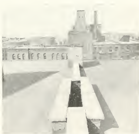
FIG. 32.—An air-shaft 12 inches wide and six floors deep.
