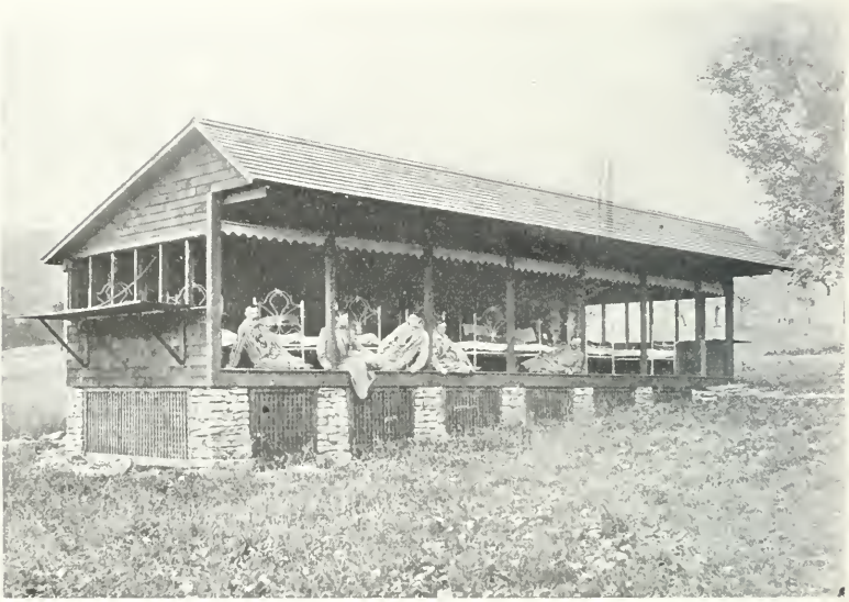
FIG. 68—Original lean-to at Loomis Sanatorium, eight patients.
