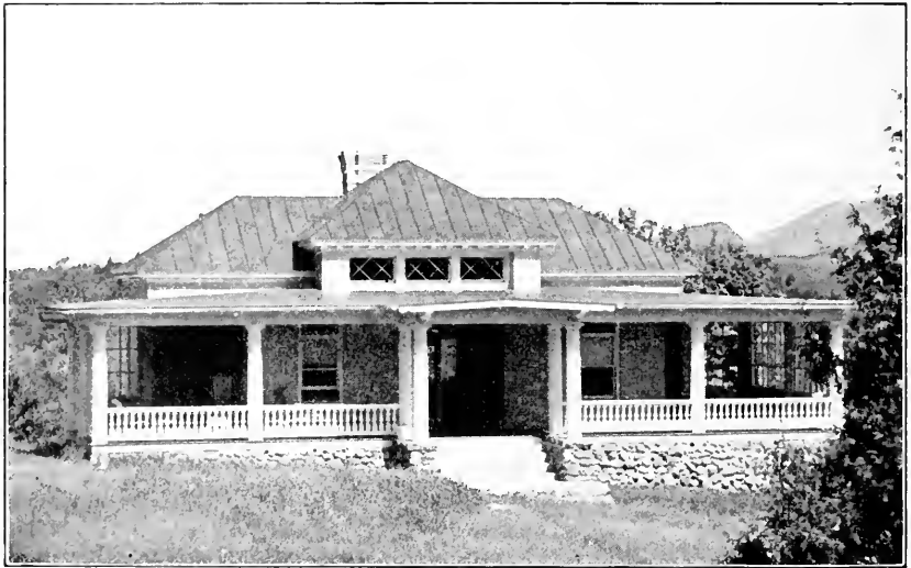
FIG. 56—Nathan cottage, Adirondack Cottage Sanatorium.
