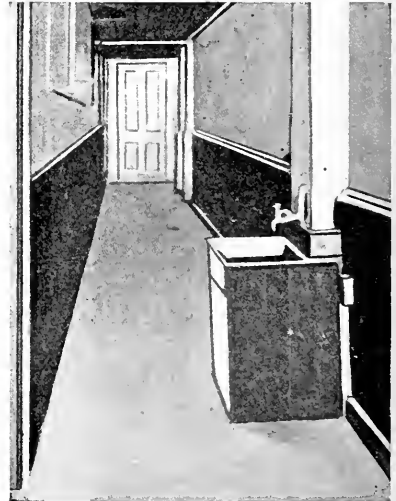
FIG. 101.—The same hall and sink as the Department left them.
