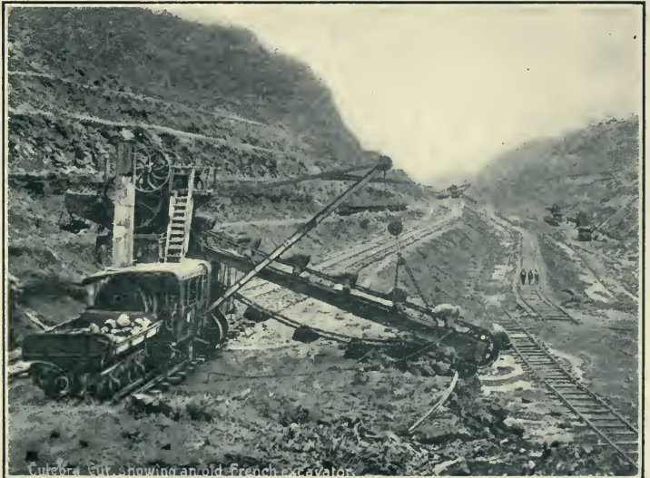
Culebra Cut, showing an old French excavator.
