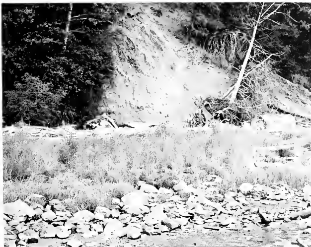
Figure 5. Landslide exposure of upper part of the Lincoln Creek Formation along the Columbia River.
