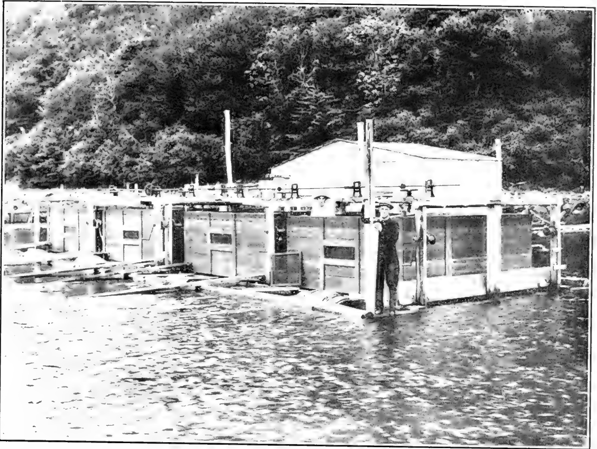
Fig. 1.—Rearing plant viewed from the east side. The four rearing or hatching boxes have been lifted out of the water. Side windows, 4 feet by 1 foot, are shown at the sides. Mr. Dawson is holding one of the paddles upright. The engine house is in the background.
