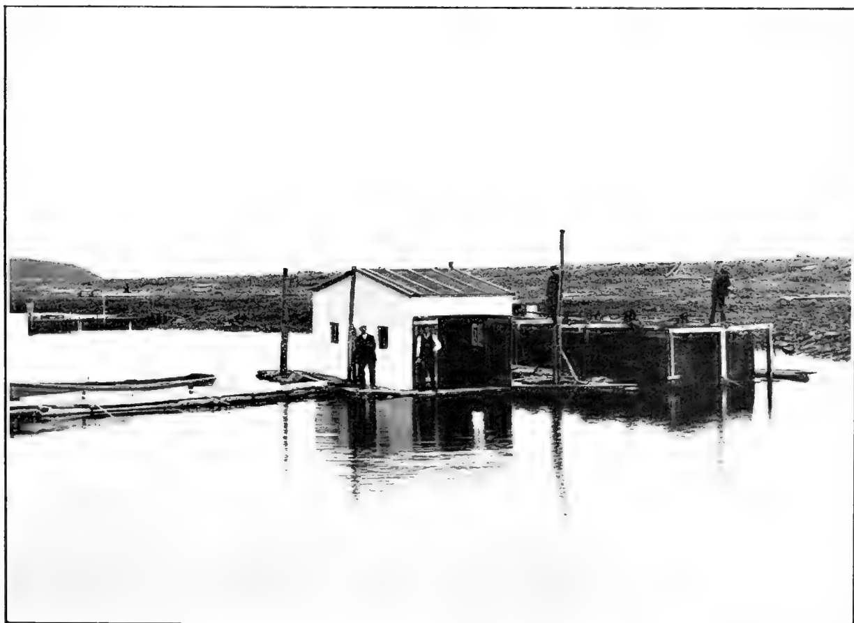
Fig. 2.—The plant viewed from the southwest side. A floating walk connects the engine house with the shore. The tall piles hold the rafts in place. The sea-wall is seen in the background.
