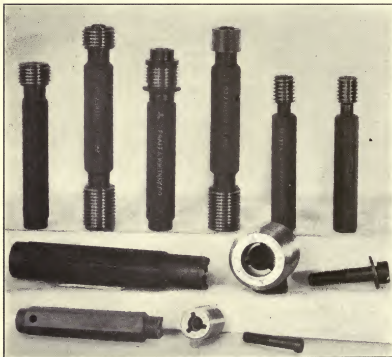
Figure 75. Typical Thread Gages—Pratt and Whitney Company
