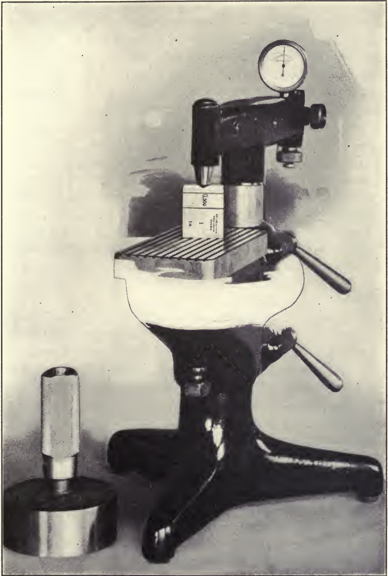
Figure 69. American Amplifying Gage Used with Swedish Gage Blocks
