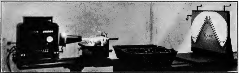
Figure 77. General View of Hartness Screw Thread Comparator
