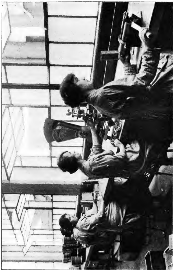
Figure 41. Piston Ring Inspection—Packard Motor Car Company
