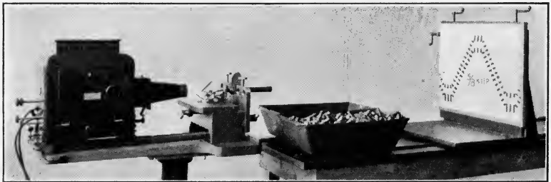
Figure 78. Another General View of Hartness Screw Thread Comparator
