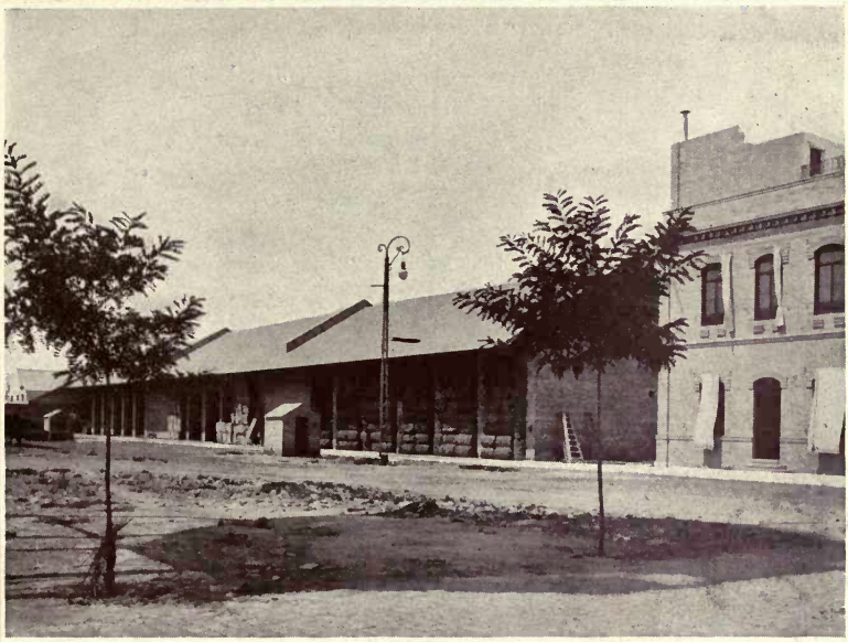
One of the Corkwood Warehouses, Seville Plant
