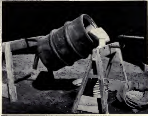
FIG. 19.—A SEED-TREATING MACHINE MADE FROM A STEEL OIL DRUM
