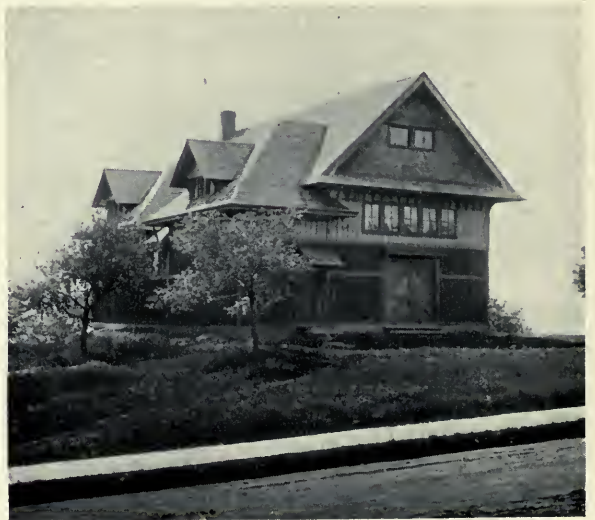
The Old Gymnasium Remodeled
