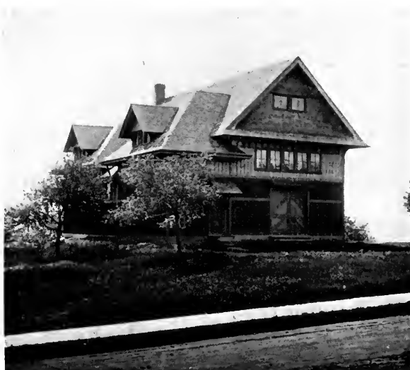
The Old Gymnasium Remodeled
