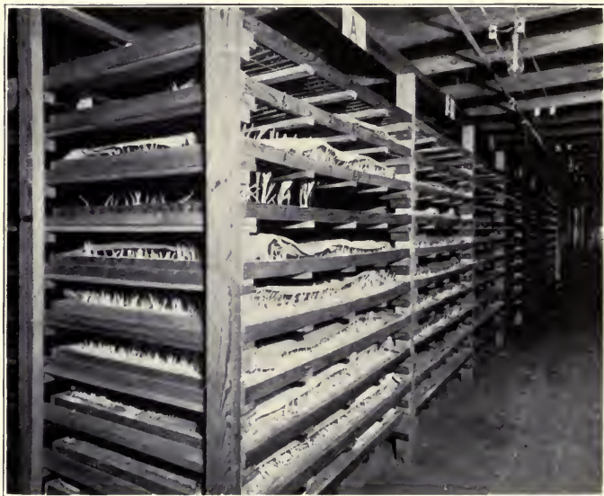
FIG. 55.—MULTIPLE TRAY GERMINATOR IN OPERATION
