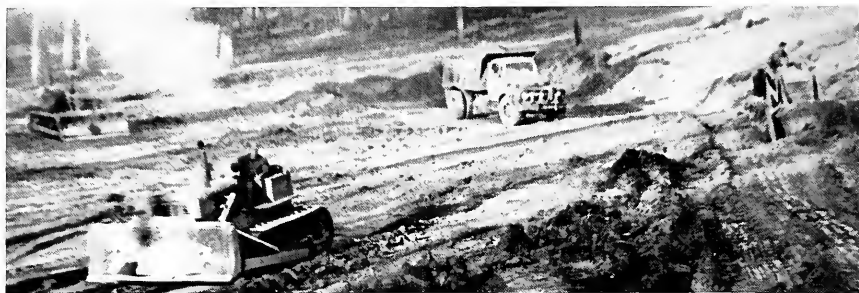
Excavation in progress.
