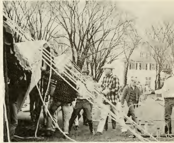
The work crew
