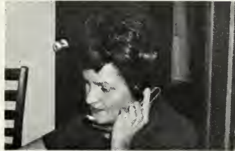
La Verna Coulton Switchboard
