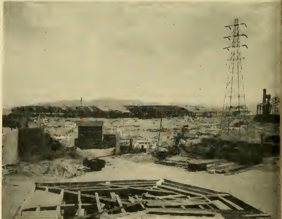
PHOTO No. 3.— Looking south toward engine-parts assembly shops. Most damage occurred in 19 January 1945 attack by 500-lb. HEs.
