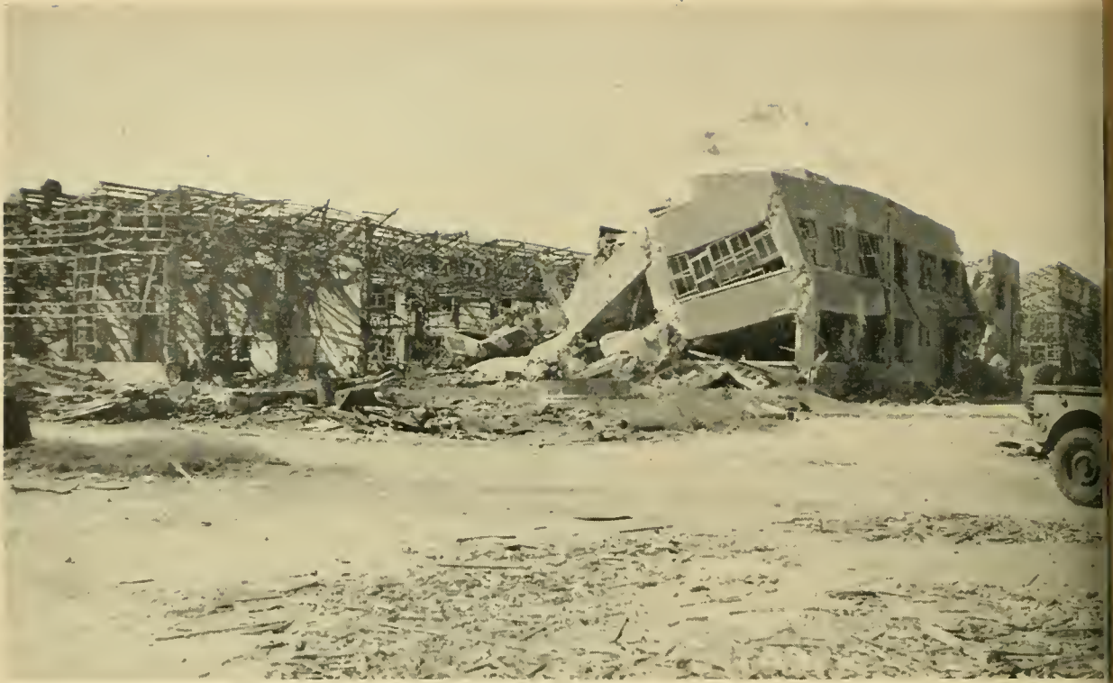
PHOTOS 4-9.—Views of Akashi plant buildings damaged and destroyed by June 1945 attacks in which 4,000-lb. H fused instantaneously were used.
