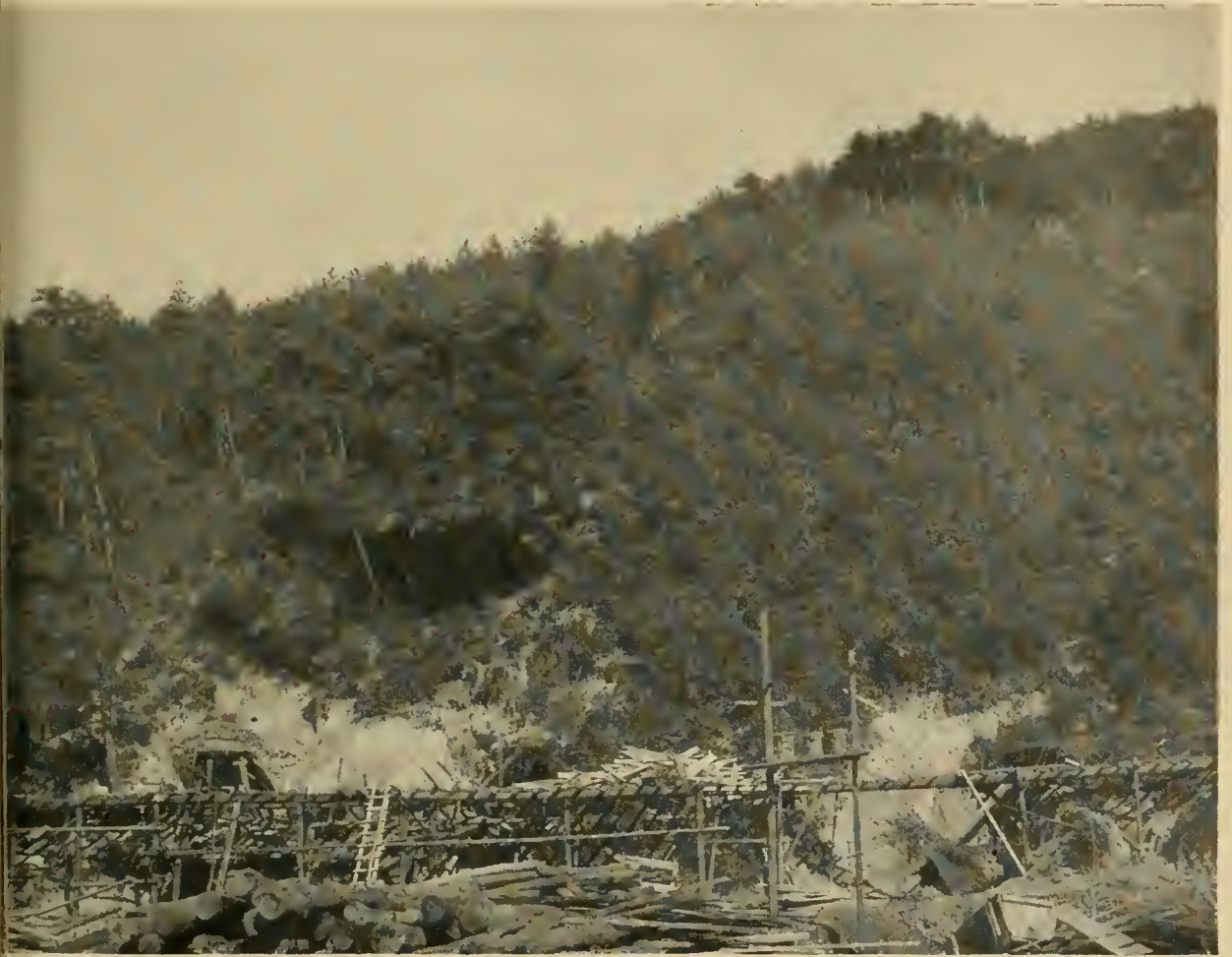
PHOTO 12.—Trellis at Takatsuki for hauling machinery to tunnels.
