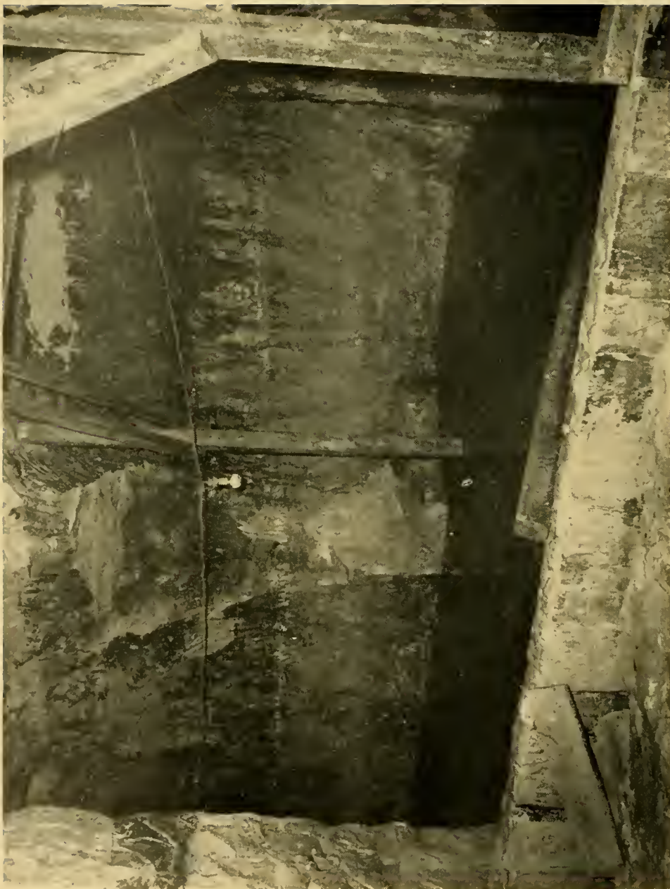
Photo No. 44. Flooded tunnel at Hisai.
