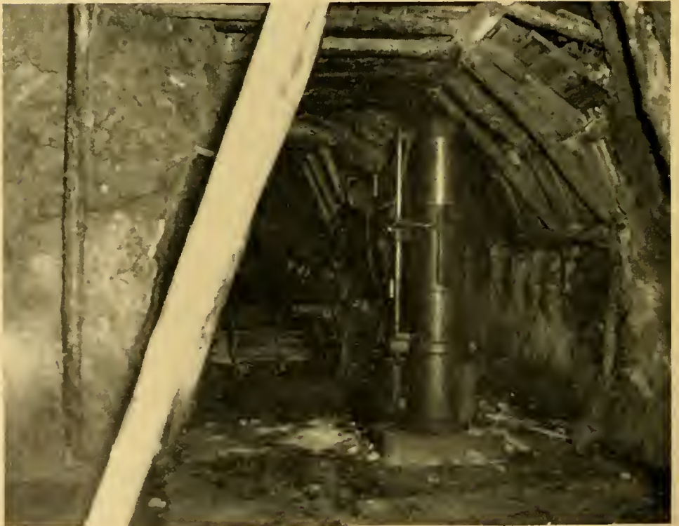
Photo No. 33. Machine tools in position, Yoshimatsu.
