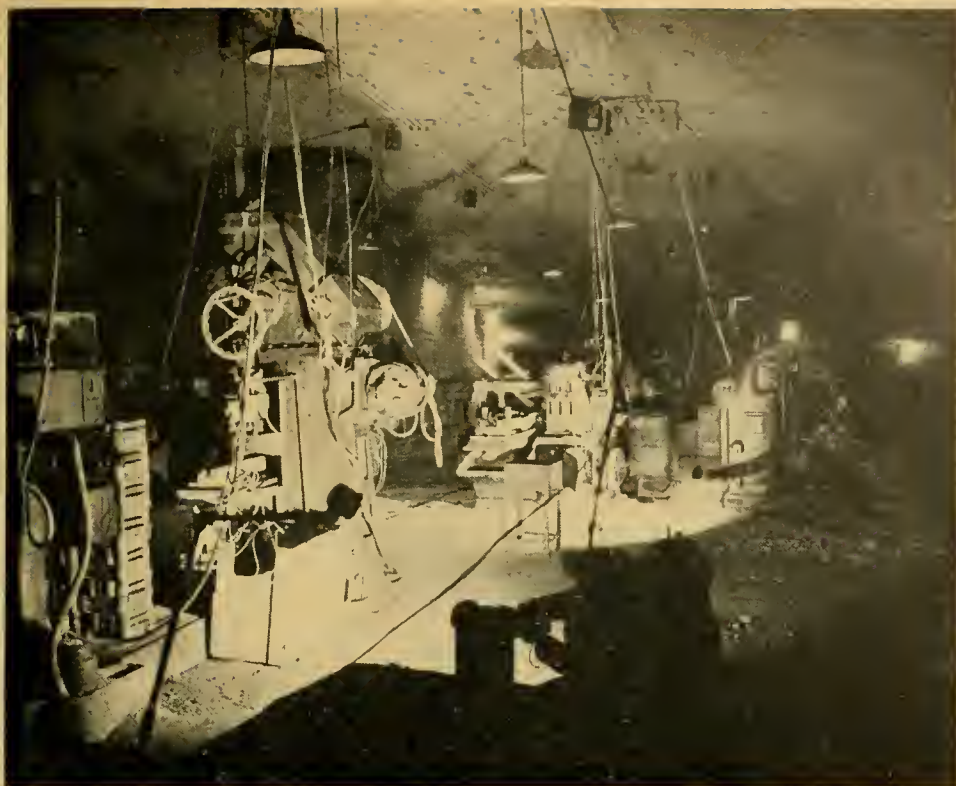
Photo No. 7. Articulating rod shop, Bente plant at Oya Works.
