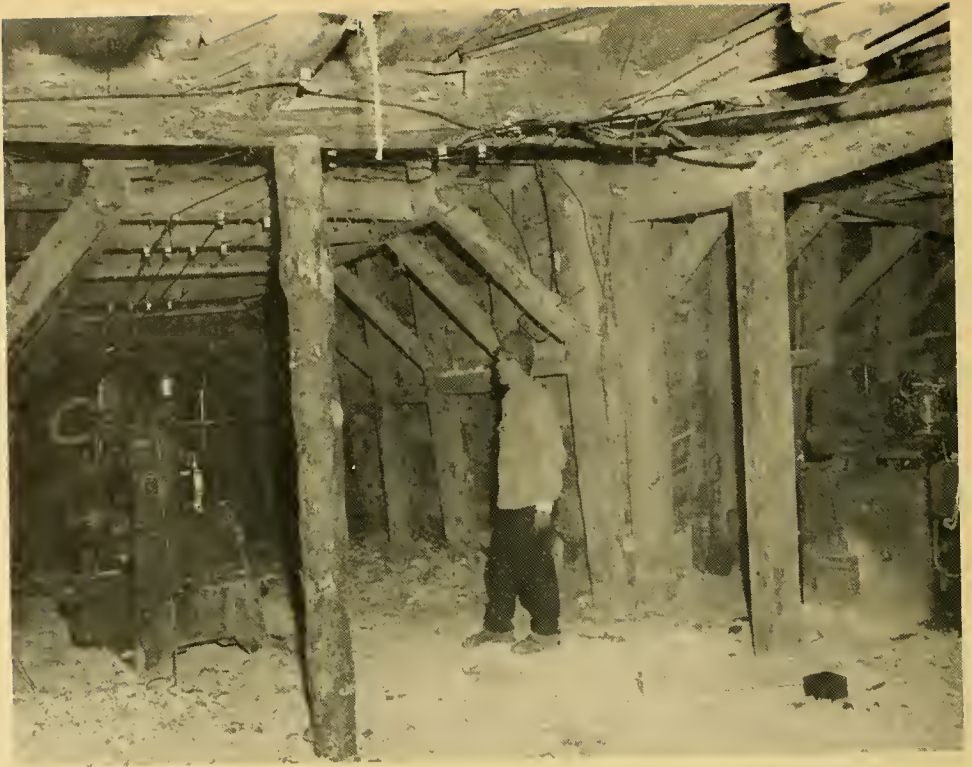
Photo No. 58. Seto plant. (Note extensive shoring.)
