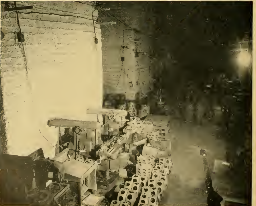
Photo No. 2. Crankcase shop, Tomura plant at Oya Works.
