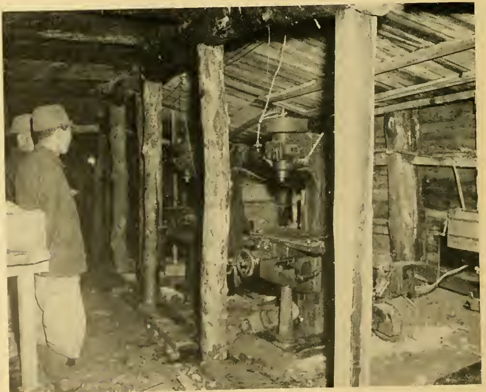
Photo No. 59. Seto plant. (The tight working quarters shown here were not uncommon.)
