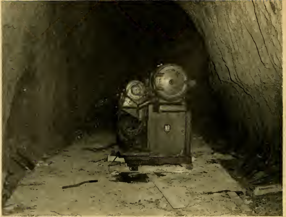
Photo No. 32. Machine tool in process of installation, Yoshimatsu.
