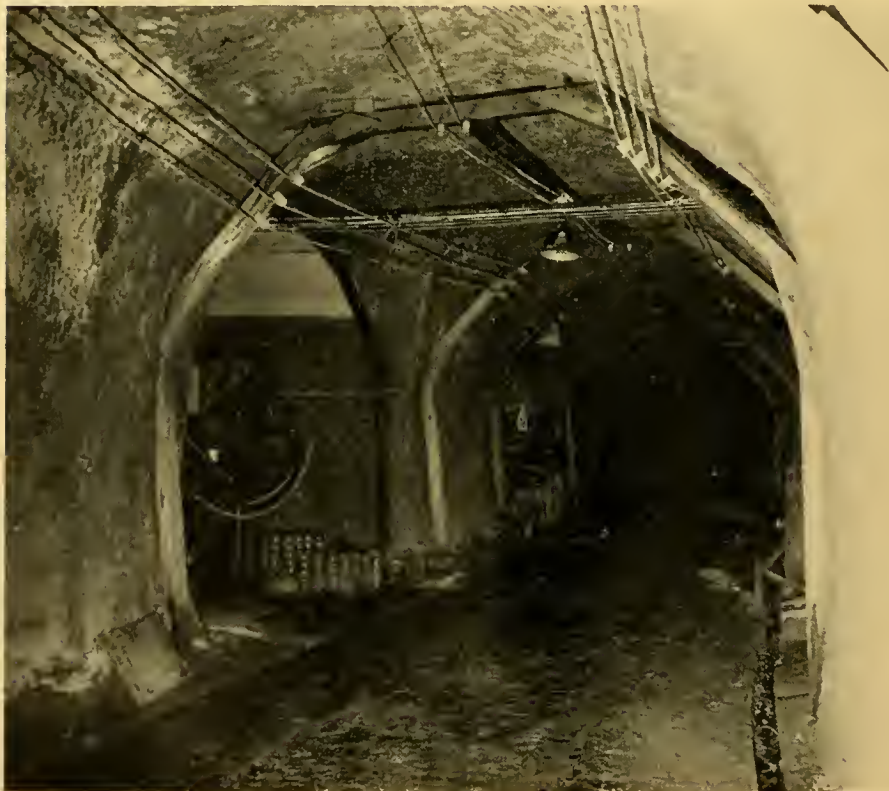
Photo No. 51. Handa plant. (Note production tunnels opening into communications tunnel.)
