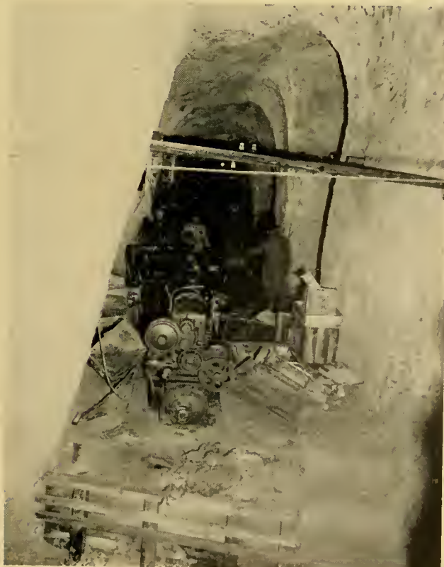
Photo No. 46. Interior at Hisai.
