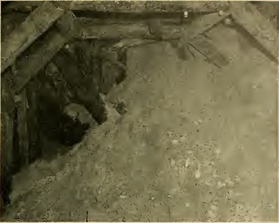
Photo No. 52. Cave-in of machine shop at Seto.
