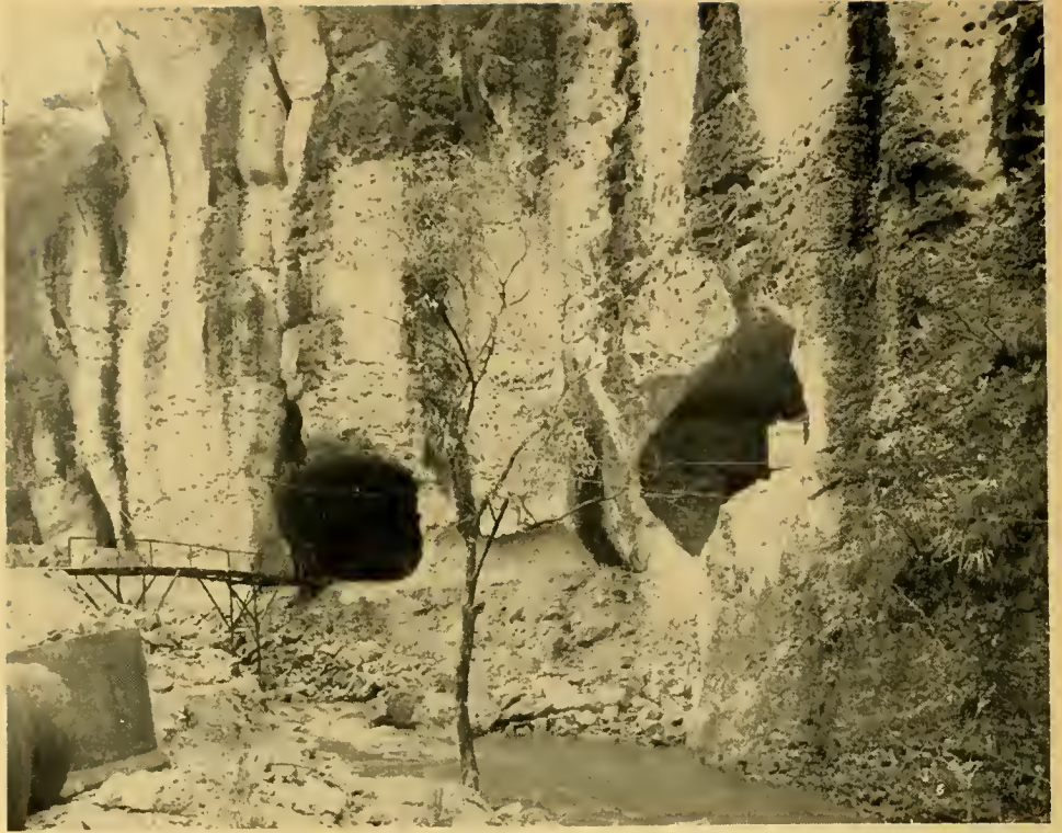
Photo No. 11. Tunnel entrances (Otomeyama plant), Shiroyama.
