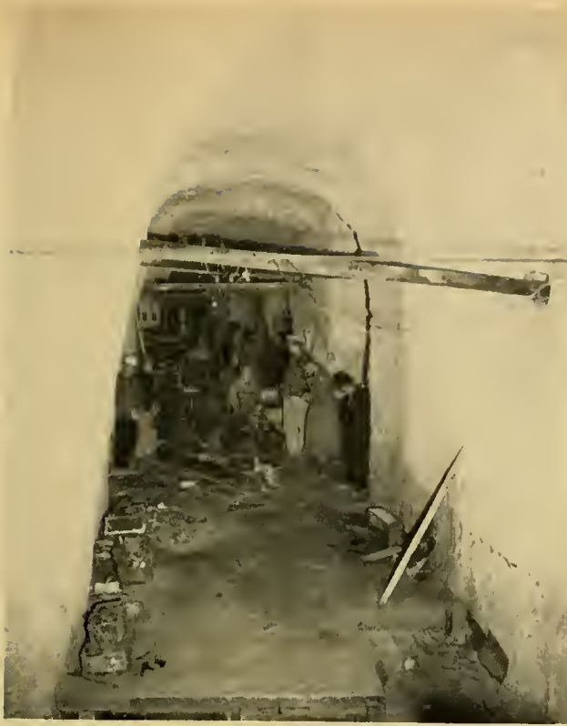
Photo No. 45. Interior at Hisai.
