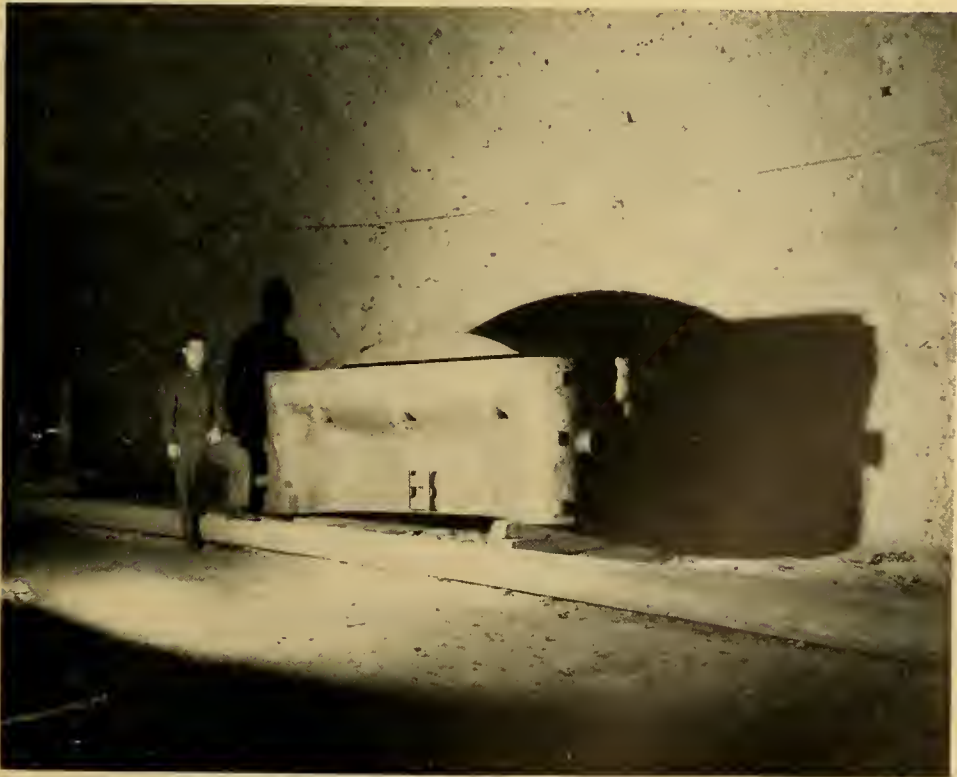
Photo No. 14. Part of 20-ton press (Otomeyama plant), Shiroyama.
