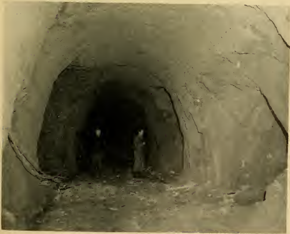
Photo No. 31. Tunnels at Yoshimatsu.
