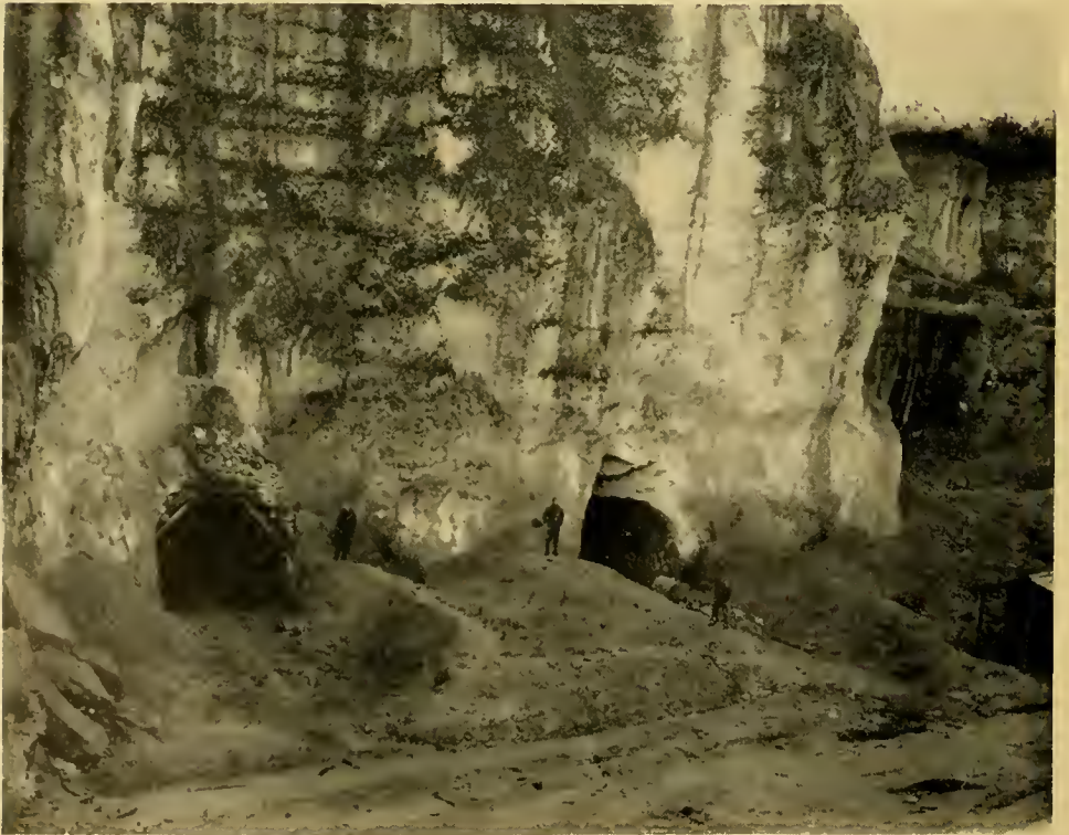
Photo No. 29. Entrances to tunnels. Yoshimatsu.
