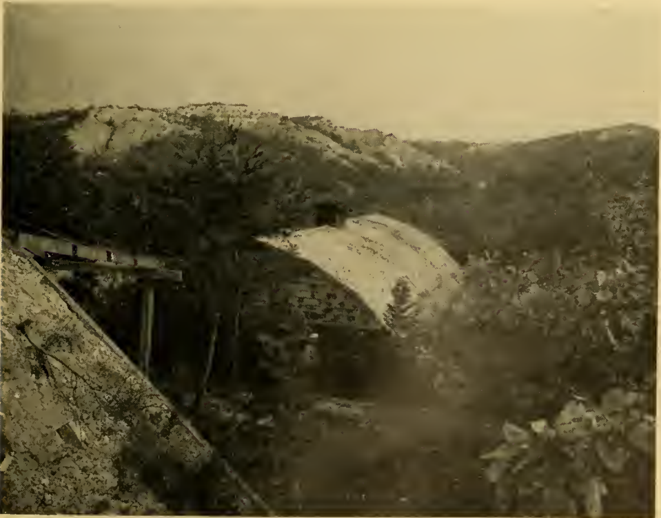
Photo No. 57. Surface building at Seto.
