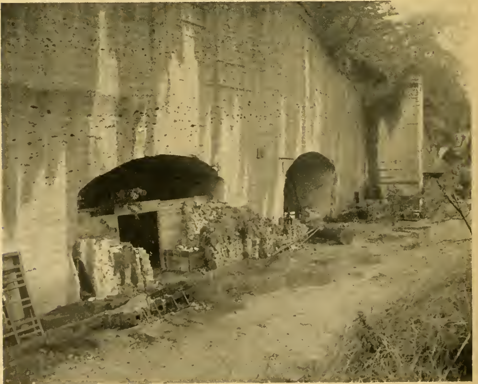
Photo No. 12. Tunnel entrances (Otomeyama plant), Shiroyama.
