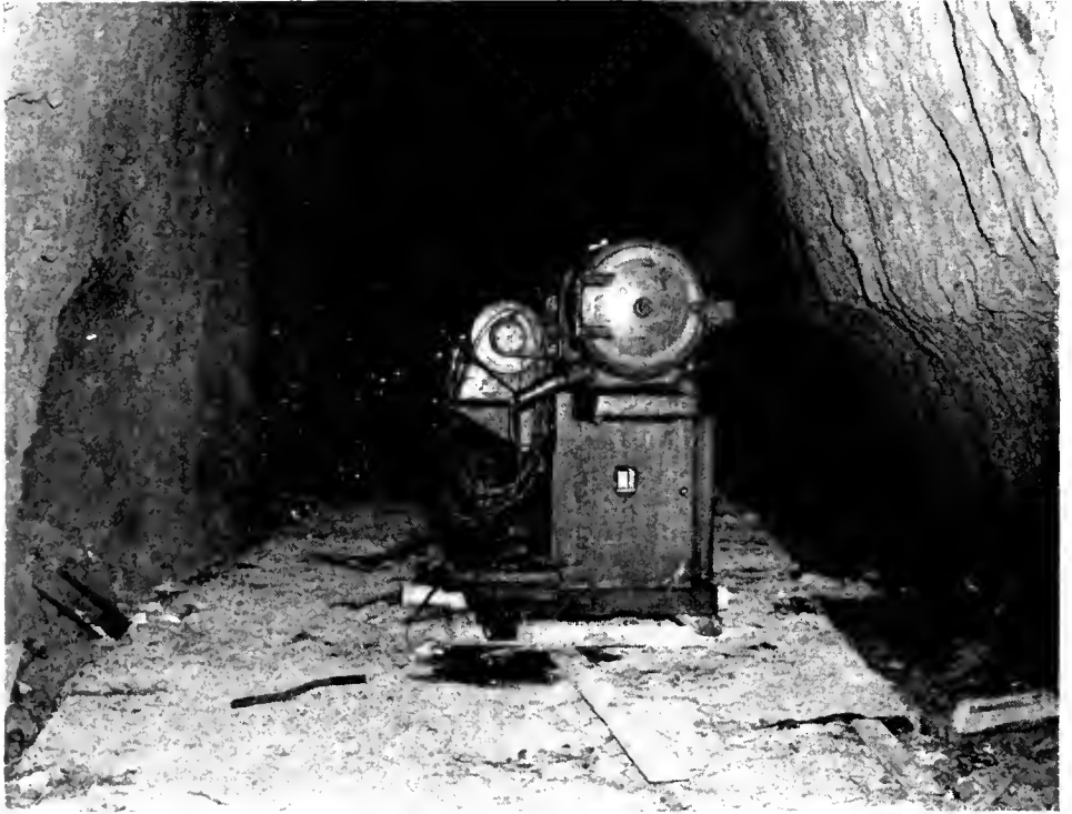
Photo No. 32. Machine tool in process of installation, Yoshimatsu.
