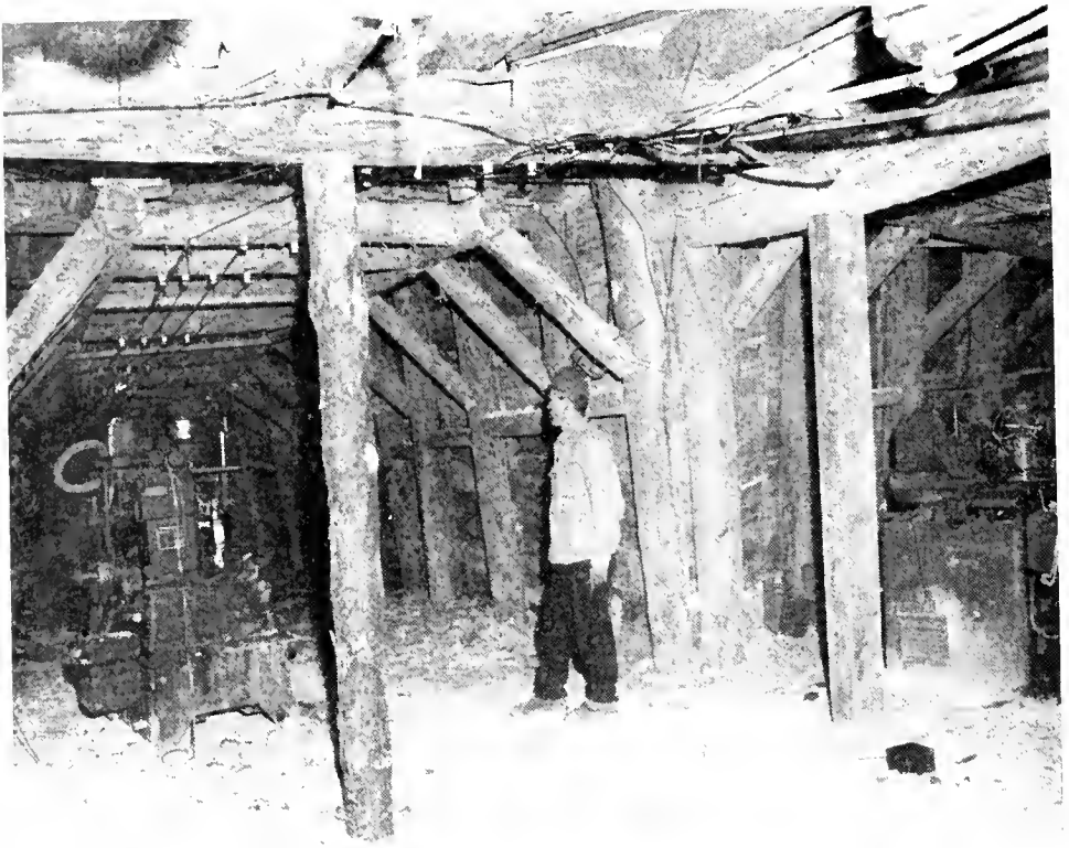
Photo No. 58. Seto plant. (Note extensive shoring.)
