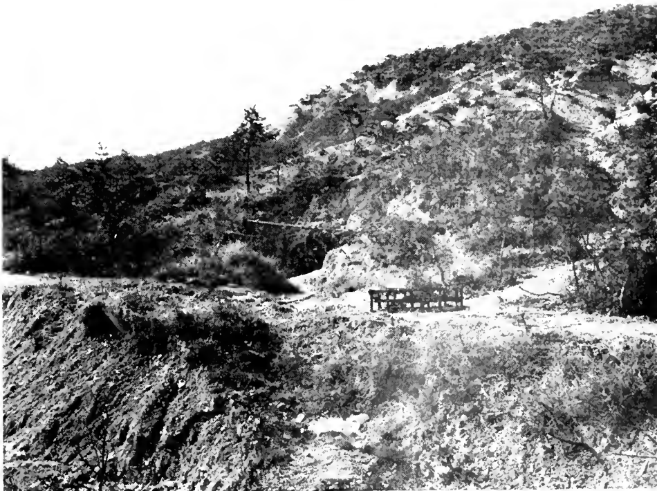
Photo No. 53. Entrance in spur of hill at Seto.
