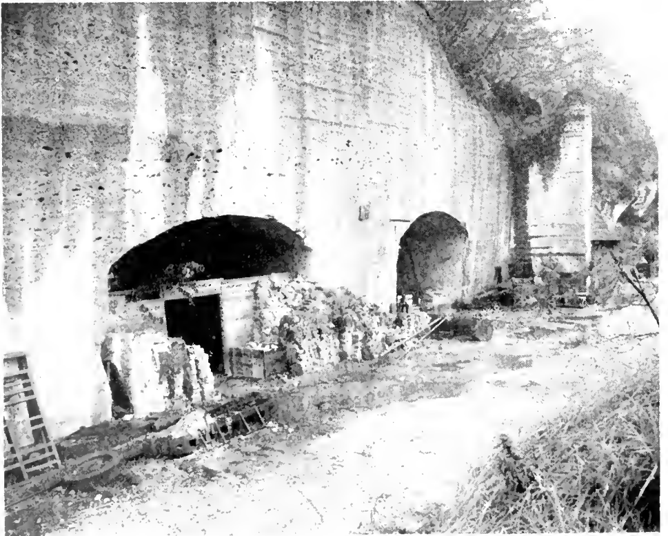
Photo No. 12. Tunnel entrances (Otomeyama plant), Shiroyama.
