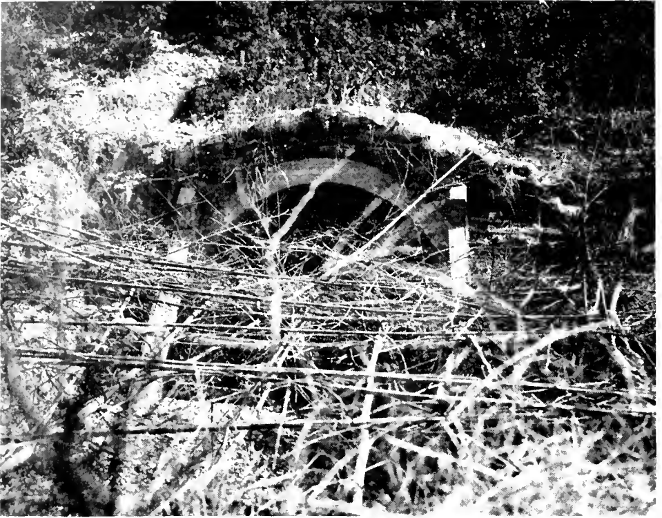
Photo No. 54. Camouflaged entrance at Seto.
