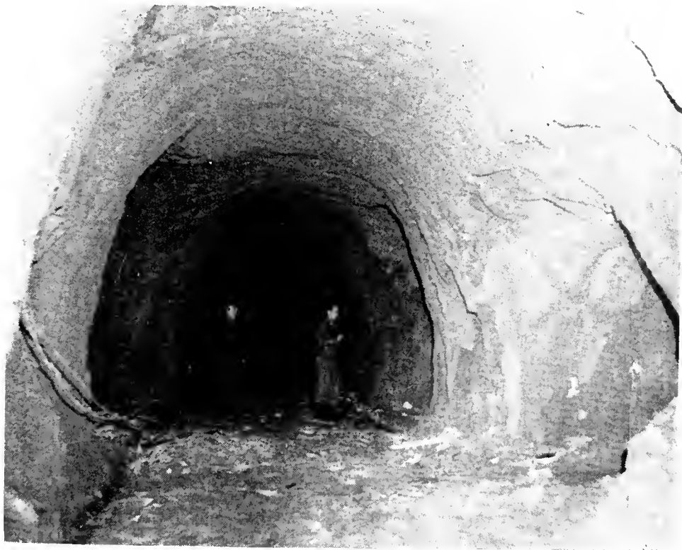
Photo No. 31. Tunnels at Yoshimatsu.
