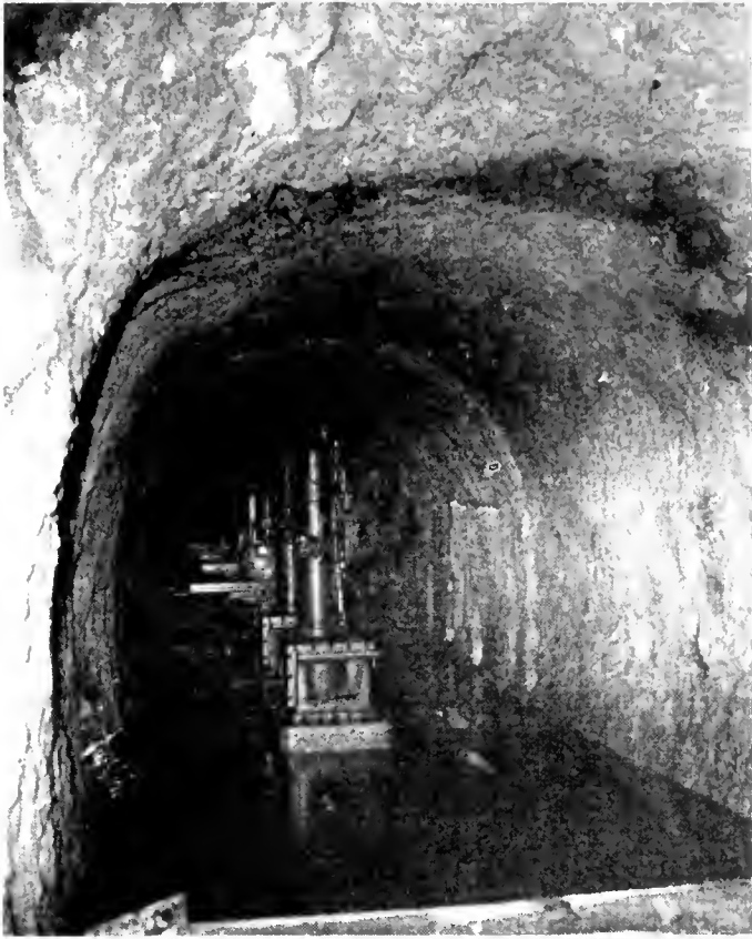
Photo No. 34. Machine tools standing in water. Landslide had formed a dam near entrance.
