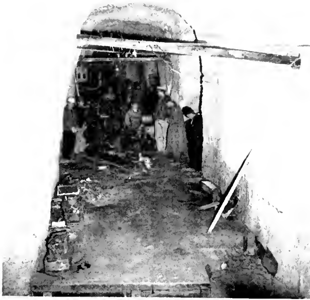
Photo No. 45. Interior at Hisai.
