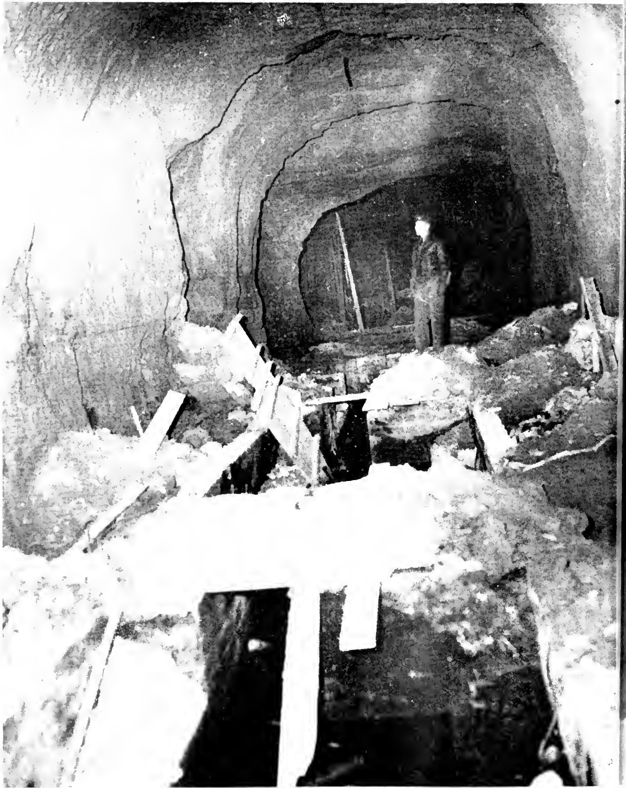
Photo No. 36. Heat treatment pits under construction, Yoshimatsu.
