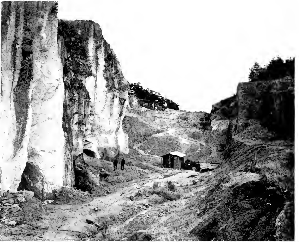
Photo No. 28. Entrance to Nakajima tunnels at base of cliff, Yoshimatsu.
