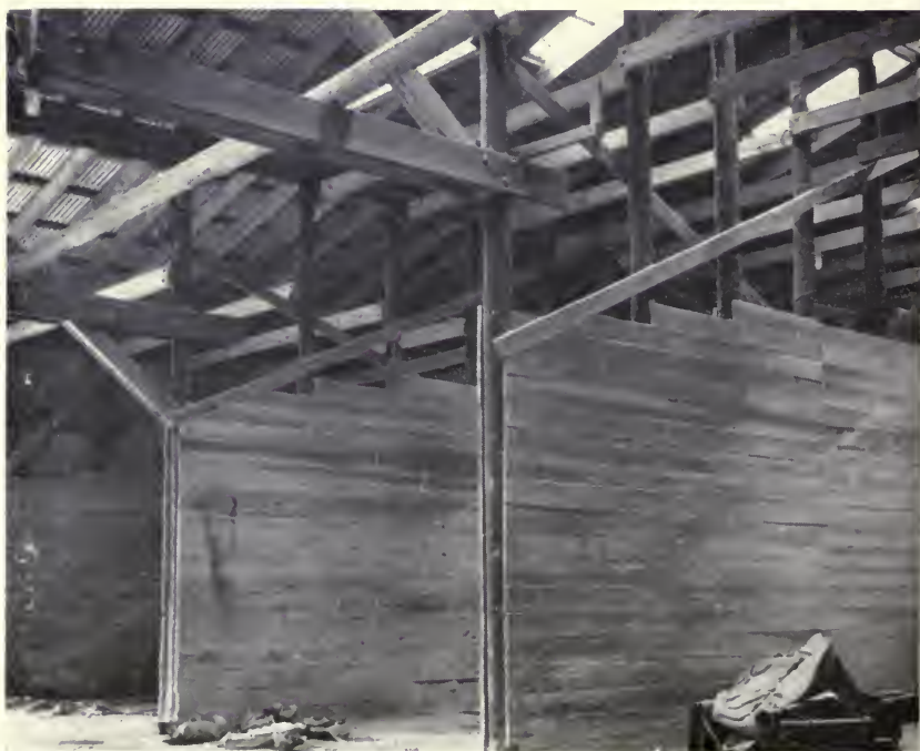
Storage-bin walls are usually lined to a height of 10 feet. Material may be piled higher than the wall height. (Fig. 8)
