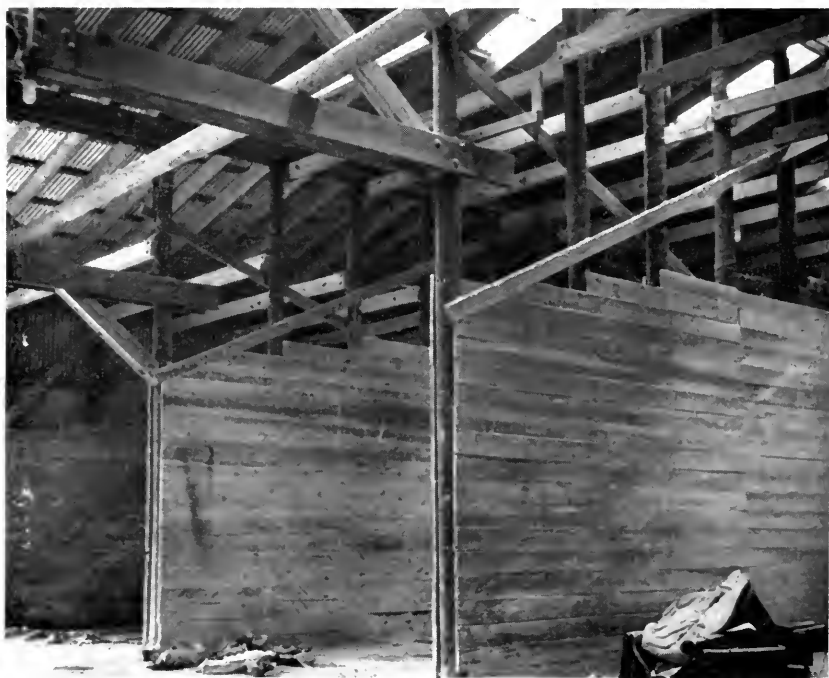
Storage-bin walls are usually lined to a height of 10 feet. Material may be piled higher than the wall height. (Fig. 8)
