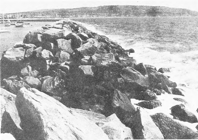
Figure 1. A rubble-mound breakwater protecting a boat harbor
