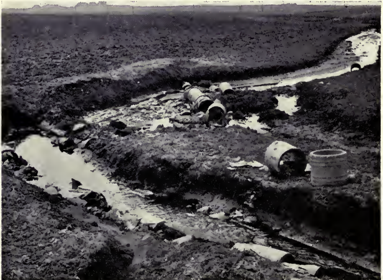
A washed out tile line makes greater inroads each year into farm income. Crops and cropland are lost, and repair becomes more costly. A grass waterway in this natural drainageway would have prevented this gully. Tile seldom work in these slowly permeable soils. (Fig. 17)
