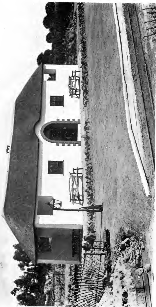
WAYSIDE STATION OF PISÉ AT SIMONIUM, SOUTH AFRICA, DESIGNED BY MR. HERBERT BAKER.
