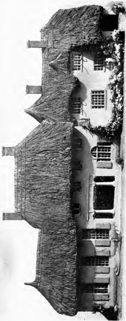
MODEL OF A PISÉ DE TERRE HOUSE TO BE BUILT IN THREE SUCCESSIVE STAGES.
