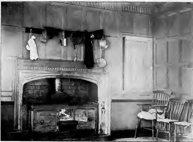
THE LODGE. PANNELED ROOM
