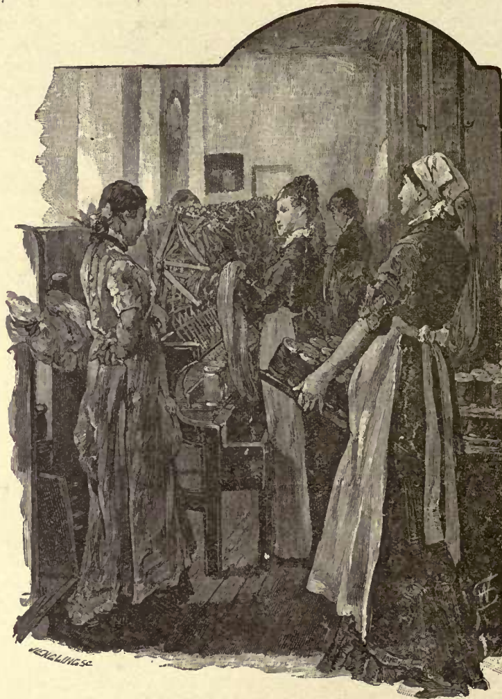
A SPOOLING ROOM.
