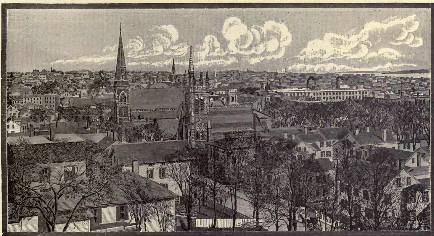
VIEW OF FALL RIVER FROM THE HIGH SCHOOL BUILDING.
