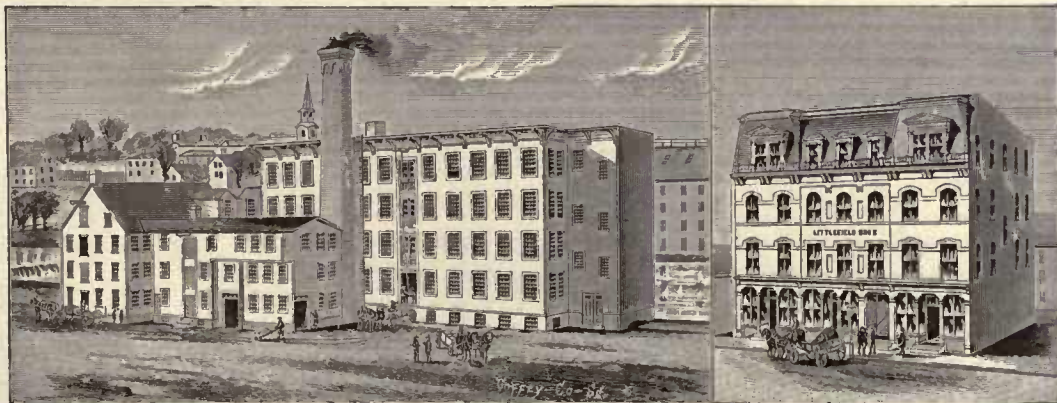
MILL AND OFFICE OF LITTLEFIELD MANUFACTURING COMPANY, PAWTUCKET.
