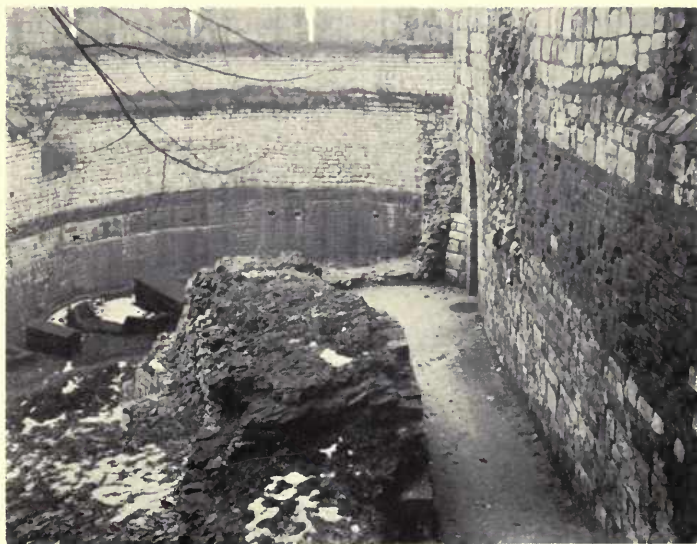
INTERIOR OF THE MULTANGULAR TOWER, YORK.
