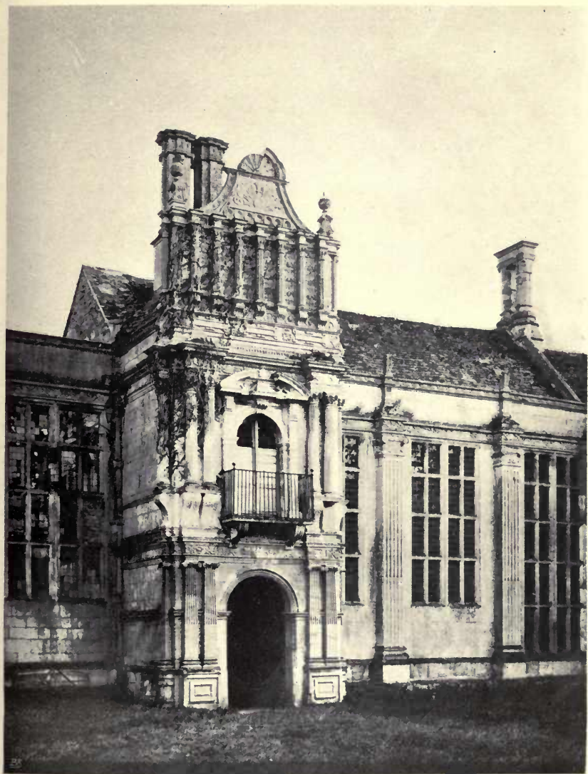
HALL PORCH, KIRBY.
