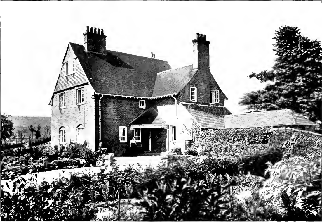
COTTAGE AT SUTTON VENY, WILTS: ENTRANCE FRONT. (See previous page.)
