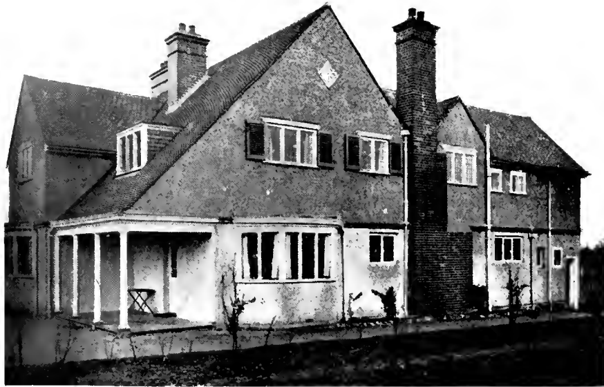
GENERAL VIEW FROM GARDEN
