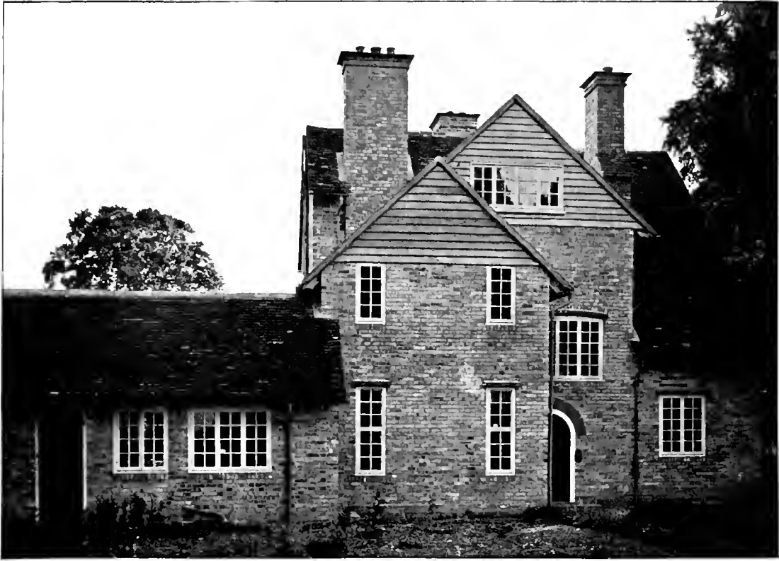
ENTRANCE FRONT. Photograph by W. H. Watts.
