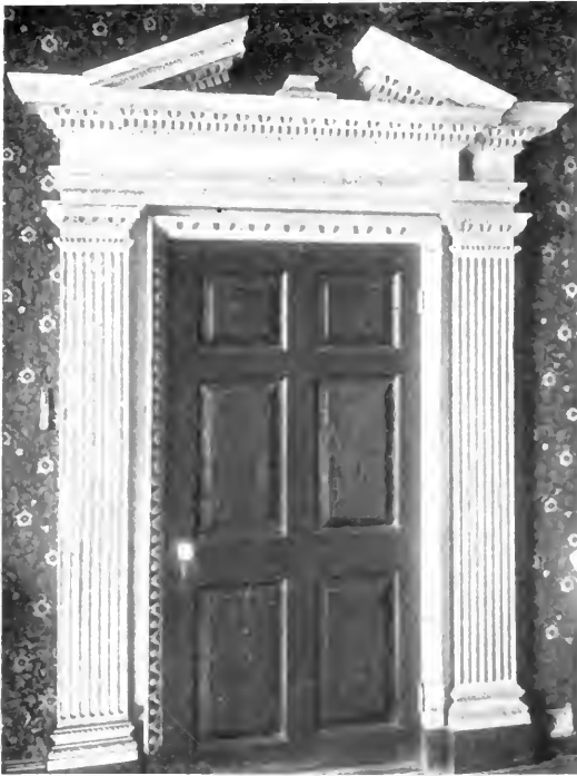
Interior doorway at "Gunston Hall," Virginia. A good example of the straight, interrupted pediment. A bust is supposed to occupy the space at the top
