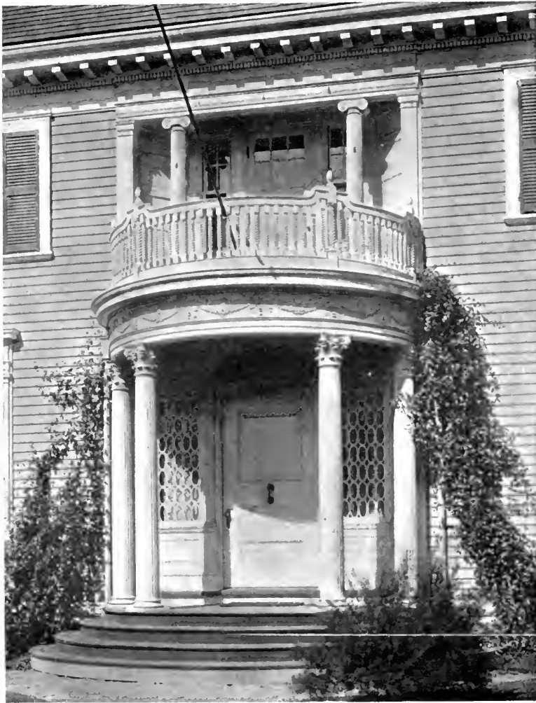
Entrance motive to house at Cambridge, Mass. The recessed windows above give added space to the balcony. The side lights below are rich and simple
