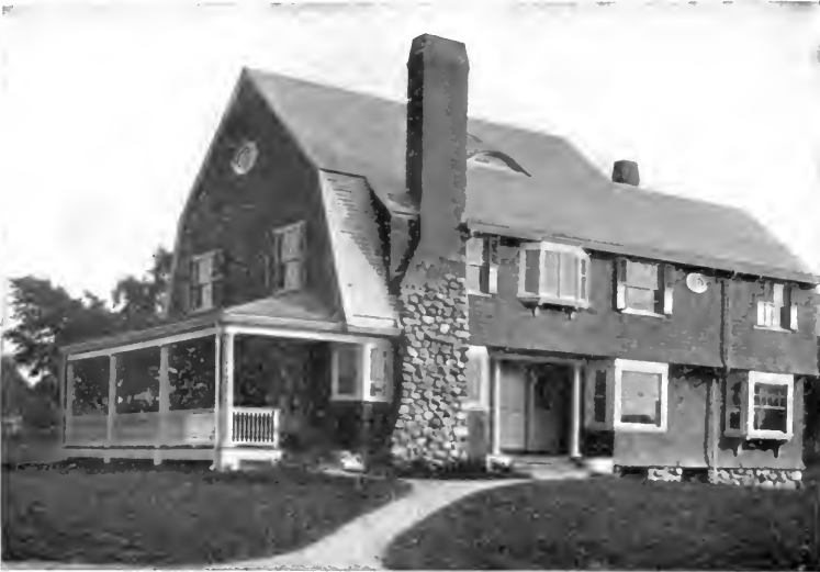
House at Chestnut Hill, Mass., showing the transition of the gambrel to the pitch roof; the cottage to the two-story effect
