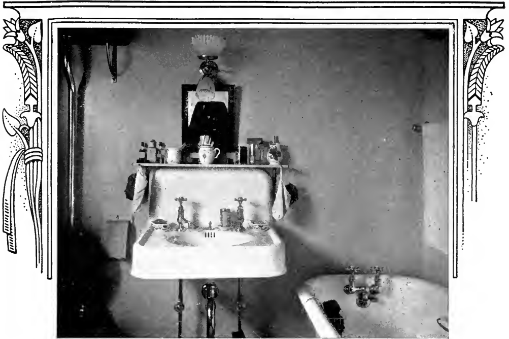
Portion of a small bathroom showing enamelled lavatory and tub, with painted walls
