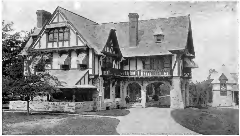
An excellent adaptation of English and French half-timber work. Cost about $17,000. Wm. L. Price, architect
