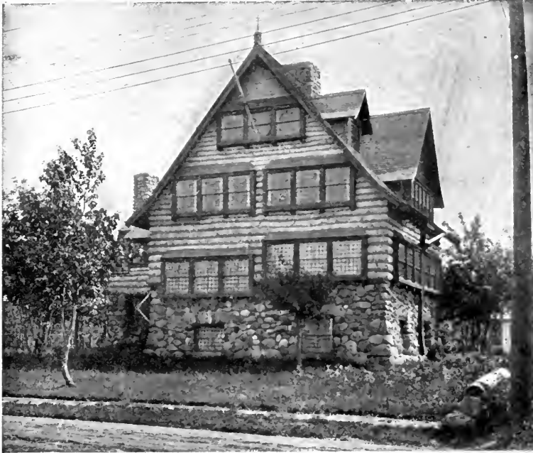
Log and stone house at Bar Harbor, Me. Designed and built by a local carpenter, and very suggestive despite its faults
