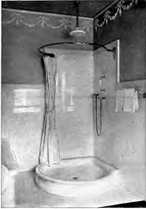
A shower bath with porcelain basin and marble back in continuation of the wainscoting
