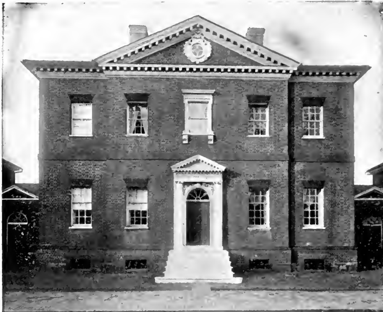
Central motive of the Hammond House, Annapolis, Md. Hip roof with pediment projection. The projecting courses between stories emphasise the floor line
