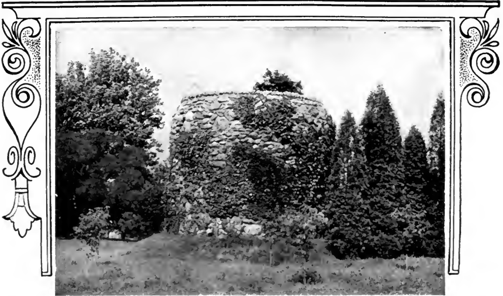
Nearly concealed by cedars and ampelopsis. This storage tank is enclosed in a shell of rough field stone. How different from many of the ugly tanks that disfigure the country
