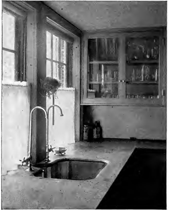
Tin-lined copper sink in butler's pantry, well lighted and convenient to cupboard
