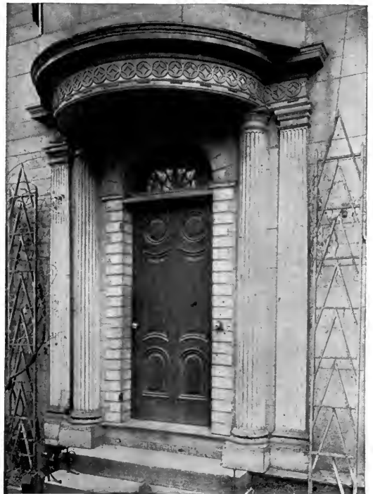
Old doorway in Washington Street, Boston, Mass. This example is somewhat marred by the more recent door and the ugly bay set foolishly on top of the hood.
