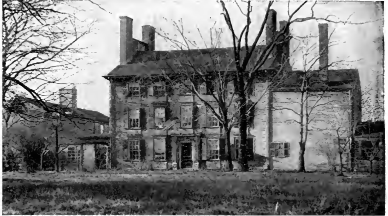
The old Royal House, Medford, Mass. Showing the simplicity of Colonial planning
