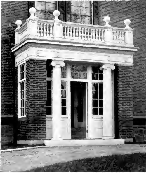
Entrance to a brick house at Cambridge, Mass. The trim is of wood, a common practice in Colonial work
