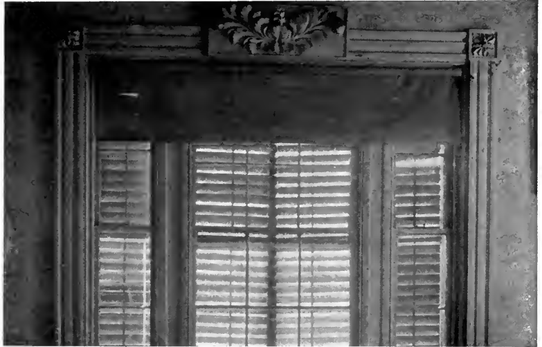
Interior of window shown on opposite page. A good example of the use of corner block and head panel
