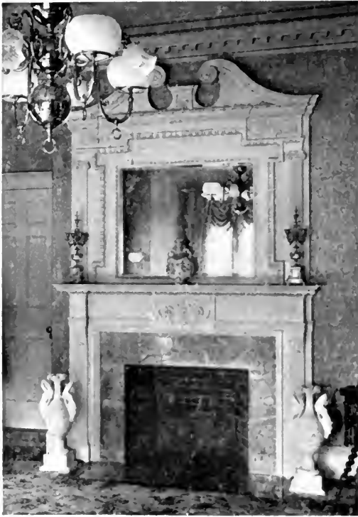
A parlor mantel at Lynn, Mass. The interrupted pediment makes a good top motive, but the mantel bears no relation to the lines of the room
