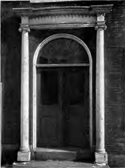
Doorway of old Custom-house, Portsmouth, N. H. This fine example has a touch of the Gothic in the entablature. It is perhaps a little light in composition with brick.
