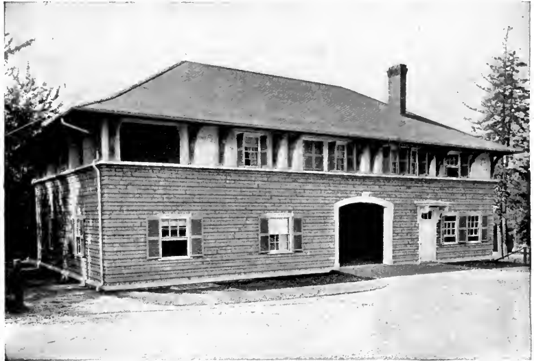
Stable on the D. C. Blair estate, at Bar Harbor, Me. Living quarters above. Could be built for about $12,000. Andrews, Jaques & Rantoul, architects
