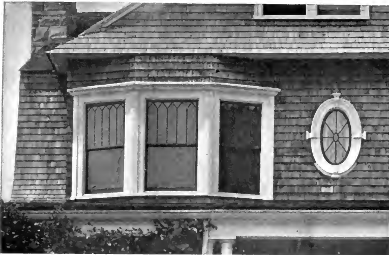
A second story bay at Newburgh, N. Y., with effective glass divisions. The oval Colonial window makes an excellent closet light
