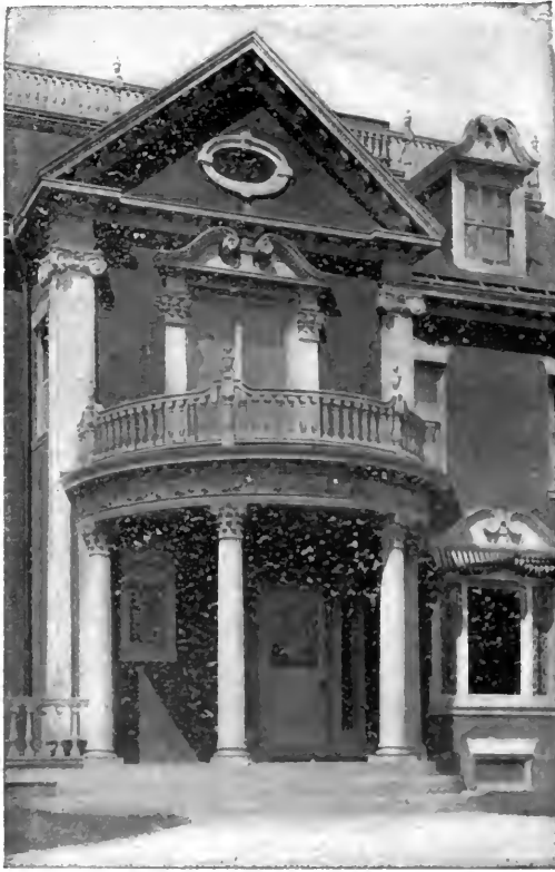
Entrance motive to house in Swampscott, Mass. Allen & Kenway, architects. The house is of brick and stone; the hood and columns of wood
