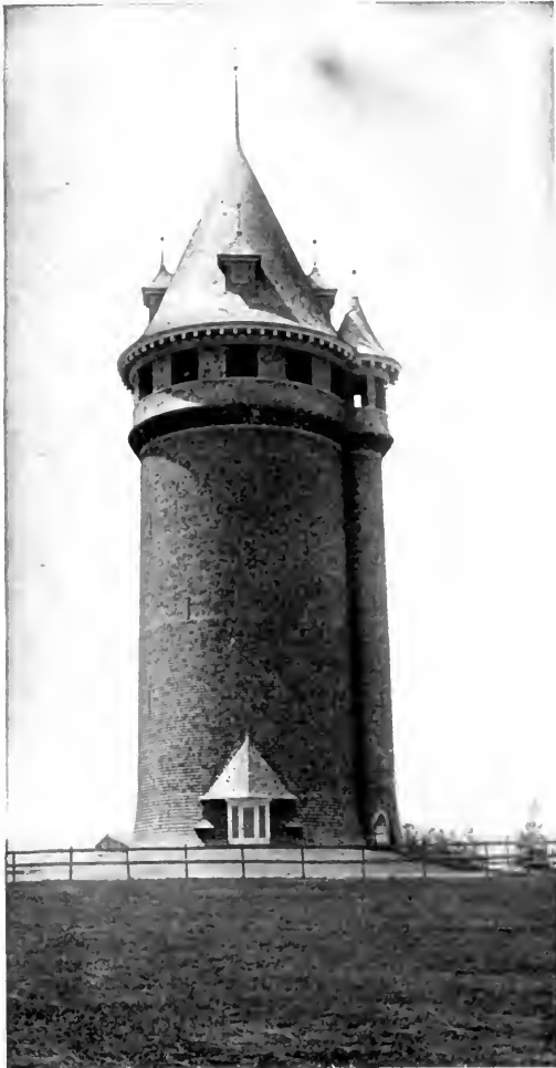
Hiding an iron standpipe by a wooden shell. A high tower near farm of Thomas W. Lawson, Esq., Egypt, Mass. A standpipe shell like this could be built for about $2,000. Coolidge & Carlton, architects
