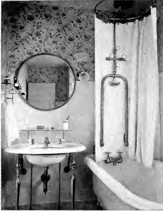
Portion of a small bathroom showing a handy shower bath and a serviceable lavatory and mirror
