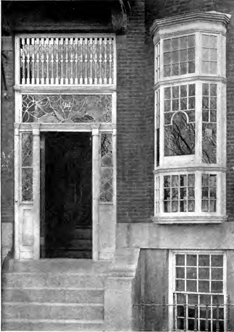
Excellent glass motives, both in the treatment of the doorway and the high bay. The latter might well be adapted to the staircase motive
