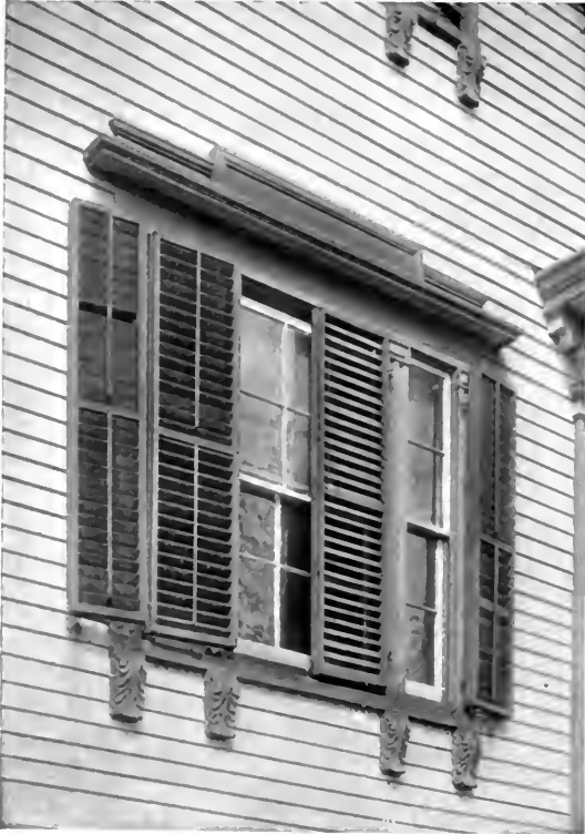
Mullioned window in old house at Flushing, Long Island, N. Y. The blinds should have been hung in two pairs so as to obtain the full light area
