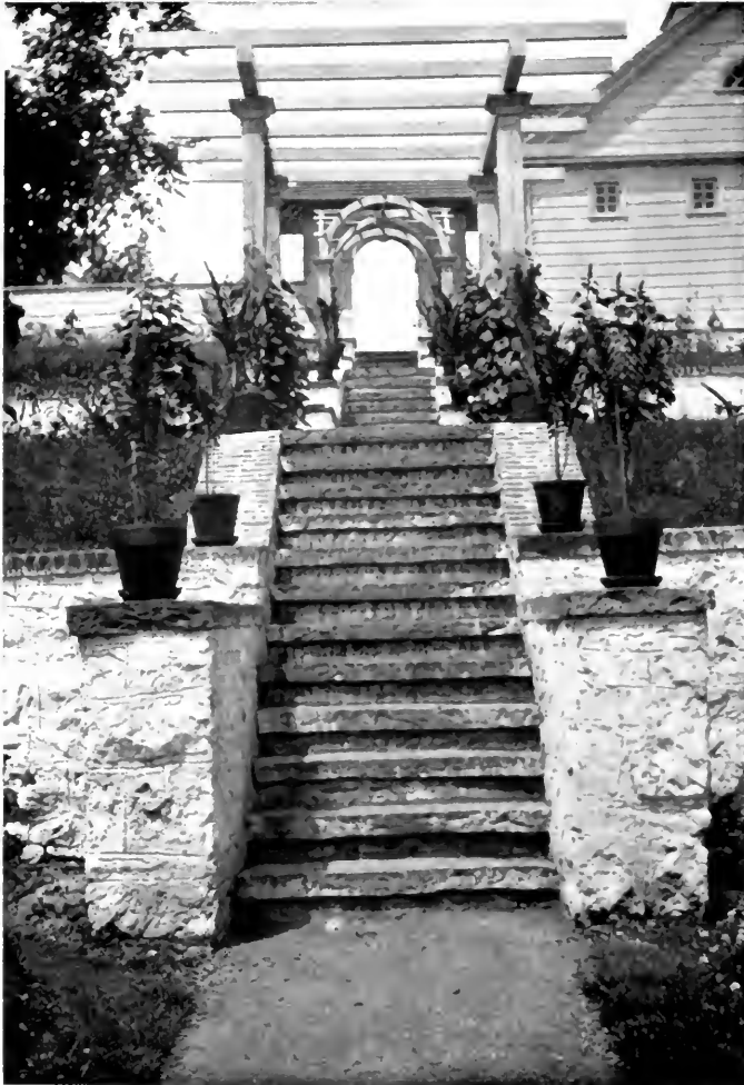
Garden steps. Estate of Mr. Frank Squires, Greenwich, Conn. Wilson Eyre, architect
