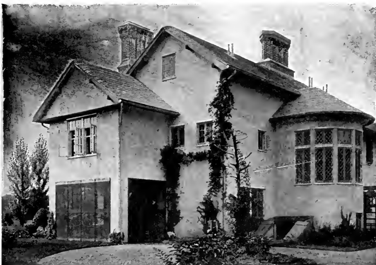
Another view of the Glen Ridge house, showing how the thatch effect has been suggested in shingles
