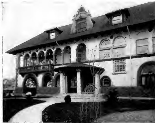
Portion of house near Philadelphia, Pa., showing good balcony and veranda motive. The cornice, while suggestive of the open type, is really a box cornice
