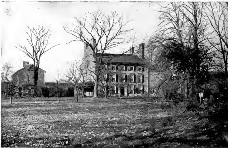
The old Royal House, Medford, Mass. Showing a flat Colonial site with deciduous growth. The lower view gives the anatomy of the general lay-out
