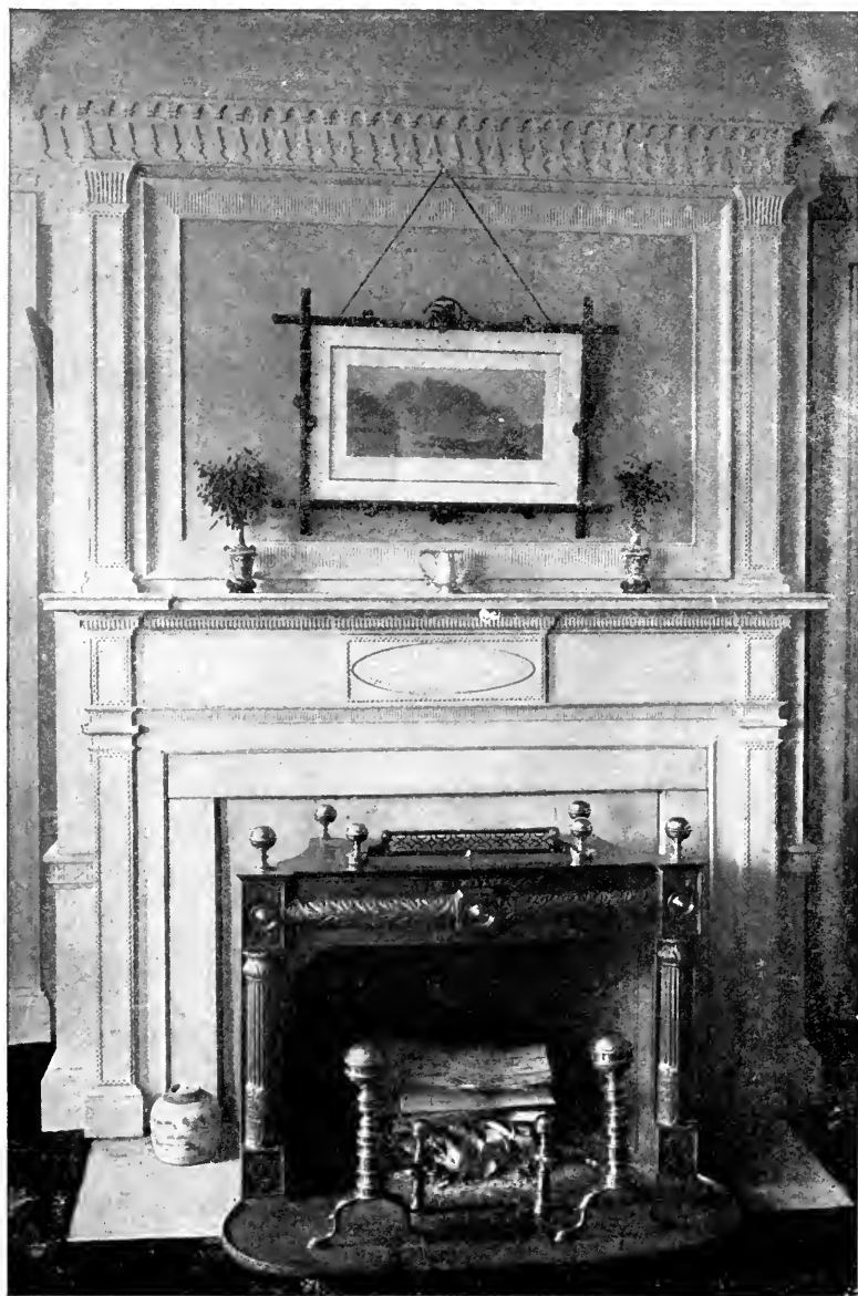
Old mantel in the Ladd House, at Portsmouth, N. H. The Franklin stove is here shown
