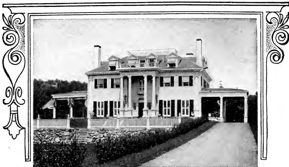
A modern Colonial house showing the hip roof "decked" at the top.
