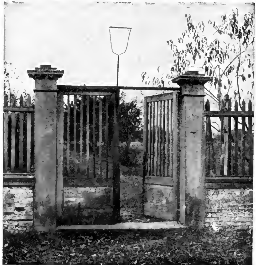
Garden gate of Royal House, Medford, Mass. A simple wood and brick treatment, having many practical advantages. Cost about $35
