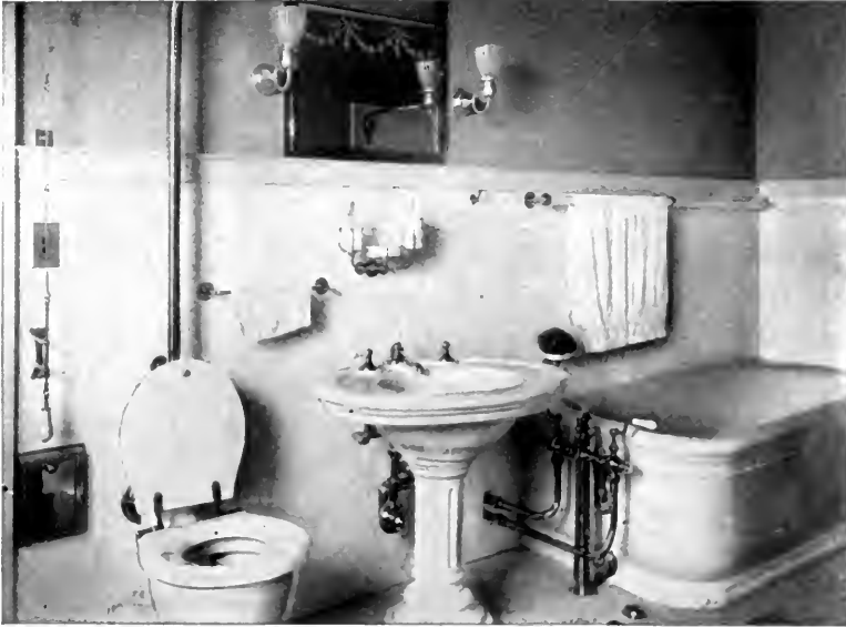
A good example of modern bathroom, with porcelain fixtures, marble wainscoting, tile floor and simple accessories
