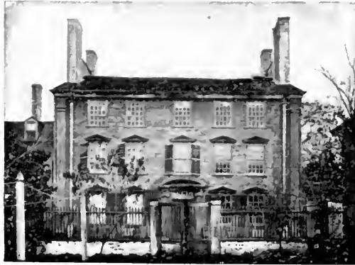
Court side of Royal House, at Medford, Mass., showing the combination of wooden side walls with brick ends in which the chimneys are placed
