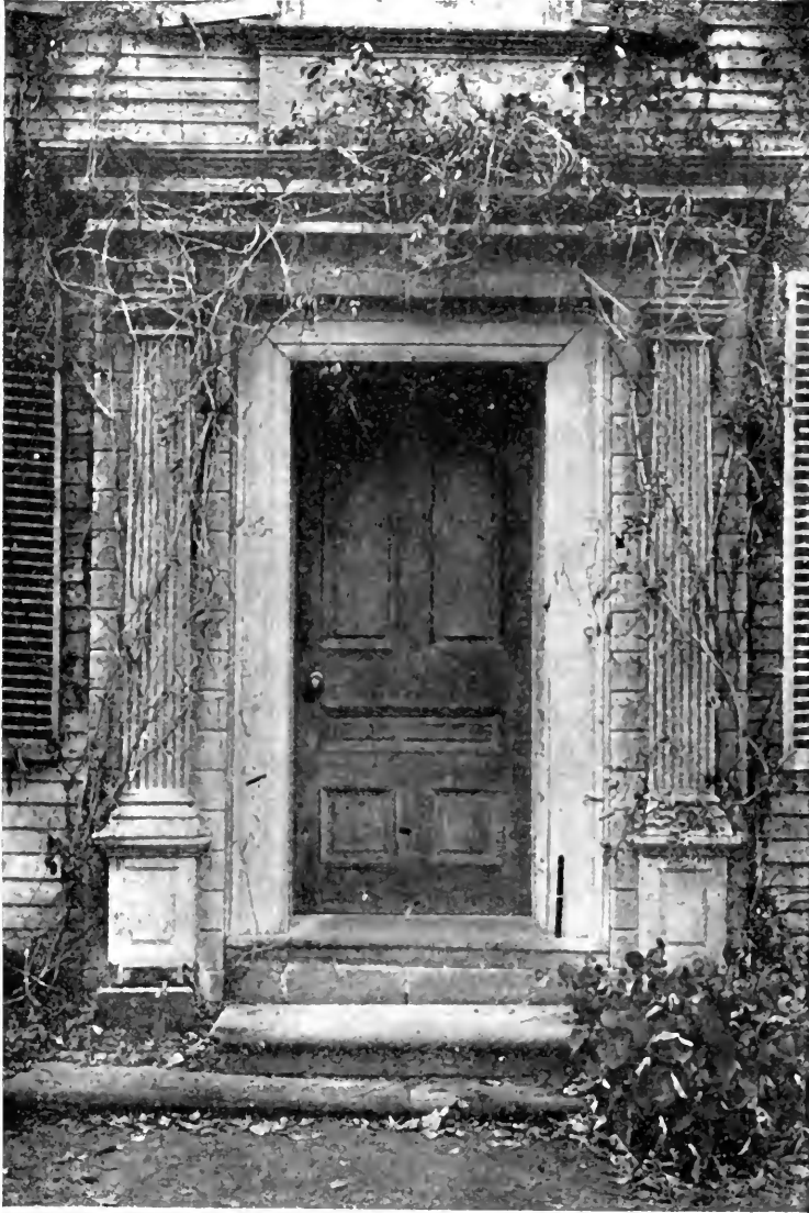
Street entrance to Royal House, Medford, Mass. This doorway is almost perfect. The proportions and mouldings are simple and good
