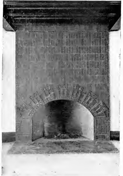
A glazed-tile mantel. For ordinary use the addition of a simple tile shelf, supported on consoles, would be desirable
