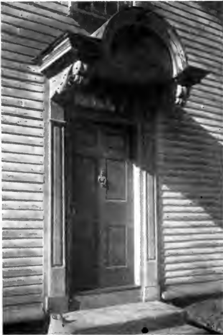
An unusual door hood at Newport, R. I.
