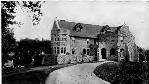
House at Merion, Pa. Gothic design in random, quarry-faced ashlar. Wm. L. Price, architect
