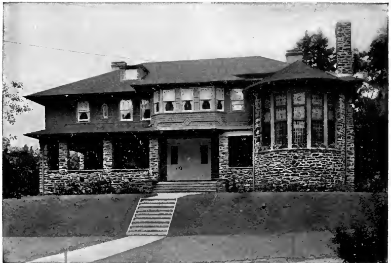
House at Lawrence Park, Bronxville, N. Y. A simple and vigorous example of stone and shingle work, with low-pitched hip roof. Wm. A. Bates, architect
