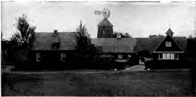
Windmill and tank combined to make a tower for the barn
