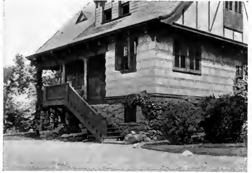
Servants' quarters of house, at Newburgh, N. Y., showing a good piazza and steps; also a telling use of the long shingle effect
