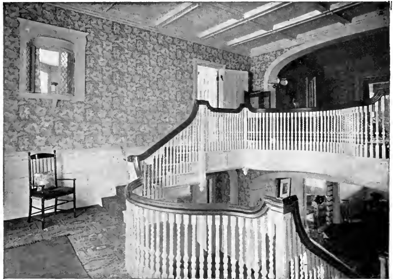
An upper stair-landing, showing the ramp and curve of the hand rail
