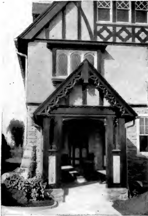
Entrance motive to house at Philadelphia, Pa. Walter F. Price, architect. A good combination of stone, plain rough-cast and half-timber work. The carving is delightfully crisp and simple
