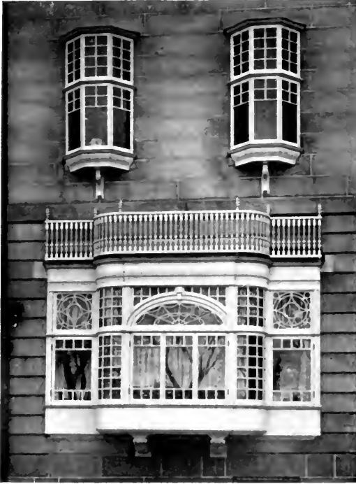
Modern Colonial bays on Beacon Street, Boston, Mass. The estimated cost of the bays, constructed of best pine stock, are: Large bay $285; small bays, each, $50
