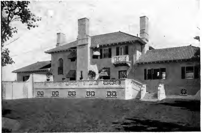
Entrance side of Cohasset house
