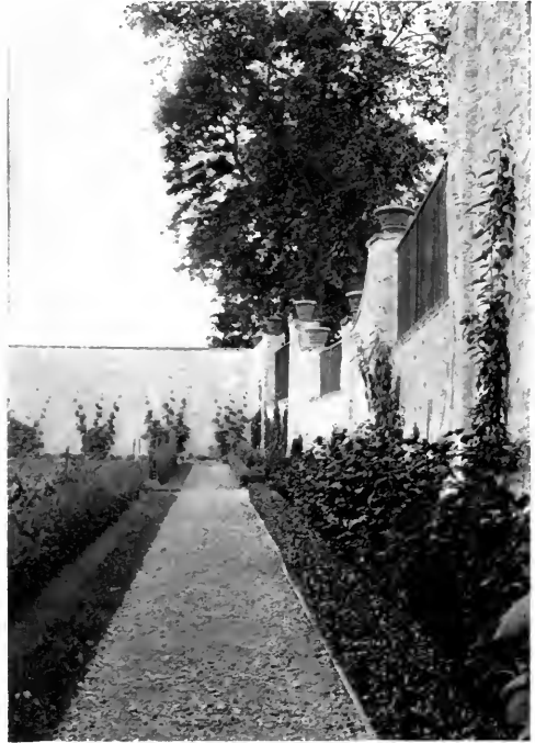
Garden wall at Greenwich, Conn. Estate of Mr. Frank Squires. Wilson Eyre, architect
