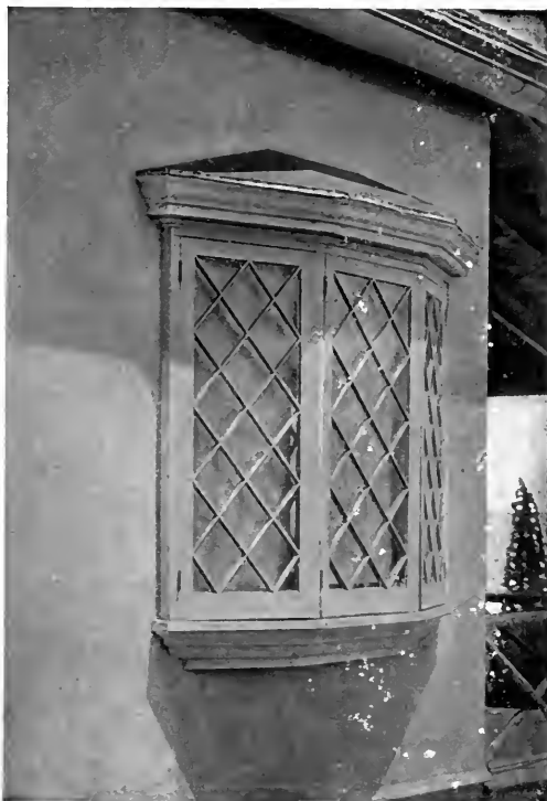
An example of the English casement window as applied to the bay. This very simple type has the English diamond panes, and is inexpensive, being in a stucco wall
