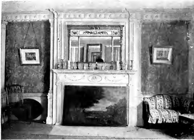
Mantel in the Nichols House, Salem, Mass. A successful rendering in which the flanking beams retain the squareness of the ceiling and serve to tie the motive to the rest of the room
