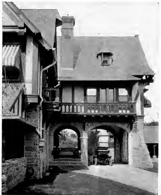
Portion of house at Bryn Mawr, Pa. Wm. L. Price, architect. A creditable handling of stone and stucco as influenced by French and English half-timber examples
