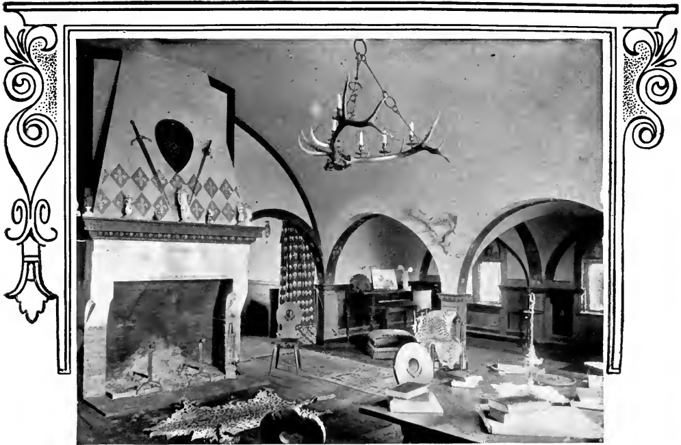
Den in the upper story of a house at Overbrook, Pa. Very suggestive of the medieval hall. Wm. L. Price, architect
