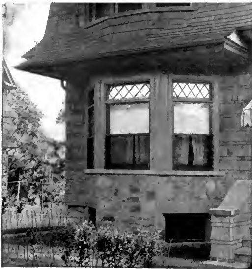
A bay at Newburgh, N. Y., used in connection with the gambrel roof. The stone underpinning extends to the window sills and gives a generous stool on the inside
