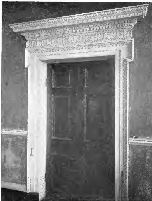
Interior doorway at "Whitehall," Maryland. A beautifully rich example of Colonial work
