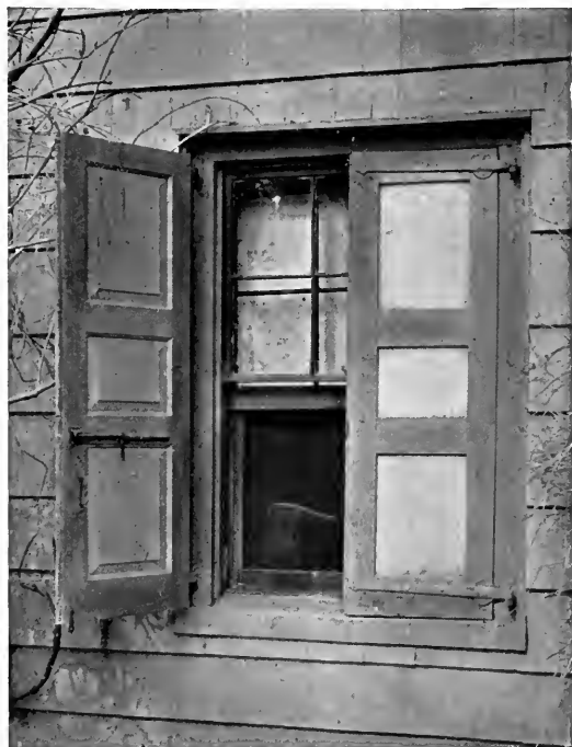
Window in old Bowne House, Flushing, Long Island, N. Y. The solid shutter, common during the Colonial period, was frequently pierced through the upper panel by a crescent or star form for the admission of a faint light
