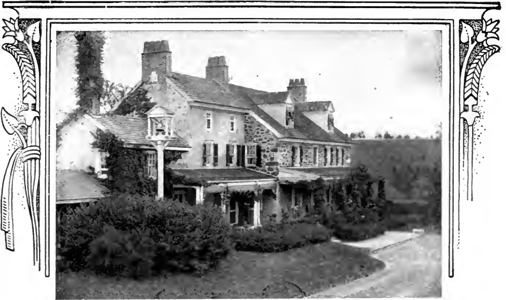
A $12,000 house of field stone partially covered with stucco; a type common in English towns
