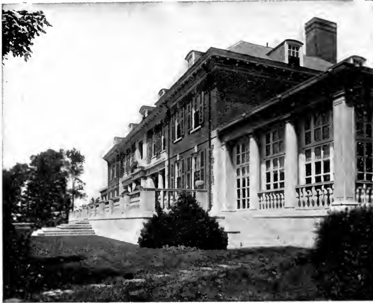
"Maxwell Court," Rockville, Conn. An excellent example of clean and healthy design. The low hip roof is decked to reduce the height, and thus add to the effectiveness of the long lines. Charles A. Platt, architect
