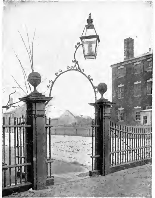
Old Colonial gates at Salem, Mass. A good example of wood design, in which the sweep of the carriage gates is continued in the smaller gate. The iron work, however, sits rather awkwardly upon the posts. Cost about $75.
