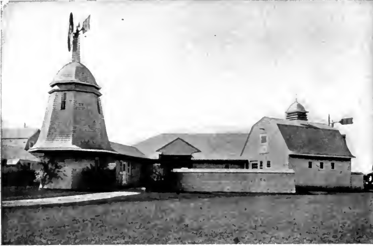
A tank at West Hampton Beach, Long Island, that harmonises with the other buildings. Many tanks are ugly and out of place. This one "belongs." It supplies both house and farm with water. Frank E. Wallis, architect
