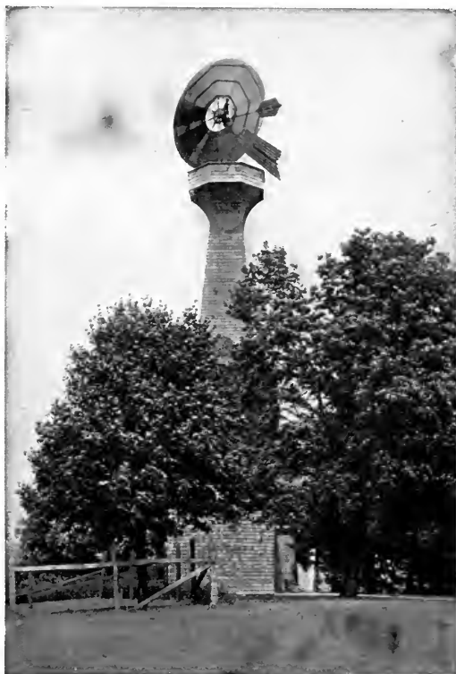
A windmill that is not unsightly. Everyone who can afford to cover the steel frame of a tank with a wooden shell should do so out of respect for neighbours, visitors, and the landscape
