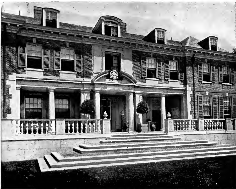
"Maxwell Court," Rockville, Conn. Charles A. Platt, architect. This is a most interesting example of brick and stone work designed on Italian lines. The wooden cornice is of the box type and is well proportioned
