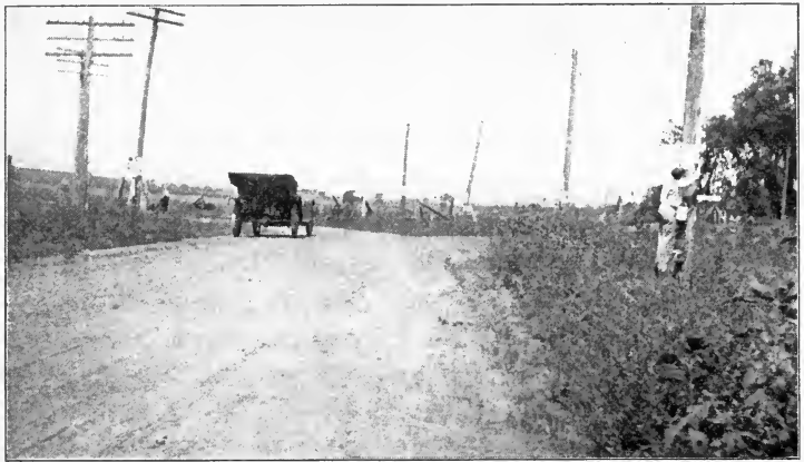
Marking the Route of the Iowa River-to-River Dragg'd Road
