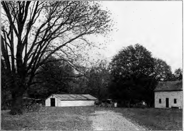
Barn and Janitor's House, John Swaney School
