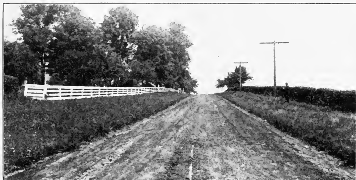
A Properly Dragged Earth Road
