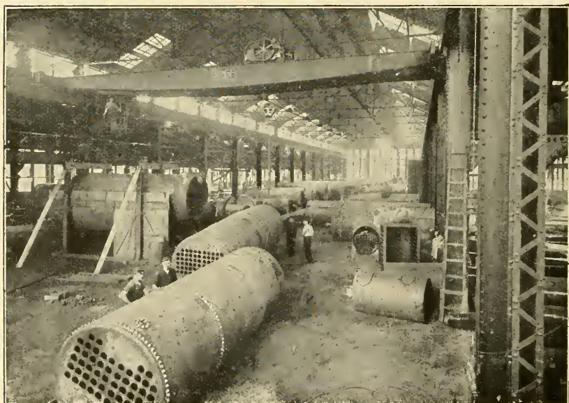
Boiler Shop - Looking North in Central Bay.
