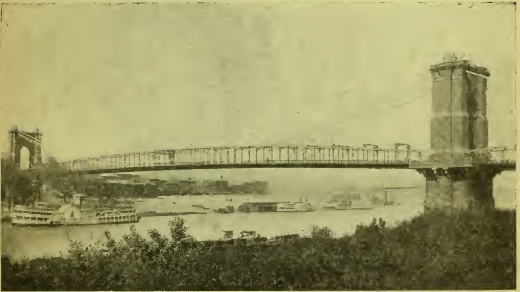
Suspension Bridge connecting Covington, Ky. and Cincinnati, Ohio
