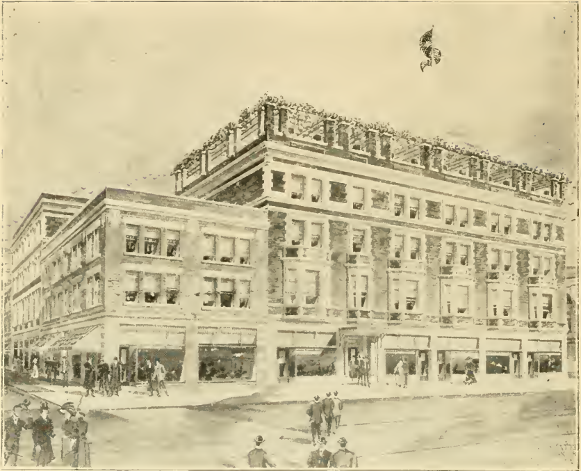
NEW $150,000 Y. M. C. A. BUILDING (in course of erection)
